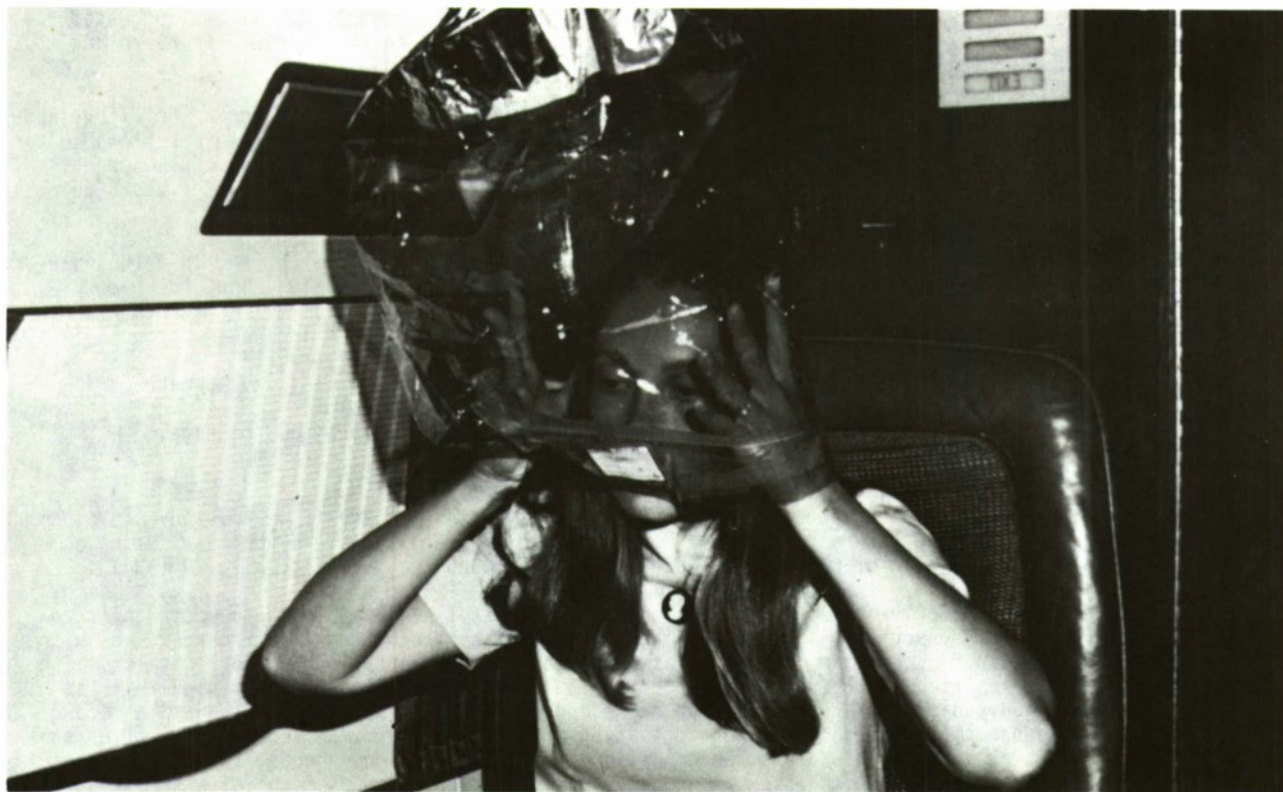
Fig. 24. Demonstration of passenger donning Schjeldahl "S" model "safety" hood in Chrysler Corporation Gulfstream. This smoke hood is presently in use in many corporate, FAA, and other aircraft and has been recommended in several studies for use in USAF air transport aircraft (Photo courtesy Chrysler Corporation).
