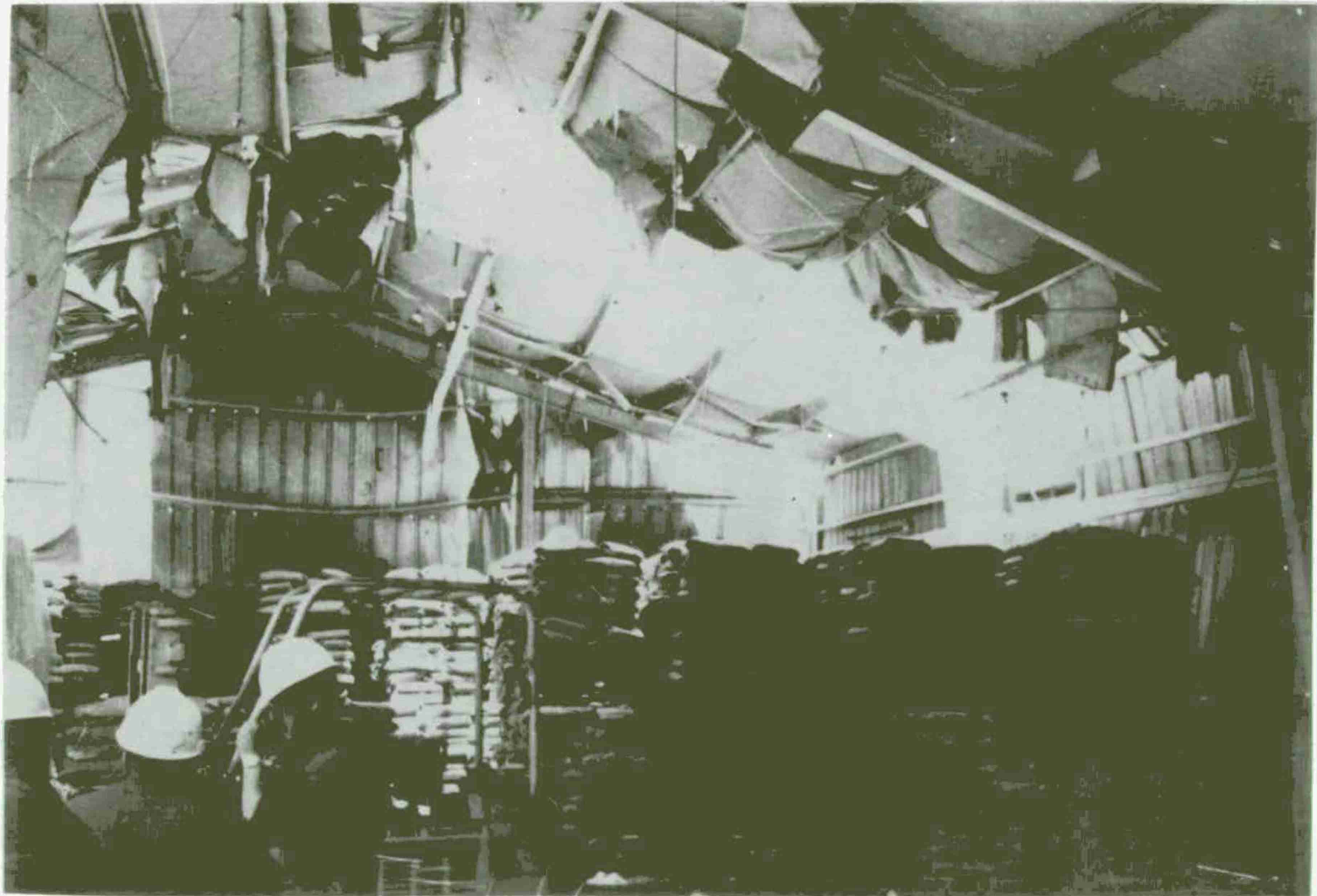
Fig 4B Rear wall of building No. 1 (interior view) ( P_{so} \approx 2.5 psi)
