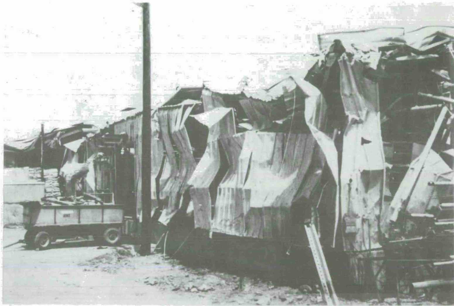
Fig 5B Side wall of building No. 1 (exterior view) ( P_{so} \approx 3.5 psi)
