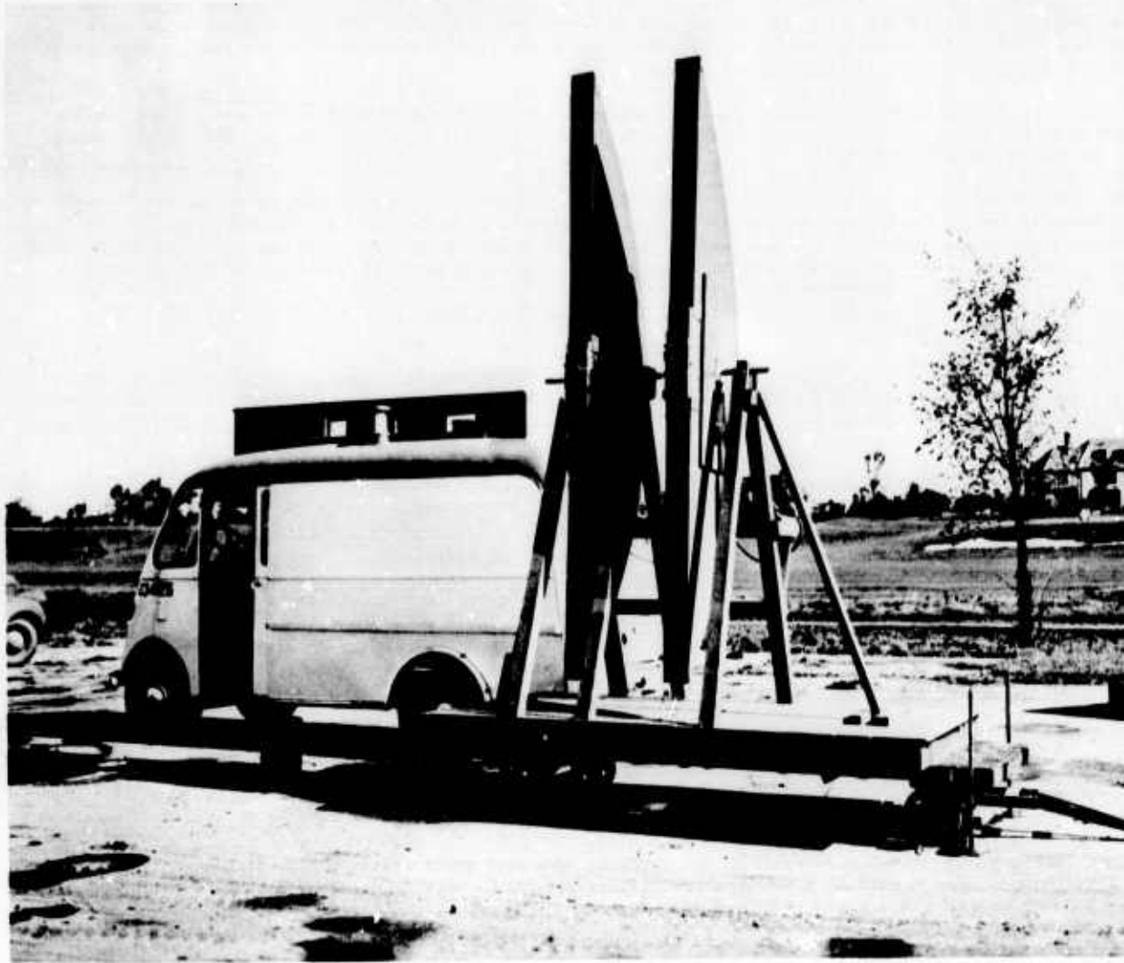
Figure 2.1 Early 3000-MHz Sperry Microwave Glide-Slope System (about 1942)
