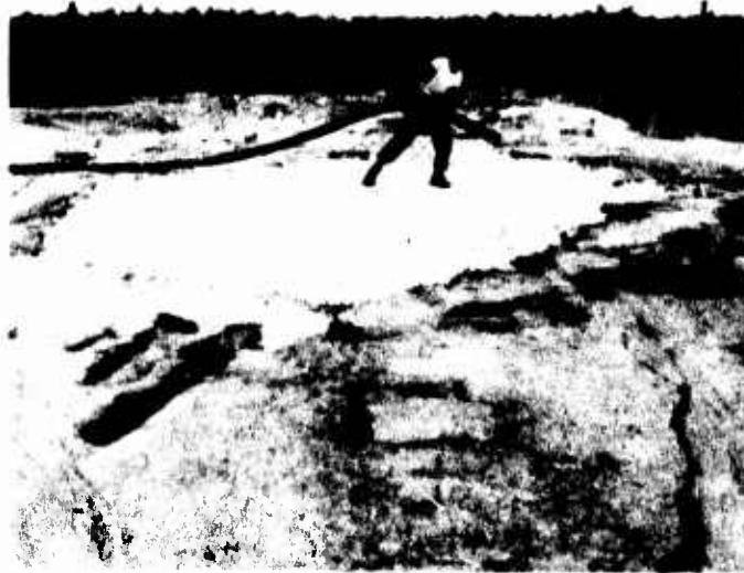
Figure 5.53 Select fill aggregate placed to existing pavement surface.
