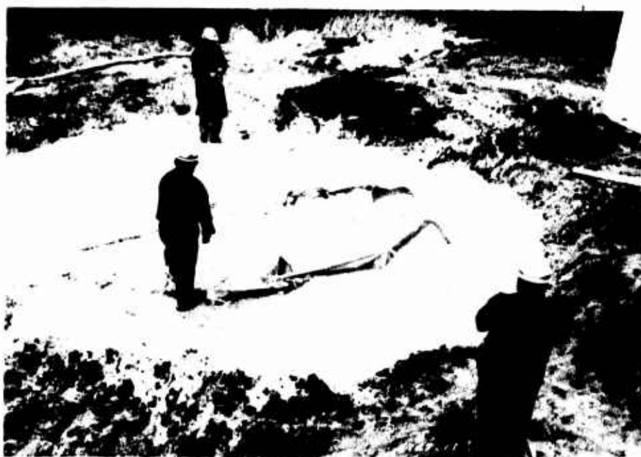
Figure 5.20 Completion of cellular concrete placing.
