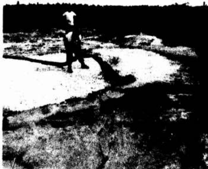
Figure 5.54 Placement of slurry on fill surface.
