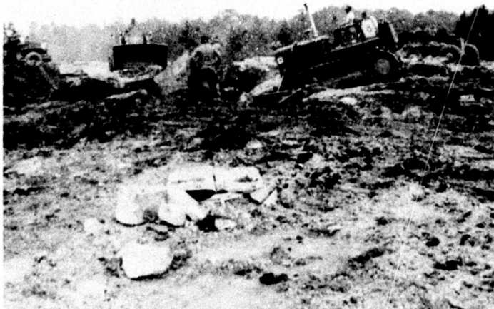
Figure 1.12 Pushing debris into crater.
