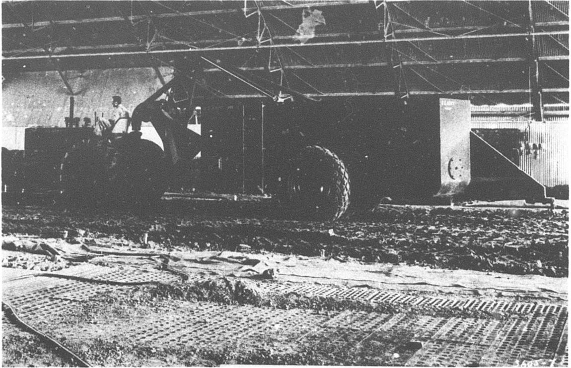
Fig. 1. Roller used in compaction of items 1 and 2
