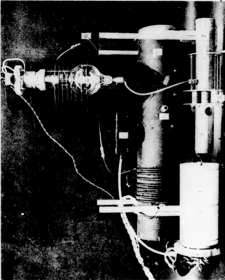
Figure 6. Coaxial Pulse Generator
