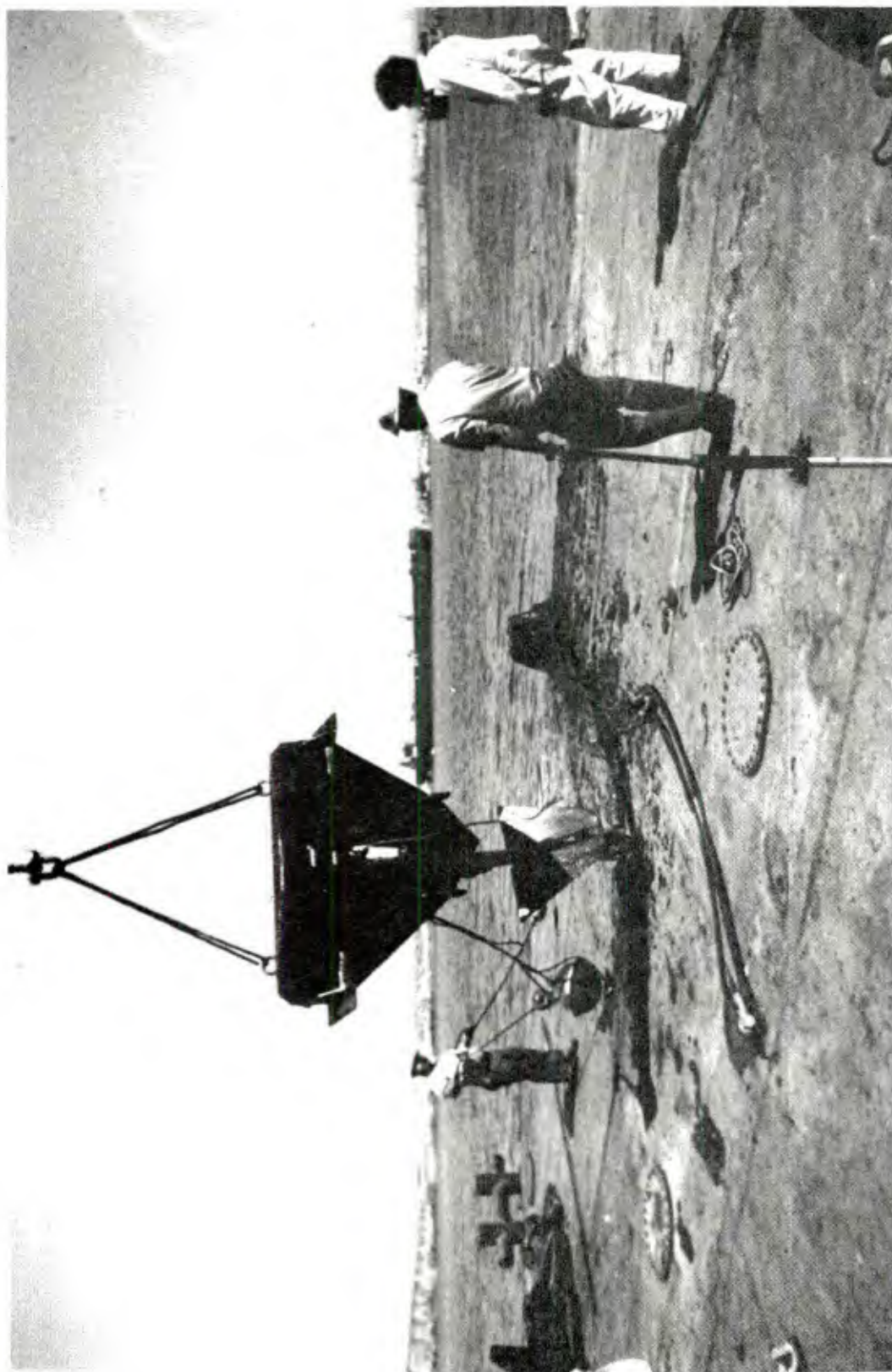
Figure 21. Hook anchor with auxiliary flukes.
