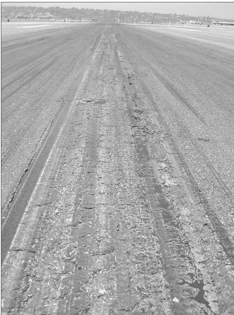
Figure 8: Cracked and Broken Runway Surface at Naval Base Coronado, California
