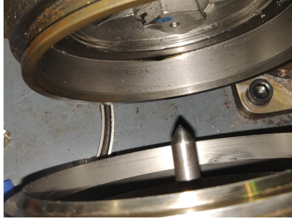
Figure 60. Turbine Axial Motion Limiter.
