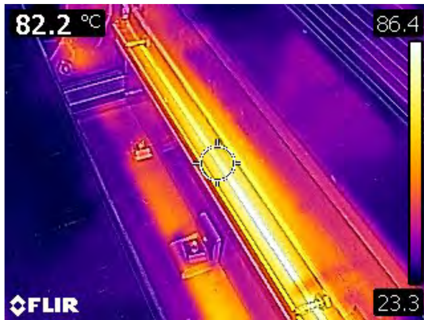
Figure 17. Capacity sensor load box 25 ohm resistor energized.
