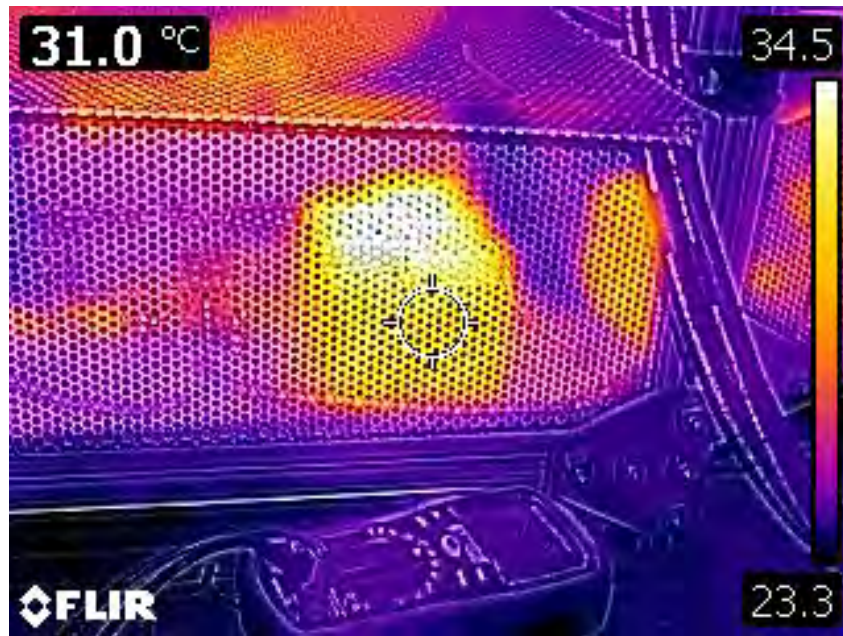
Figure 12. Capacity sensor controller under operation.
