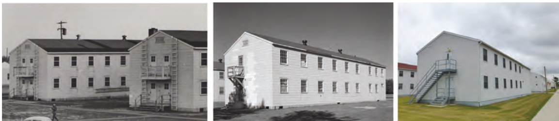
Front elevation of a 74-man barracks with comparison of the original construction, design, and materials from 1950 (left) to 1988 (middle) to 2018 (right). Note the original wood porch, steps, and handrails have already been removed and replaced with a concrete stoop and metal handrails in middle image (Left: NARA; middle: Library of Congress, HABS; right: ERDC-CERL).
