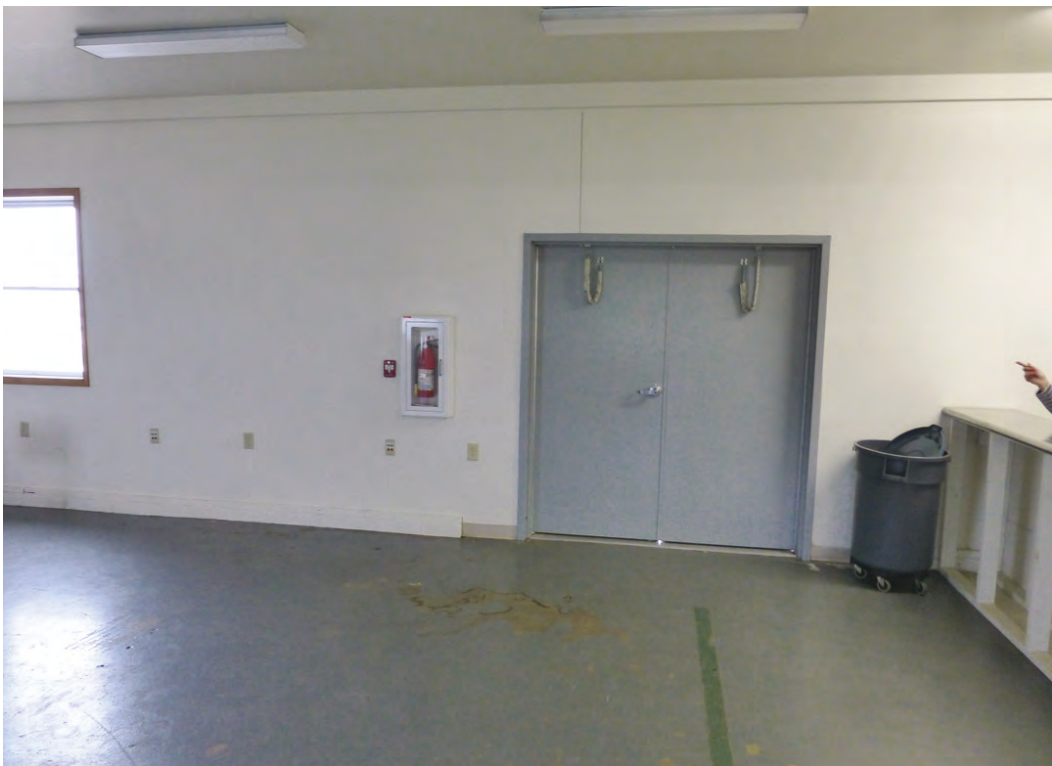
Photo 22. New metal doors replace the original wood sliding door on the east wall of the former storehouse/administration portion of Building 1621 (ERDC-CERL, 2018).
