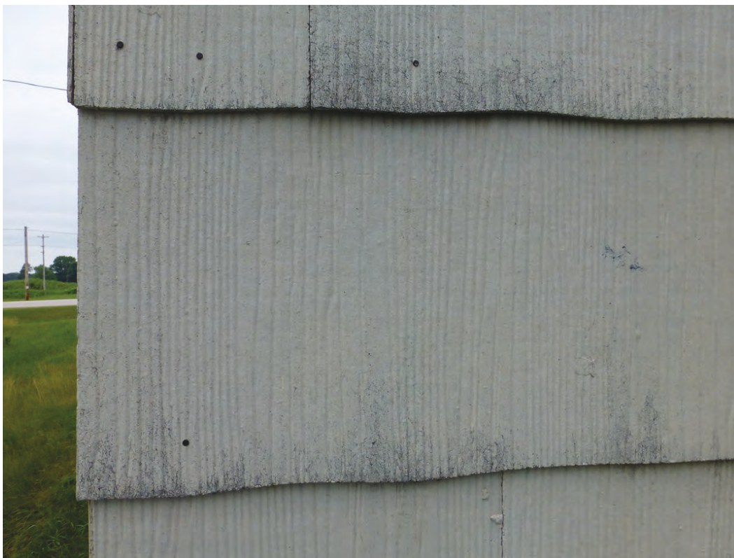
Photo 8. Close-up of the textured asbestos cement siding with scalloped bottom edge on Building 550 (ERDC-CERL, 2018).
