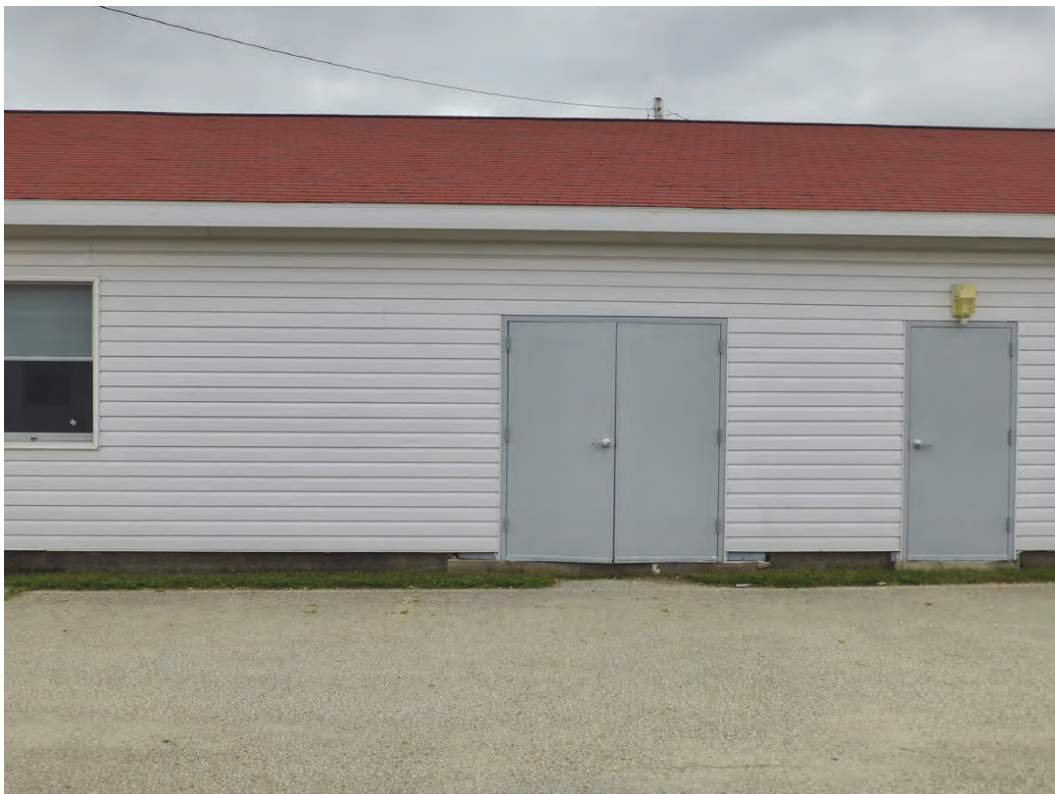
Photo 10. Replacement metal doors on the east elevation of Building 1621 (ERDC-CERL, 2018).
