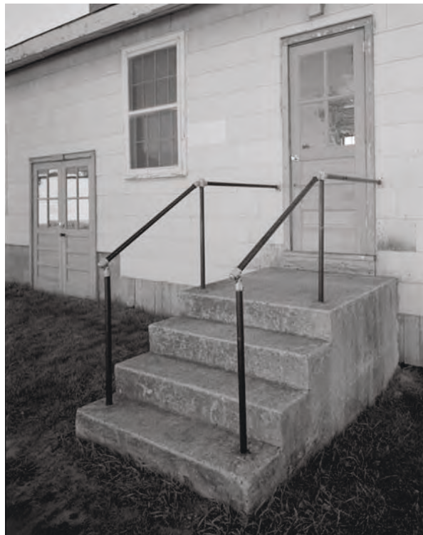
Close-up detail of concrete stoop, cast-iron metal handrails, wood panel and divided light doors, and multi-pane wood window and screen on Building 801, Company Storehouse/Administration and Recreation Building, September 1988 (Library of Congress HABS WIS, 41-SPAR.V, 1-B—5). The original WWII wood steps and handrails were replaced across Fort McCoy between 1965 and 1975.
