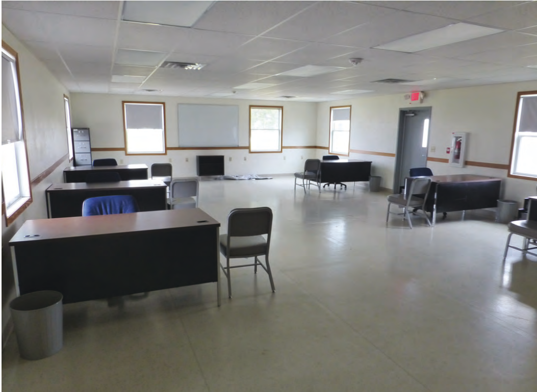
Photo 27. Looking north in the former recreation portion of Building 1621. Note the addition of drywall, drop-ceiling tiles, fluorescent light fixtures, wood trim around the windows, and vinyl tile flooring (ERDC-CERL, 2018).
