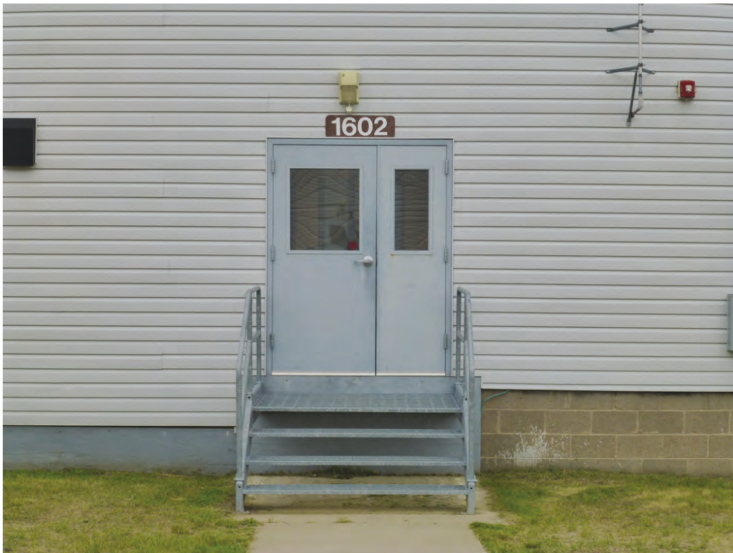
Photo 6. Replacement metal and glass doors, metal steps and metal handrails, vinyl siding, wood foundation skirting, and light fixture of Building 1602 (ERDC-CERL, 2018).
