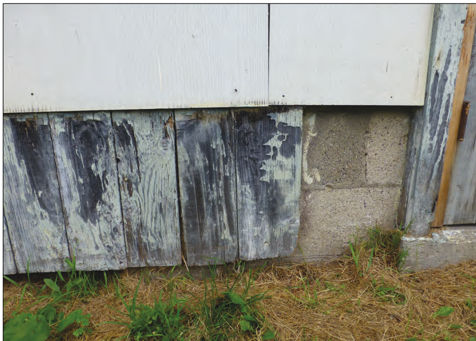
Figure 18. Wood foundation skirting on Building 849 (ERDC-CERL, 2018).
