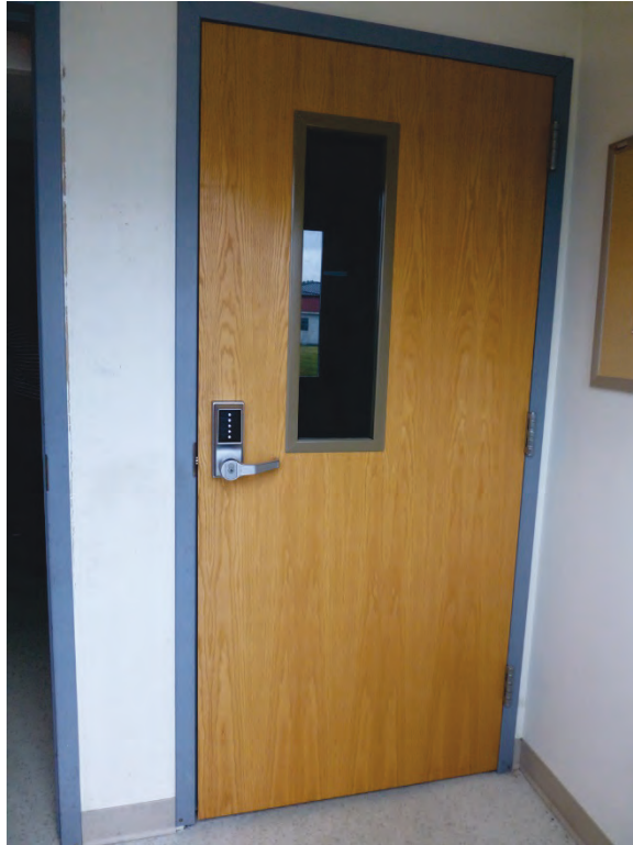
Photo 78. Replacement wood and glass interior doors used throughout the WWII barracks buildings (ERDC-CERL, 2018).
