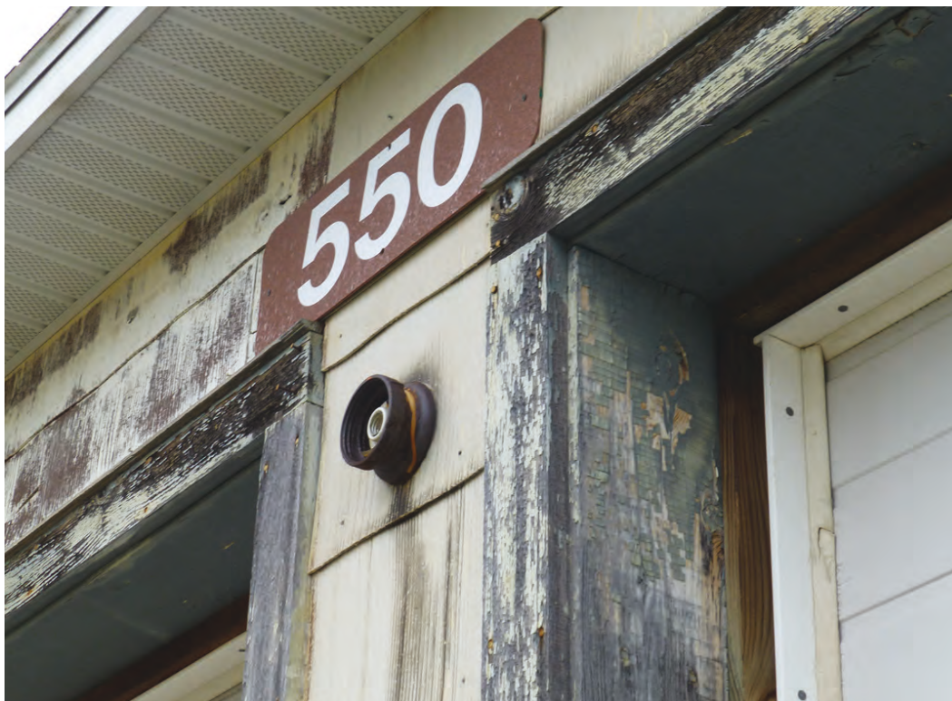
Photo 7. Close-up of the asbestos cement siding, wood trim around door openings, missing light fixture, and replacement metal soffit on Building 550 (ERDC-CERL, 2018).
