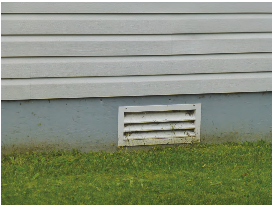
Photo 9. Close-up of replacement wooden foundation skirting on Building 1602 (ERDC-CERL, 2018).
