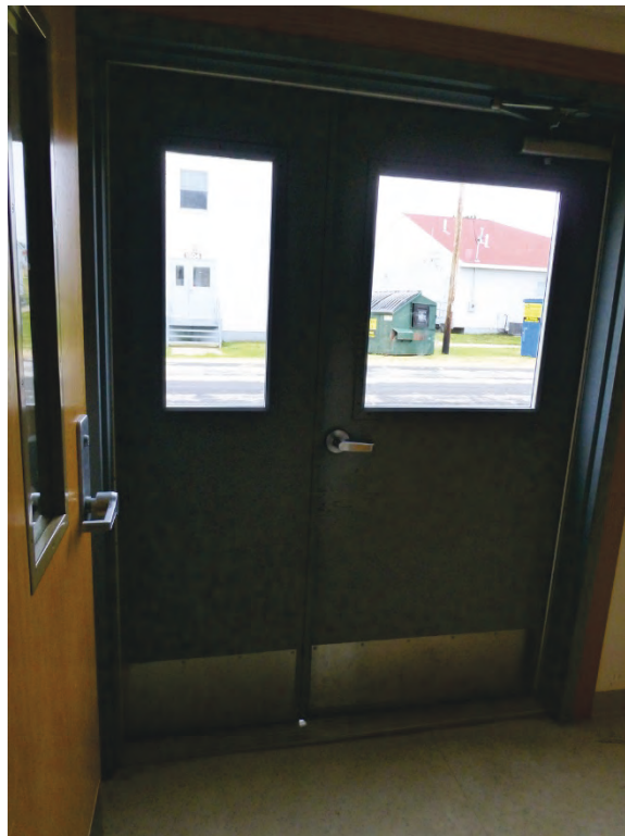
Photo 77. Interior view of the replacement metal and glass entry doors used throughout (ERDC-CERL, 2018).
