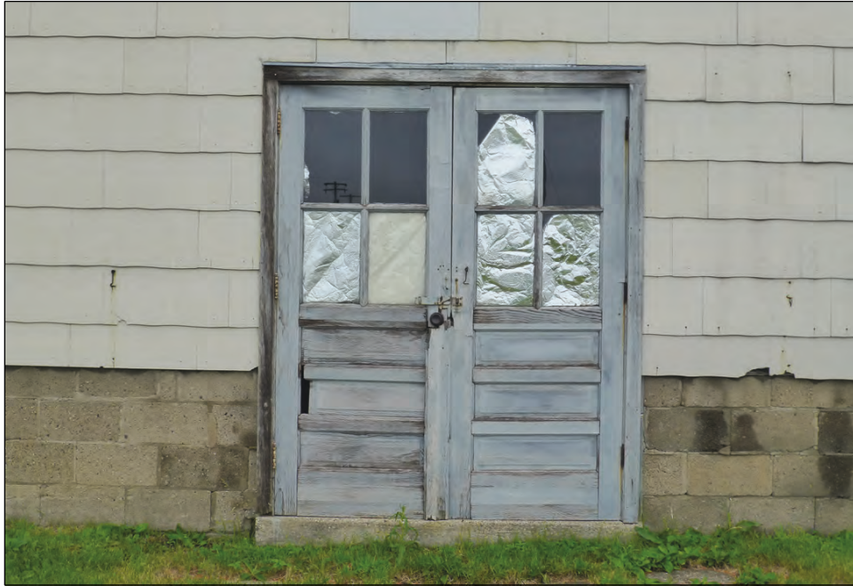
Figure 15. Multipaned doors with panels below on Building 849 (ERDC-CERL, 2018).
