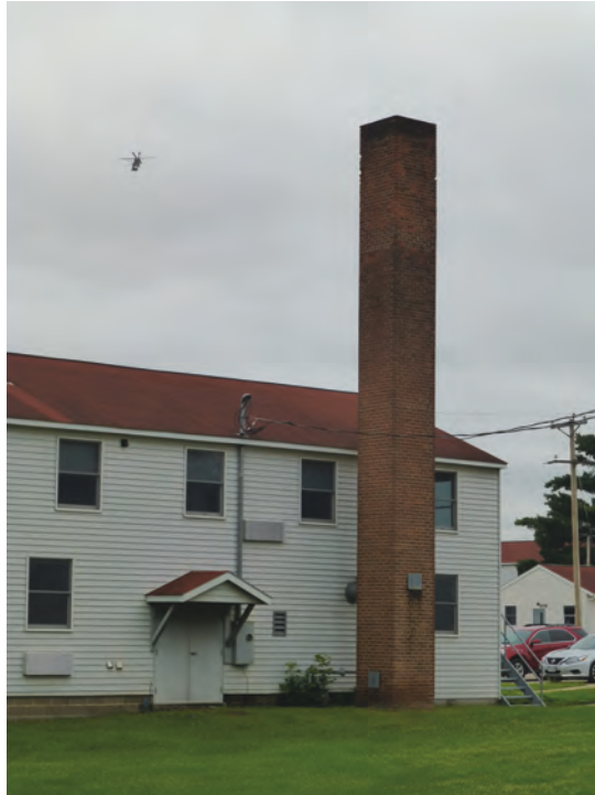
Figure 19. External brick chimney on Building 629 (ERDC-CERL, 2018).
