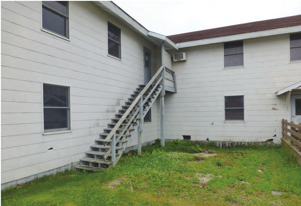
Photo 20. Connection between the east wing (left) and north wing (right) of Building 2000, with replacement windows, replacement fire escape door, and original wood fire escape stairs (ERDC-CERL, 2018).
