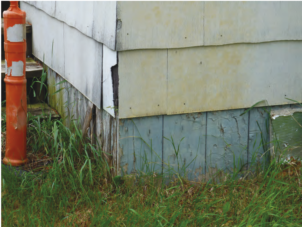
Photo 11. Close-up of the wooden foundation skirting of Building 550 (ERDC-CERL, 2018).
