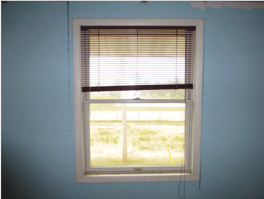
Photo 54. Replacement wood window trim in Building 2000 (ERDC-CERL, 2018).
