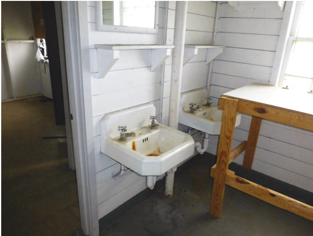
Photo 29. Original sinks, wood plank walls, mirrors, and shelves in Building 550 (ERDC-CERL, 2018).
