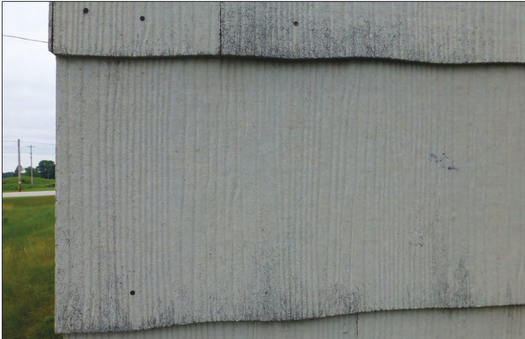
Figure 11. Cement asbestos siding with scalloped bottom on Building 550 (ERDC-CERL, 2018).
