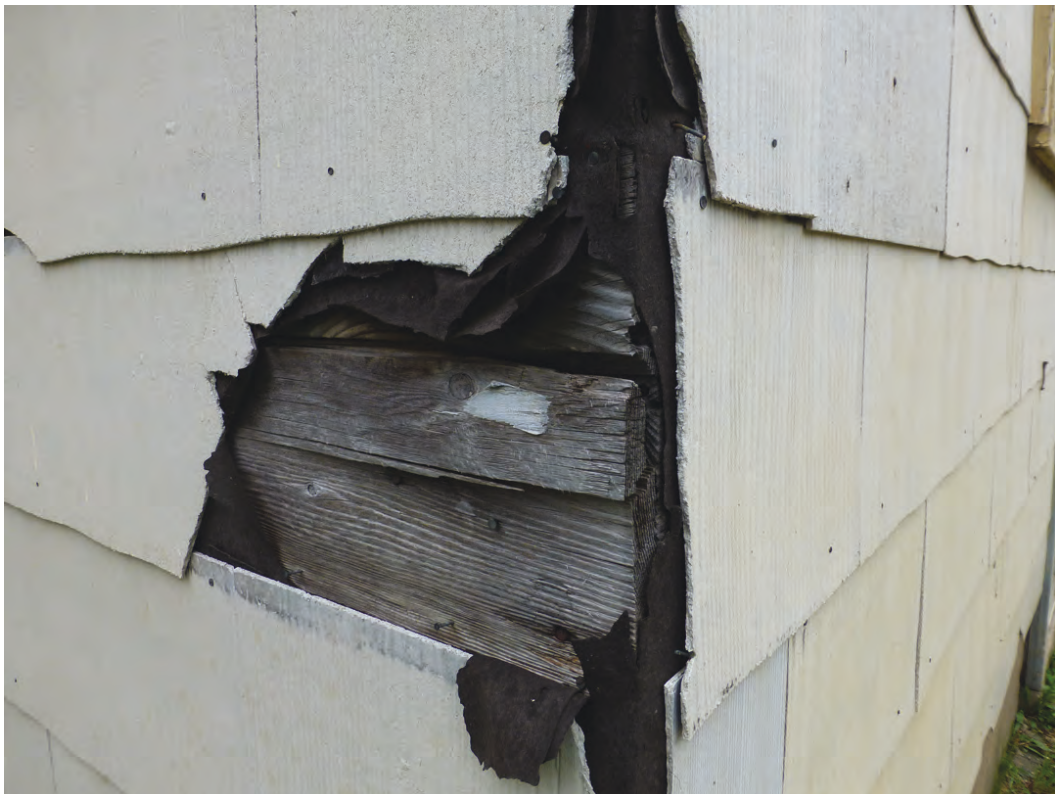
Photo 10. Close-up of damaged asbestos cement siding on Building 550 (ERDC-CERL, 2018).
