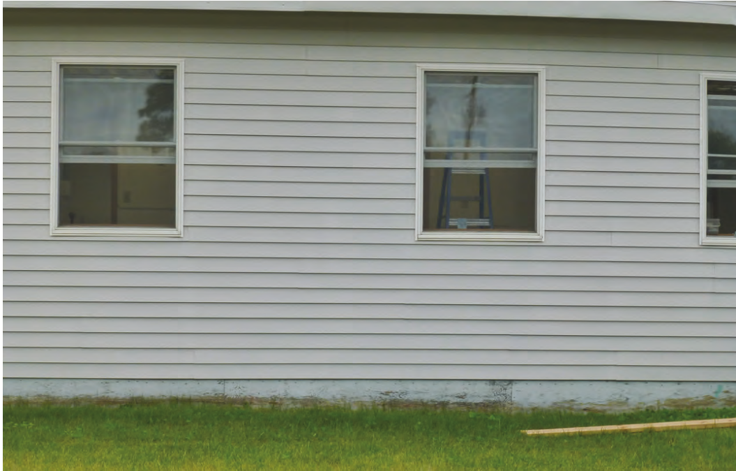
Photo 3. Close-up of the new vinyl siding, new wood foundation skirting, and replacement windows of Building 2668 (ERDC-CERL, 2018).
