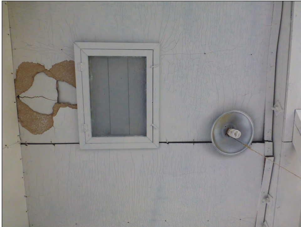
Figure 36. Fiberboard ceiling with in Building 550 (ERDC-CERL, 2018).
