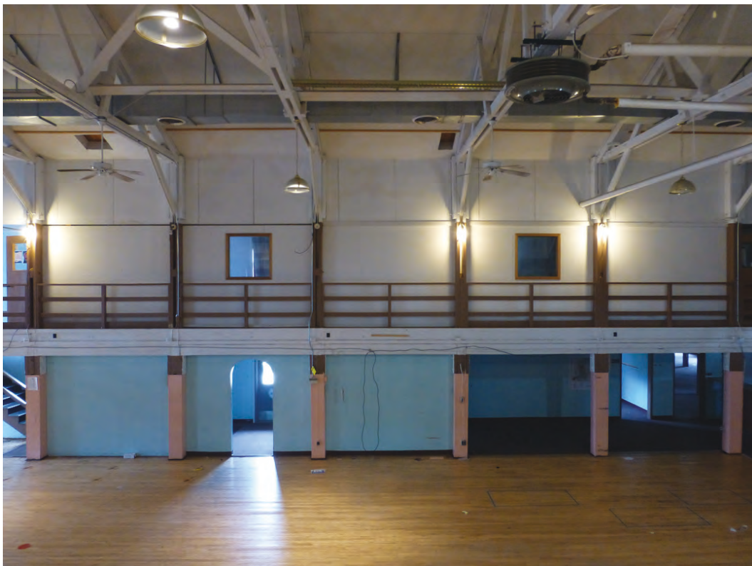
Photo 31. Looking at the east wall of the dance hall in Building 2000, with new partition walls enclosing the balcony level (ERDC-CERL, 2018).
