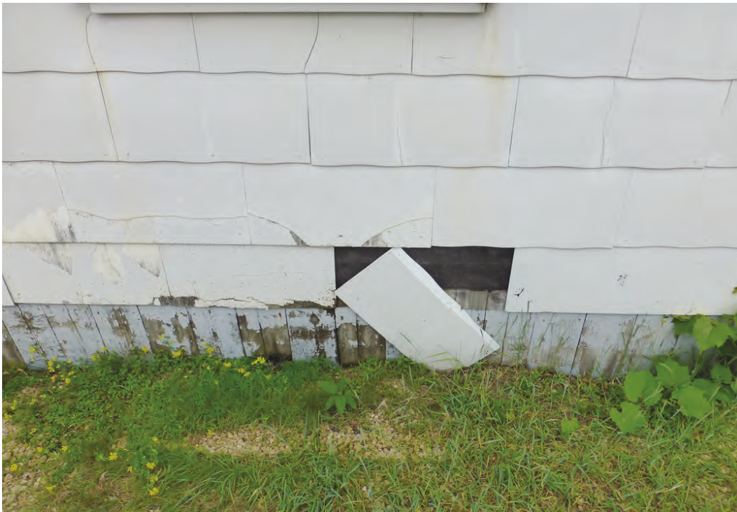
Photo 21. Close-up of original cement asbestos siding with scalloped bottom edge detail and original wood foundation skirting on Building 2000 (ERDC-CERL, 2018).
