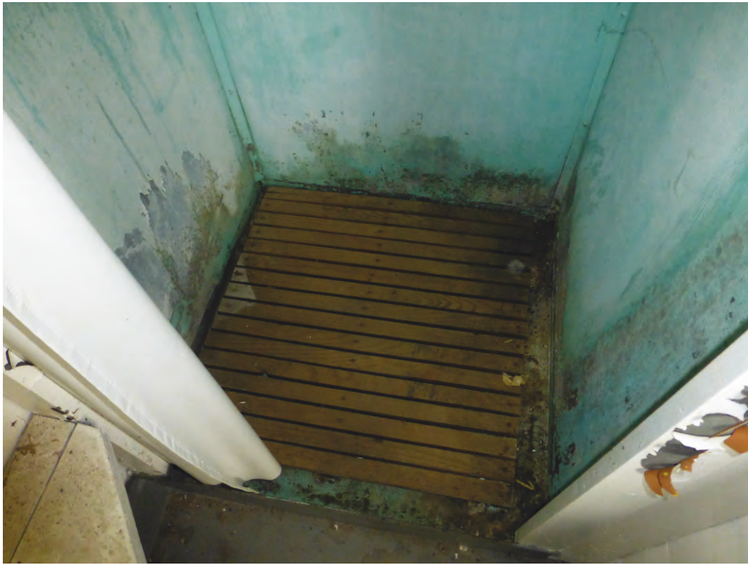
Photo 31. Shower stall in Building 550 with wood plank floor (ERDC-CERL, 2018).
