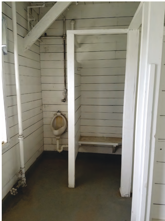
Photo 26. Original latrine area in Building 550 with original wood plank walls, exposed ceiling, concrete floor, and urinal (ERDC-CERL, 2018).
