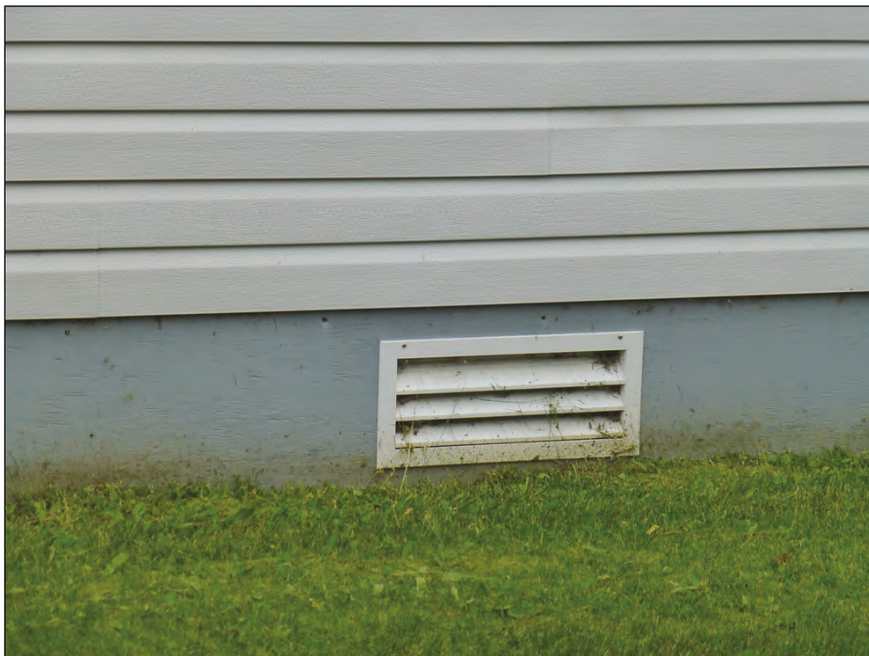
Figure 64. Replacement siding, foundation covering, and vent on Building 1602 (ERDC-CERL, 2018).
