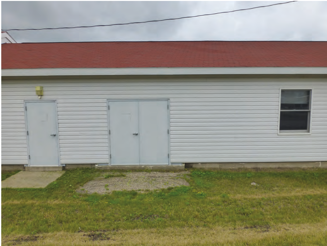
Photo 7. Replacement metal entry doors on the west elevation of Building 1601 (ERDC-CERL, 2018).
