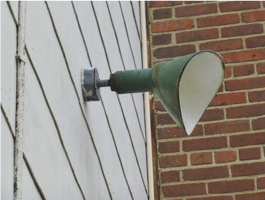
Photo 26. Original exterior light fixture located on the north elevation of the north wing of Building 2000, near the chimney (ERDC-CERL, 2018).
