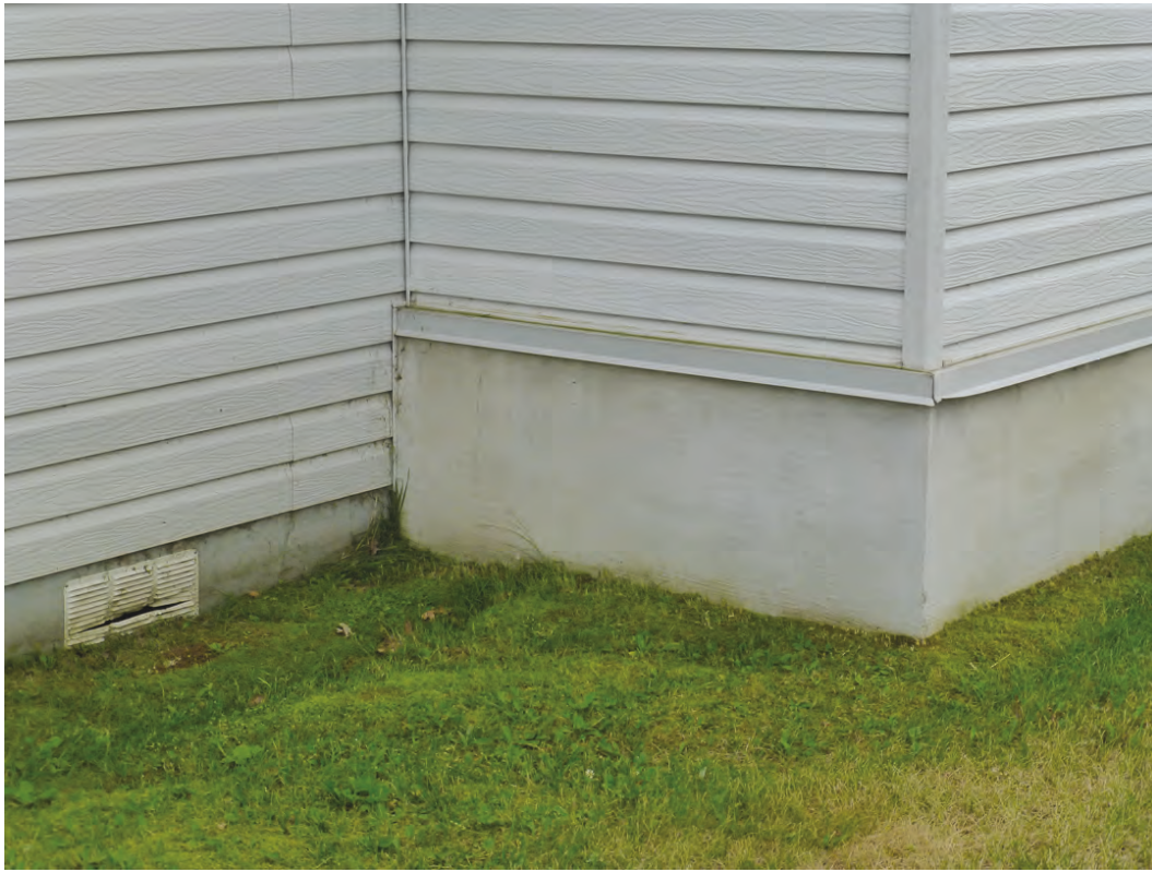
Photo 12. Close-up of foundation skirting on original part of the structure (left) compared to the poured concrete foundation of an appendage that was constructed at a later date (right) (ERDC-CERL, 2018).
