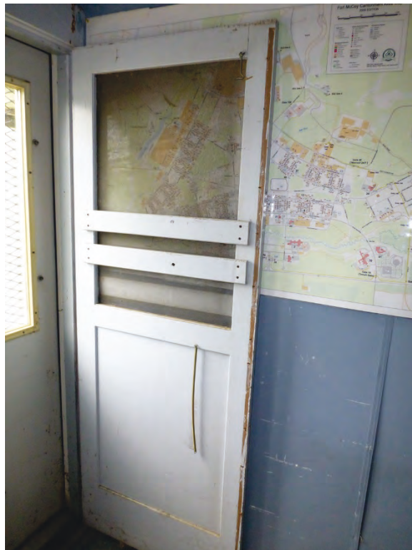
Photo 55. Original wood screen door on the south wall of the 1943 addition to Building 2000 (ERDC-CERL, 2018).
