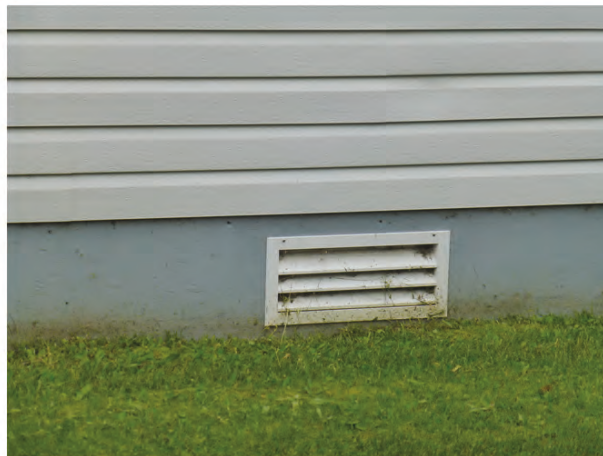
Original cement asbestos siding with scalloped edge detail and wood foundation skirting (left), compared to the replacement materials of vinyl siding and plywood foundation skirting (right) (left: Library of Congress, 1988 HABS; right: ERDC-CERL, 2018).
