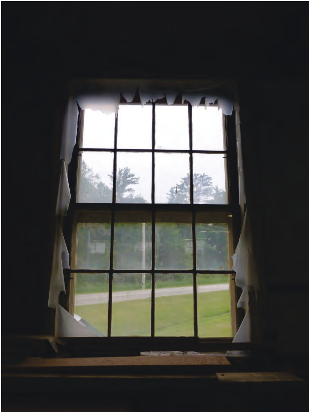
Photo 45. Interior view of an original multipane wood double-hung window in Building 550 (ERDC-CERL, 2018).
