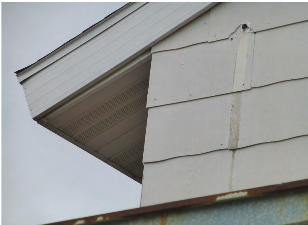
Photo 19. Close-up of modified roof overhang with replacement metal soffit and fascia on Building 2000 (ERDC-CERL, 2018).
