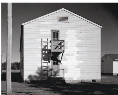
Rear elevation of a 74-man barracks with the original construction, design, and materials, as shown in 1988 photo (left) compared to 2018 (right). Note that the original first-floor wood porch, steps, and handrails have been removed and replaced by 1988 with a concrete stoop and metal handrails, plus the two original fire exit doors have been removed from the squad rooms, and those door openings have been covered with newer cement asbestos siding by 1988 (left: Library of Congress, HABS; right: ERDC-CERL).
