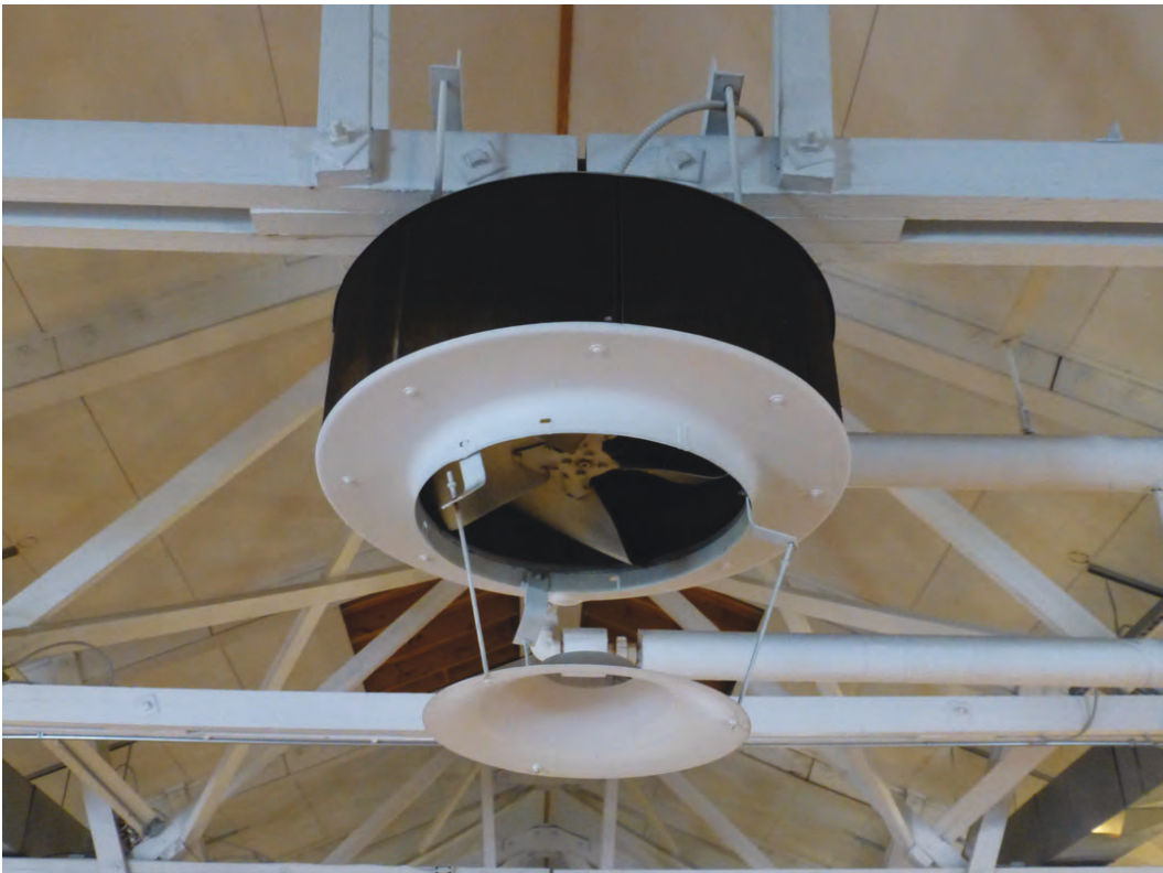
Photo 39. Close-up detail of the an original heater with diffuser that is supended from the truss system over the dance hall in Building 2000 (ERDC-CERL, 2018).
