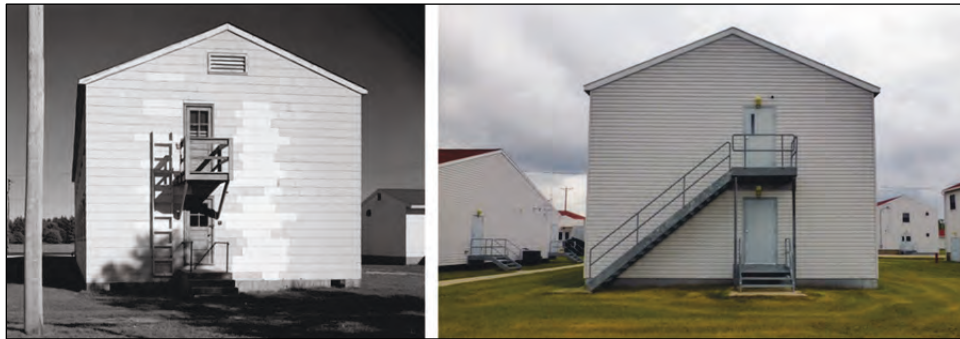
Figure 132. Window comparison of the original eight-over-eight wood double-hung window on a 74-man barracks (left) to the current replacement one-over-one vinyl window (right) (left: Library of Congress, HABS; right: ERDC-CERL).
