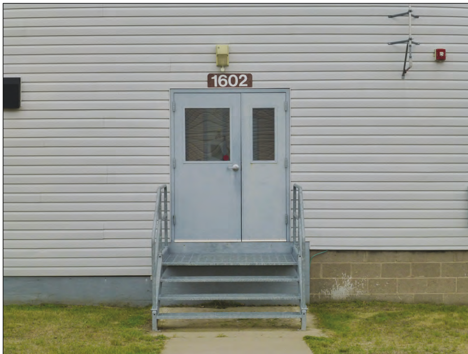
Figure 62. Main barracks entrance with metal door and metal steps on Building 1602 (ERDC-CERL, 2018).
