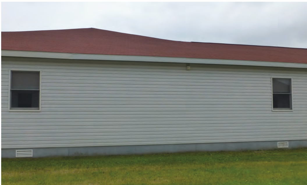
Photo 9. Close-up of replacement one-over-one vinyl windows, vinyl siding, and replacement wood foundation skirting (ERDC-CERL, 2018).
