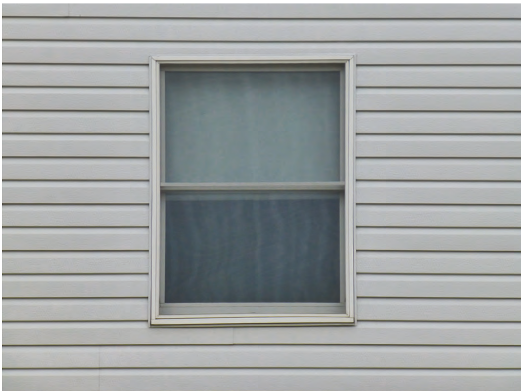
Photo 7. Close-up of replacement one-over-one vinyl window on Building 1602 (ERDC-CERL, 2018).
