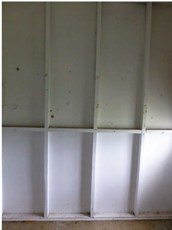
Photo 40. Interior view of the wood frame structural members in Building 550 (ERDC-CERL, 2018).
