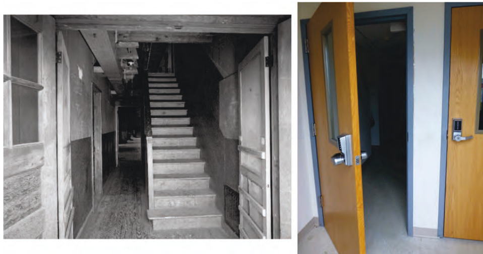
Figure 134. Interior view of the original open-bay entry vestibule with wood screen doors leading to the first floor and to the staircase (left) compared to the modified entry vestibule with partition wall and replacement interior wood door (right) (left: Library of Congress, HABS; right: ERDC-CERL).
