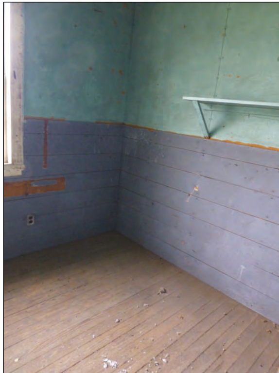
Figure 35. Fiberboard walls with wainscoting in Building 1866 (ERDC-CERL, 2018).
