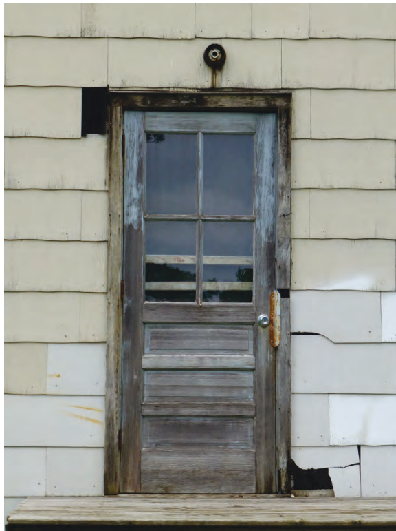
Photo 12. Original wood-panel and divided-light entry door on Building 550 (ERDC-CERL, 2018).
