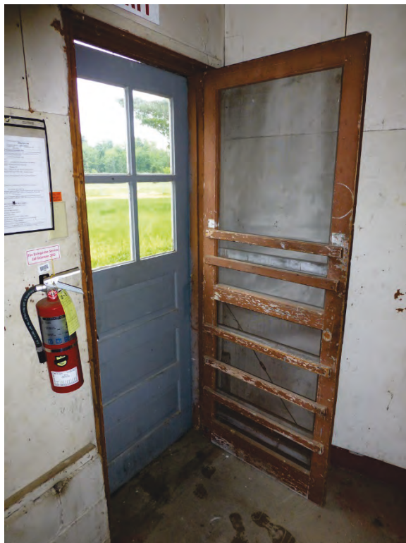
Photo 42. Original interior wood screen door in Building 550 (ERDC-CERL, 2018).
