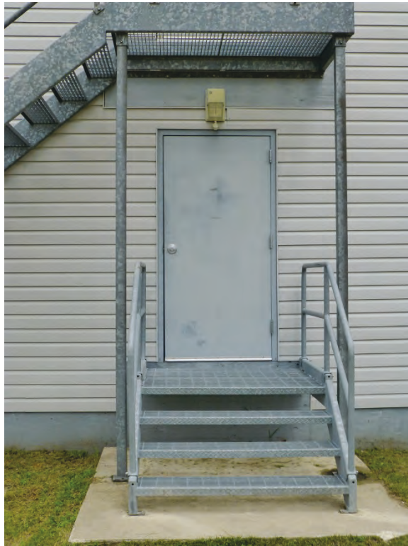
Photo 10. Replacement metal door, metal steps, and metal handrails on Building 1602 (ERDC-CERL, 2018).
