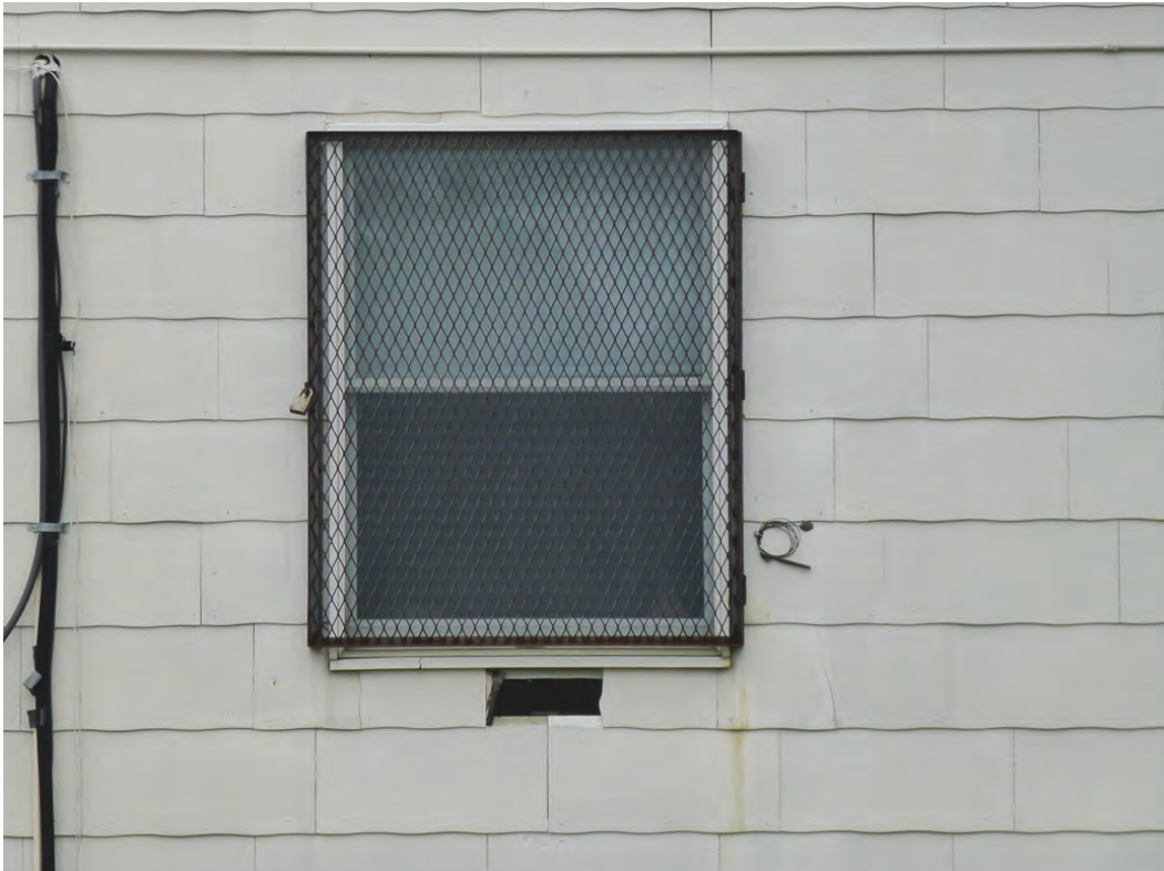
Photo 17. Close-up of replacement one-over-one vinyl window with new metal security screen and close-up of original cement asbestos siding of Building 2000 (ERDC-CERL, 2018).
