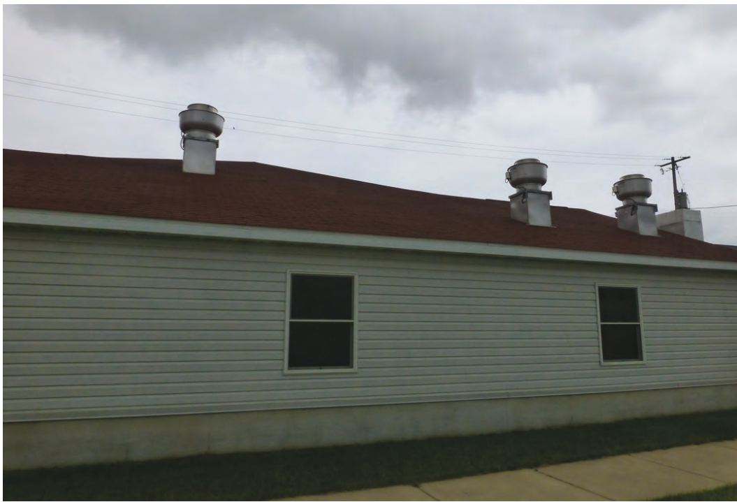
Photo 13. Close-up of replacement windows, vinyl siding, and newer roof ventilators (ERDC-CERL, 2018).
