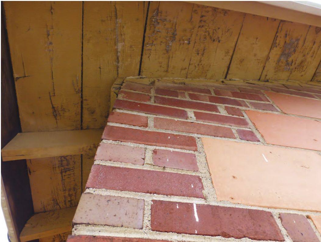
Photo 5. Close-up detail of exposed wood overhang eaves and rafters, and the brick and structural terra cotta tile wall in Building 2159 (ERDC-CERL, 2018).
