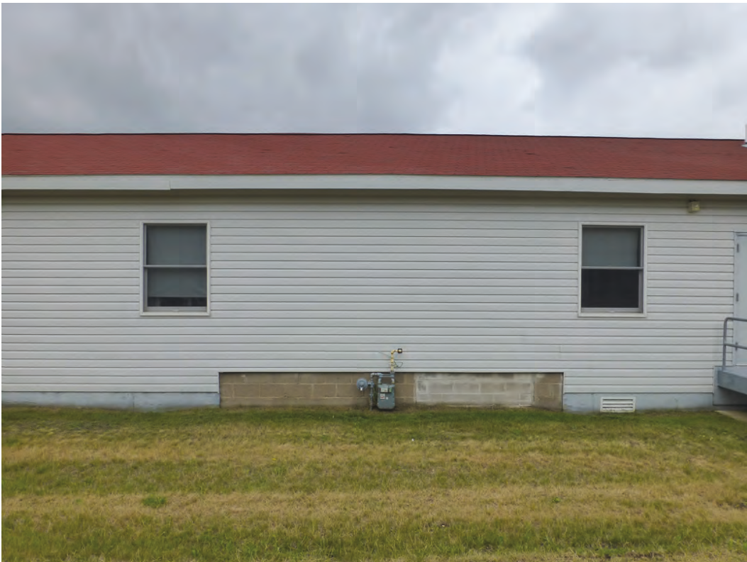
Photo 6. Concrete block foundation wall of the heater room on Building 1601 (ERDC-CERL, 2018).
