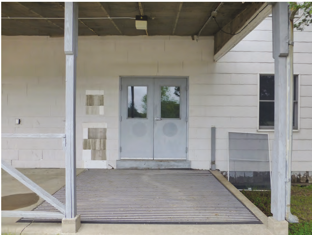
Photo 23. Typical replacement metal door with large pane on Building 2000 (ERDC-CERL, 2018).
