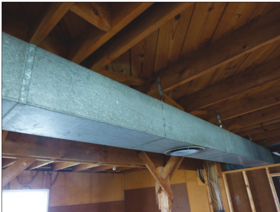
Figure 38. Metal heater duct in Building 1129 (ERDC-CERL, 2018).
