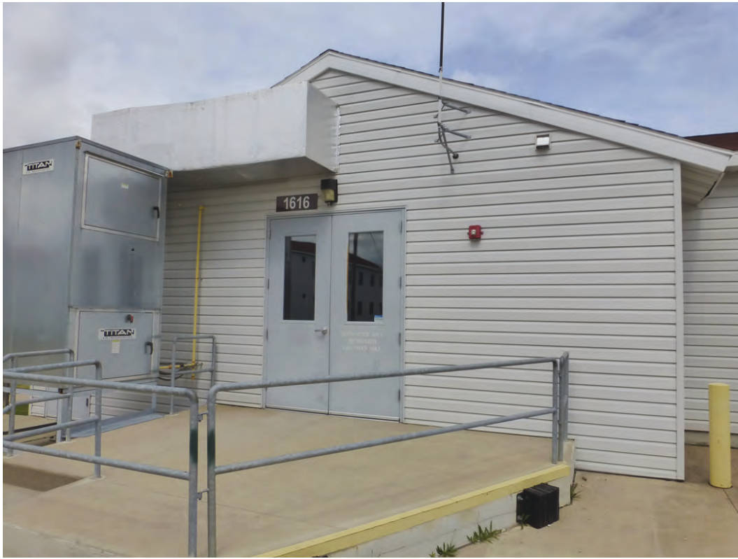
Photo 10. Close-up of replacement metal and glass entry doors and newer poured concrete ramp/steps with metal handrails used on both Buildings 1616 and 1617 (ERDC-CERL, 2018).
