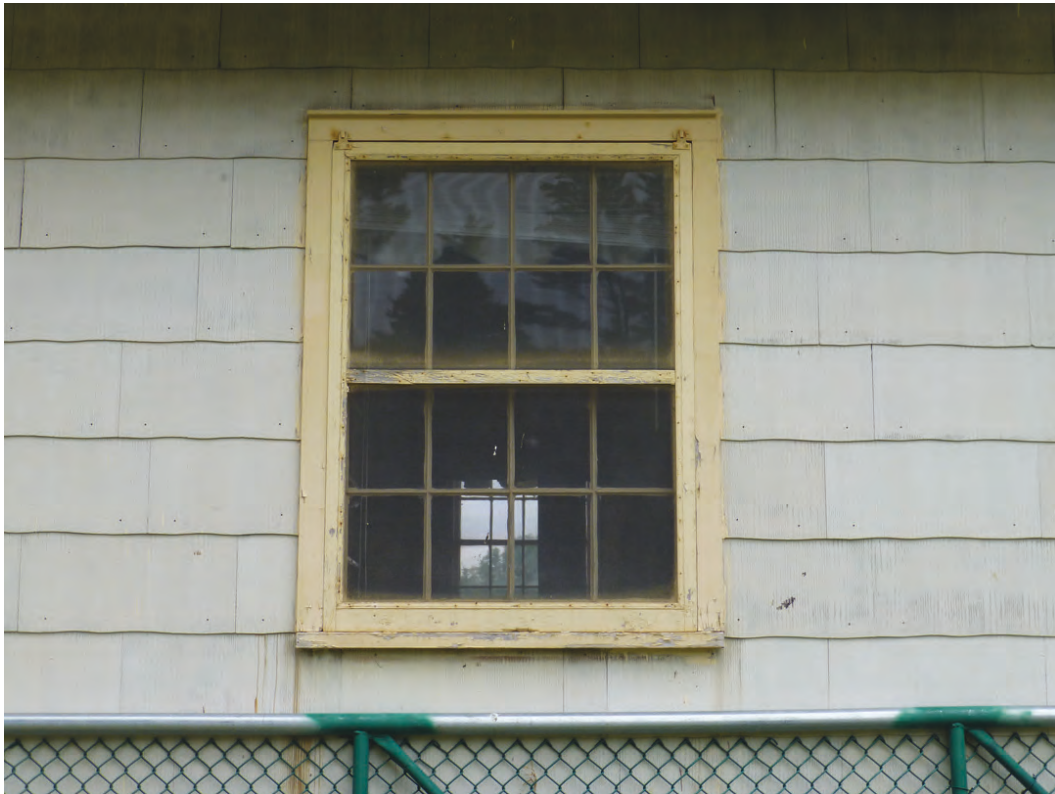
Photo 13. Original multipane wood double-hung window and wood screen on Building 550 (ERDC-CERL, 2018).
