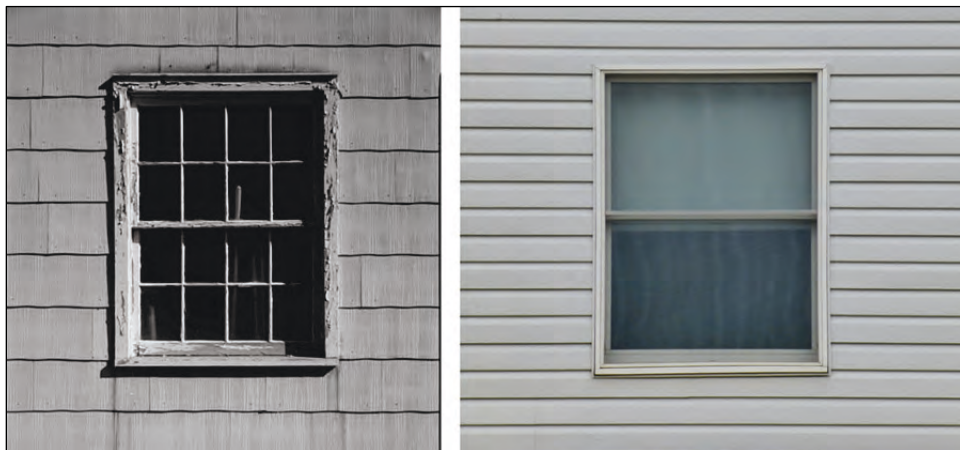
Figure 132. Window comparison of the original eight-over-eight wood double-hung window on a 74-man barracks (left) to the current replacement one-over-one vinyl window (right) (left: Library of Congress, HABS; right: ERDC-CERL).
