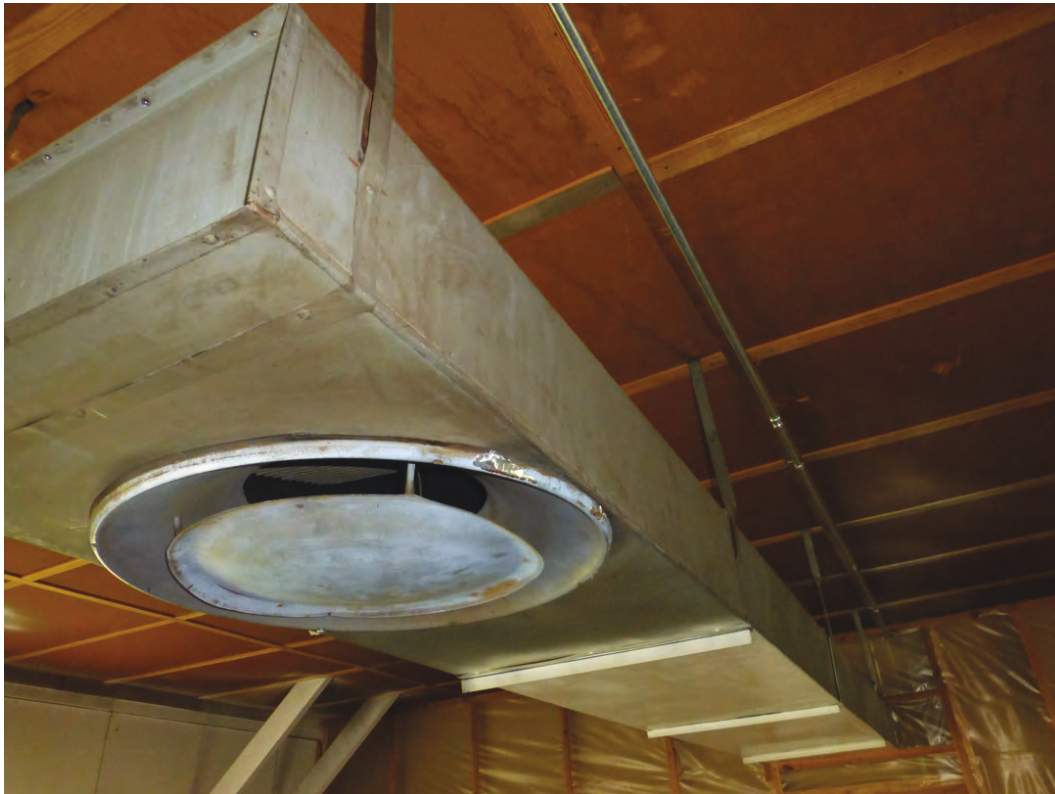
Photo 37. Original suspended mechanical and exhaust system in the squad room of Building 550 (ERDC-CERL, 2018).
