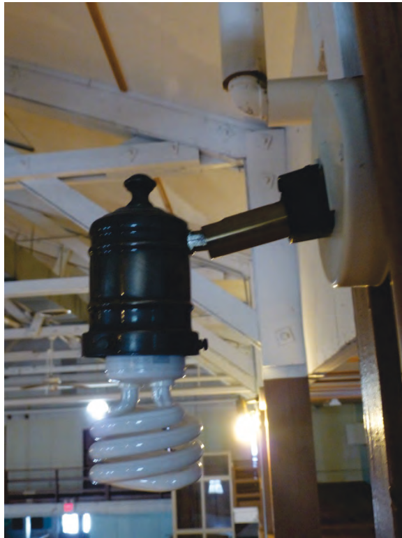
Photo 40. Replacement wall-mounted light fixture on the wood columns at the balcony level in the dance hall of Building 2000 (ERDC-CERL, 2018).
