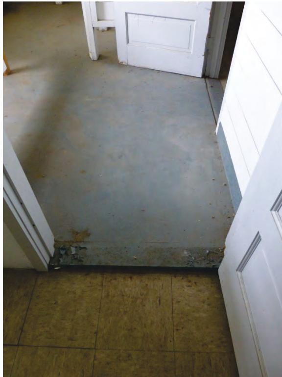
Photo 41. View of concrete floor of the latrine and the replacement tile floor of what originally was the NCO two-bunk room in Building 550. Note, this view shows a new modified door opening and new tile flooring in the bunk room (ERDC-CERL, 2018).
