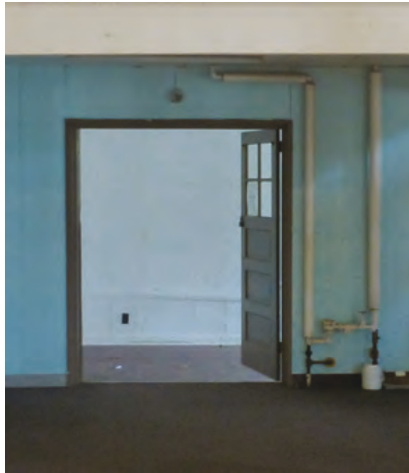
Photo 56. Original four-light, three-panel, wood interior door on the west wall of the dance hall in Building 2000 (ERDC-CERL, 2018).
