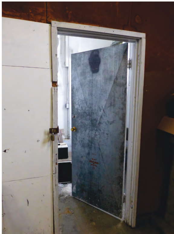
Photo 44. Original metal door into the work room from the apparatus room in Building 550 (ERDC-CERL, 2018).
