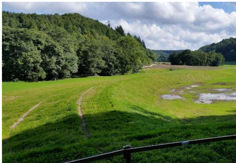
Top: View of completed low-level berm following revegetation of grasscrete surface. (Photo by Tom Nisbet, Forest Research)
