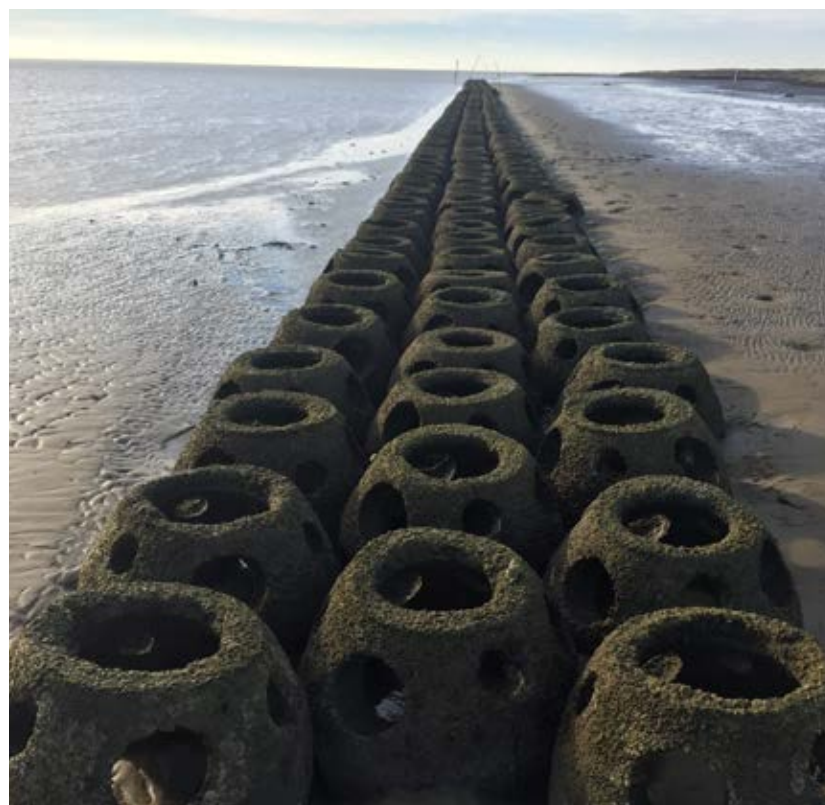
Bottom: Reef Balls form a breakwater. (Photo by Mary Kate Brown, The Nature Conservancy)
