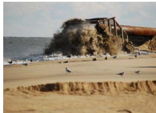
Below: The USACE Philadelphia District is renourishing Dewey, Rehoboth, and Bethany Beaches, Delaware, as part of a regular project in 20011–2012. Work was completed at South Bethany Beach, Fenwick Island, and Lewes, Delaware, in 2011. The projects are designed to reduce storm damage to public and private infrastructure. (Photo by Ann Cameron Siegal, USACE Philadelphia District)
