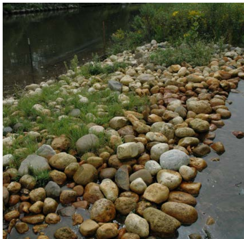
Bottom: Cobble bars help prevent erosion and stabilize the banks. (Photo by USACE Chicago District)
