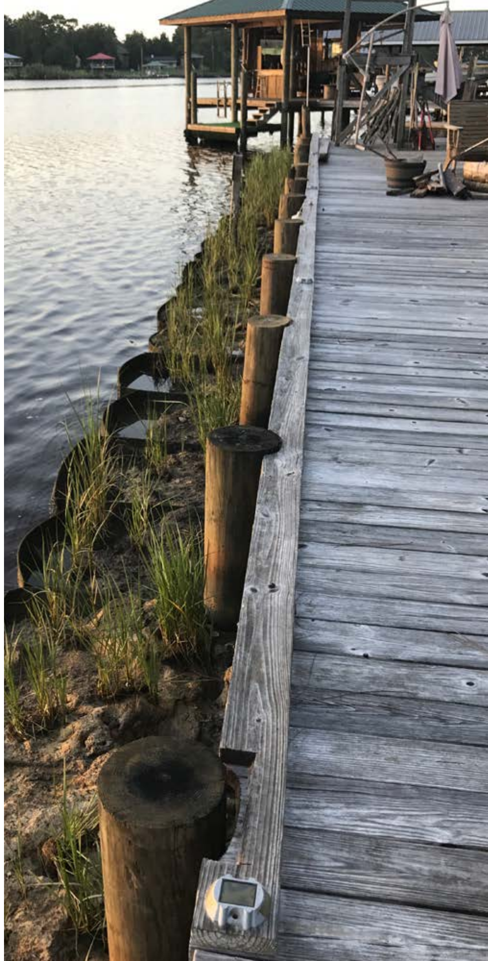
Previous page and right: Completed bulkhead retrofit with marsh grasses. (Photo by Jacob Blandford, The Nature Conservancy)
