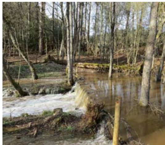
Top: View of completed low-level berm following revegetation of grasscrete surface. (Photo by Tom Nisbet, Forest Research)
