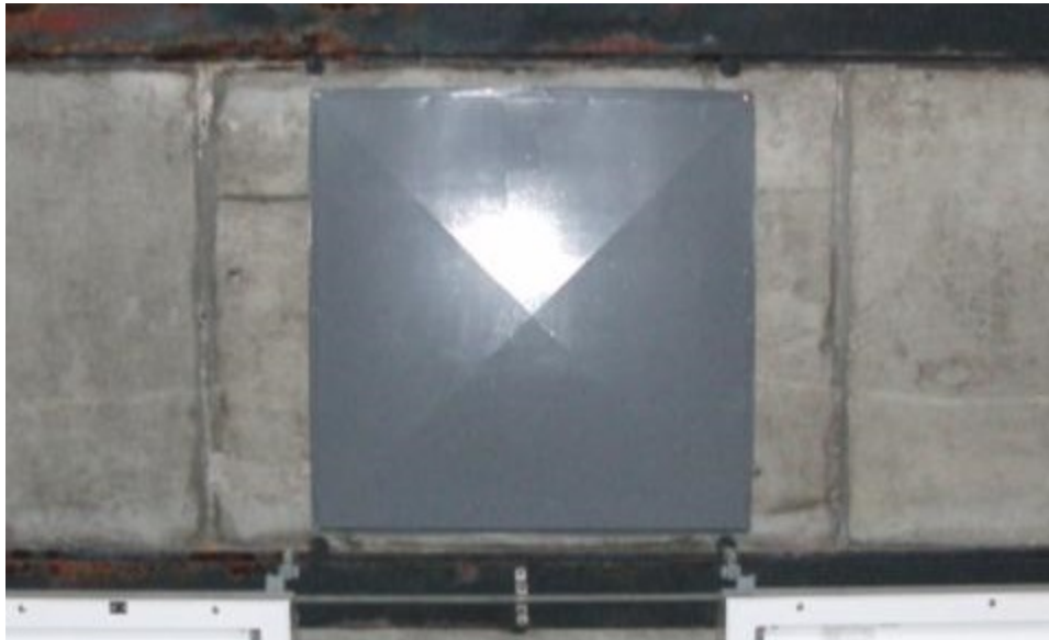
Figure 6. Roof vent cover.
