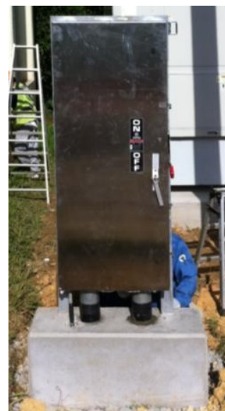
Figure 4. Disconnect switch.
