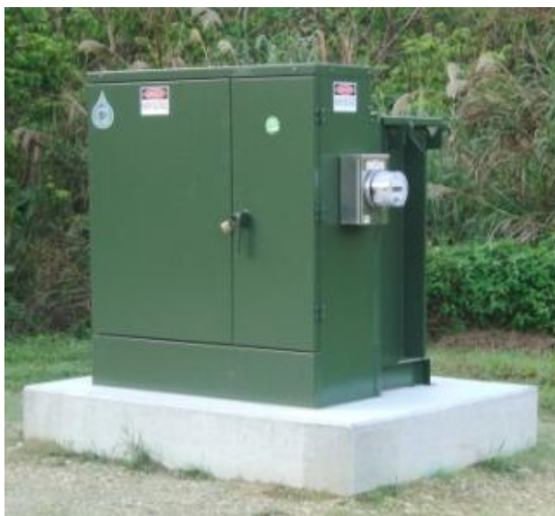
Figure 3. Transformer unit.
