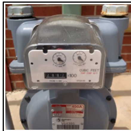
Figure 5-5. Existing utility gas meter for Bldg 1540A.
