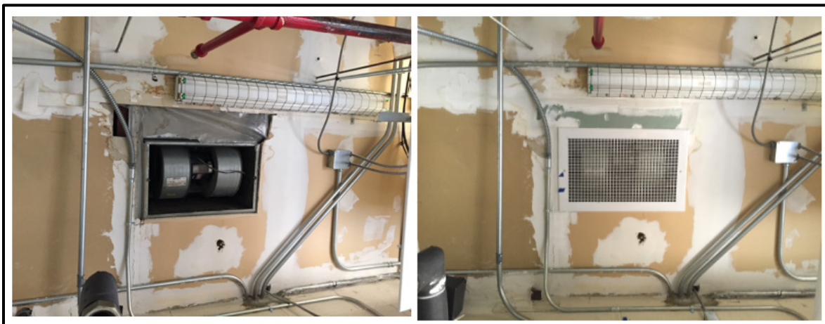
Figure 3-4. Sealing of leaks around an exhaust fan in the mechanical room.
