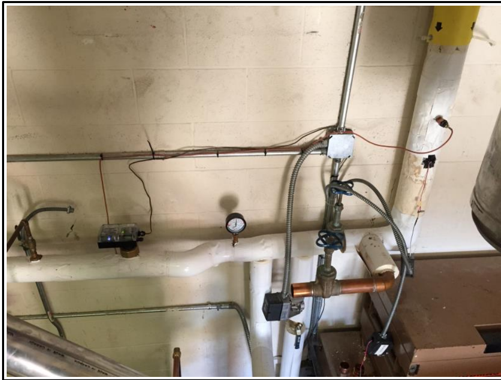
Figure 5-15. Boiler BTU meter as installed.
