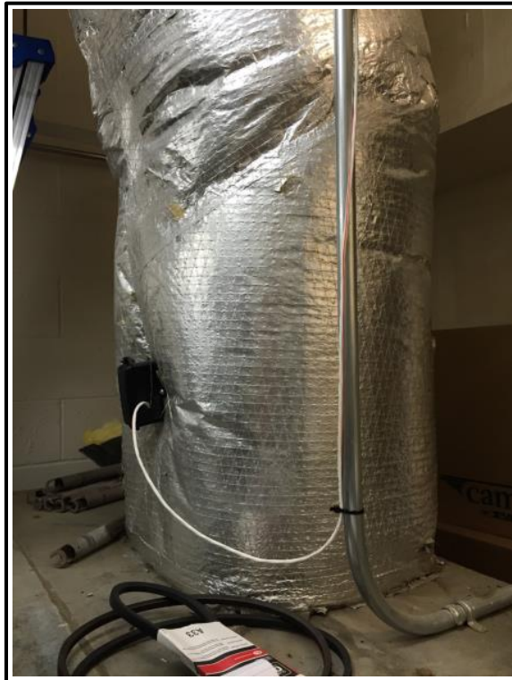
Figure 5-23. Supply air temperature AHU-4 duct sensor.
