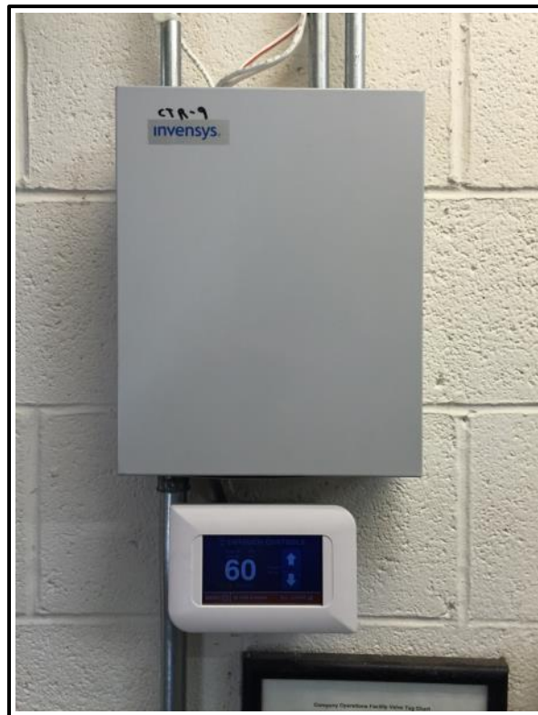
Figure 5-18. EMS master monitoring device with Global System for Mobile Communications (GSM) communication device.
