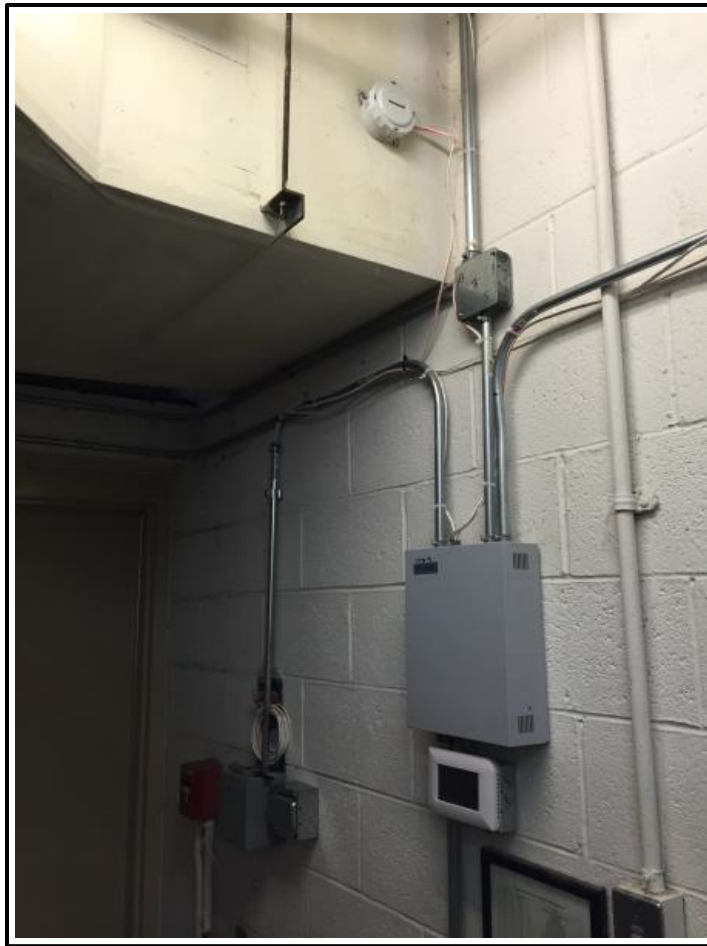
Figure 5-20. EMS installation within the Bldg 1540B mechanical room, showing EMS controller and outside air (OA) temperature sensor.
