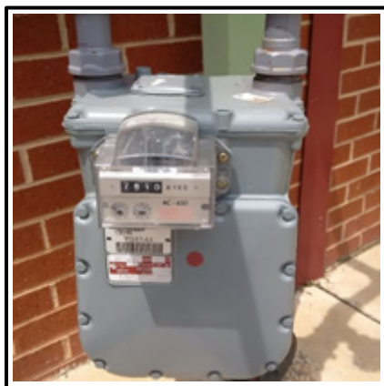
Figure 5-6. Existing utility gas meter for Bldg 1540B.
