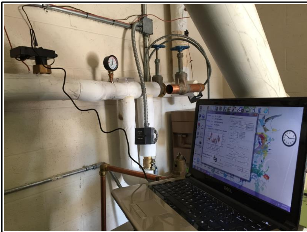
Figure 5-14. Boiler BTU meter connected to programming software.
