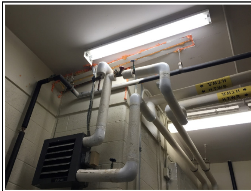
Figure 3-2. Leaks sealed at pipe hangers in “heated-only” portion of Bldg 1540A.
