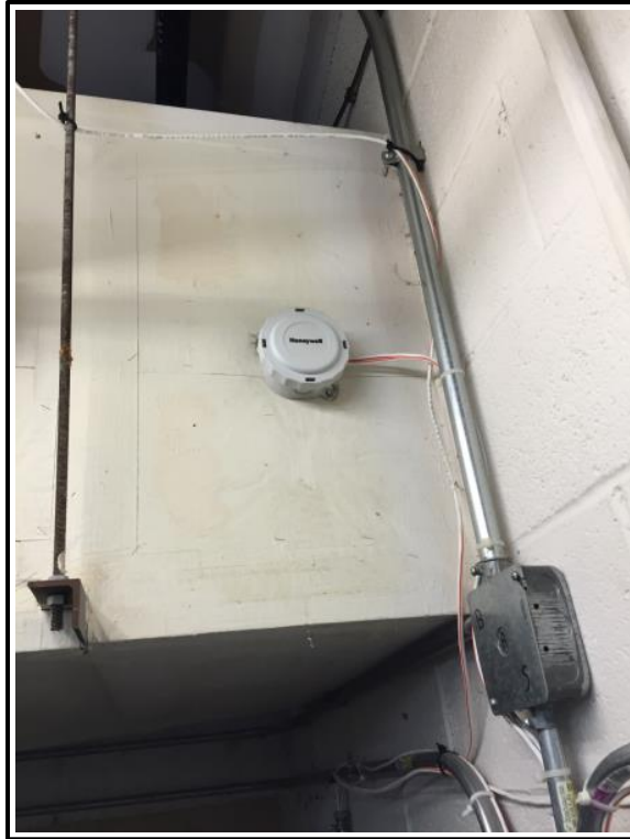
Figure 5-22. Outside air temperature sensor.
