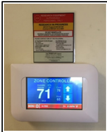
Figure 5-4. Typical room thermostat and RH sensor.
