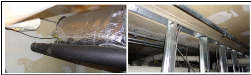
Figure 3-1. Leakage sources at pipe penetrations and at framing systems.
