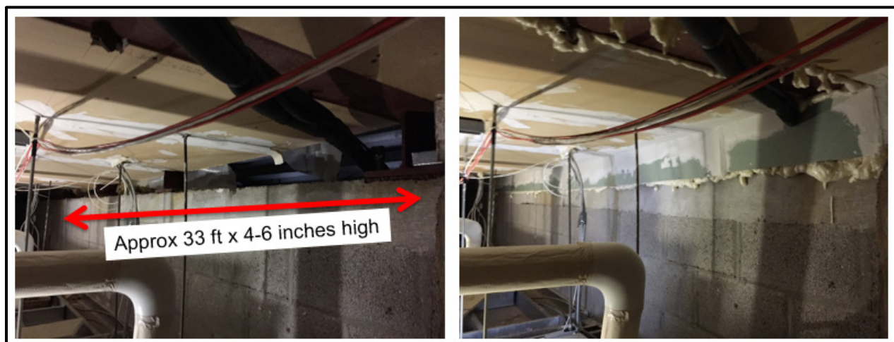
Figure 3-5. Sealing of a major opening above the hard ceiling above the men's latrine.
