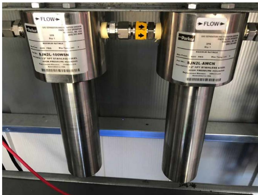
Figure 12. Parker High Pressure Filters
