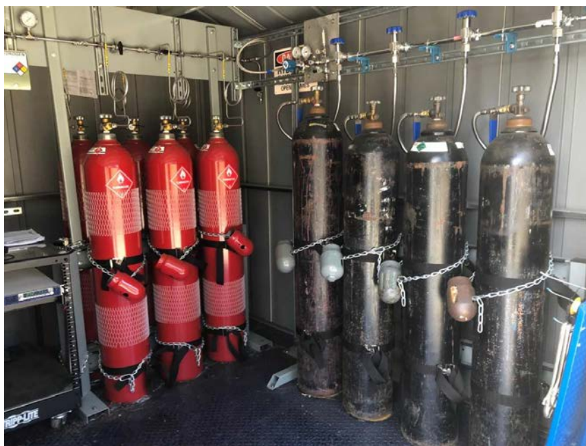
Figure 13. High Pressure Hydrogen Storage Tanks (left) and Nitrogen Storage Tanks (right)
