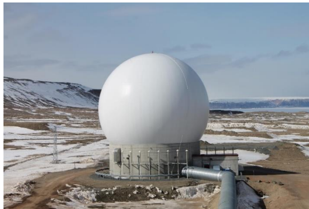
Figure 5: AFSCN Antenna at Thule Air Base, Greenland (26)
