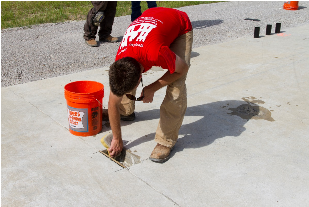
Figure 16. Applying water as bonding agent (saturated surface dry condition).
