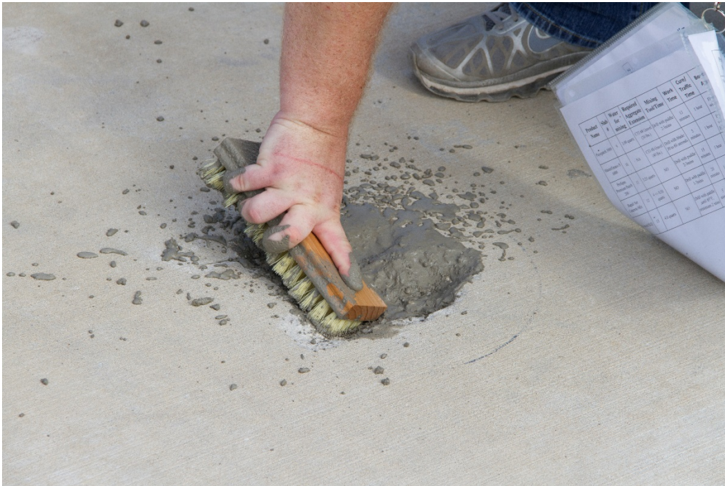
Figure 17. Scrubbing repair material mortar onto the repair perimeter.
