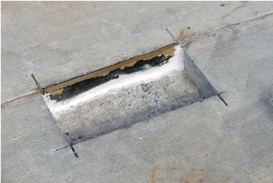
Figure 13. Example of final spall “popout” repair.
