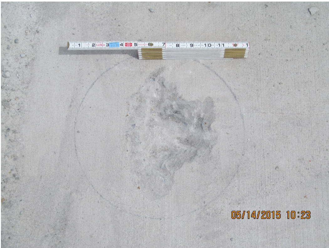
Figure 13. Example of final spall “popout” repair.
