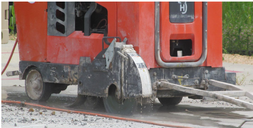
Figure 4. Saw cutting existing joints to meet airfield specifications.
