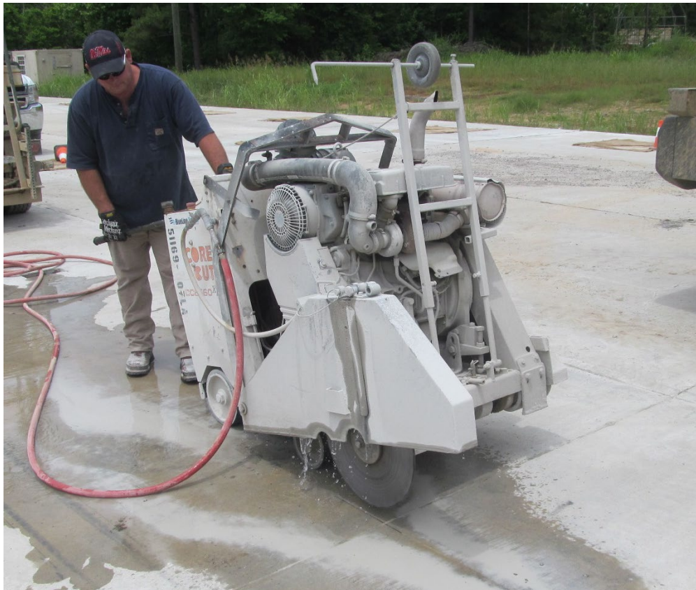
Figure 6. Cutting out joint spall repairs with a wet saw.
