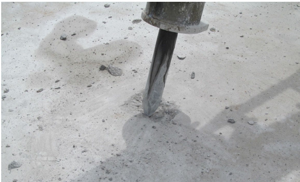
Figure 11. Jackhammer attachment (moil point) used to create “popout” spall repairs.
