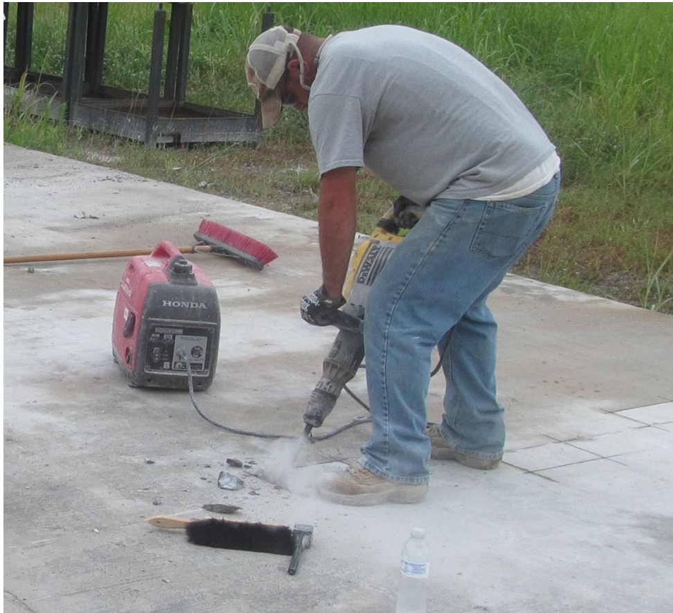
Figure 8. Removing concrete from joint spall cutouts with a jackhammer.
