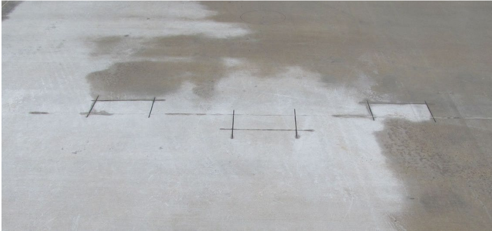
Figure 7. Concrete wet saw cutouts for joint spall repairs.
