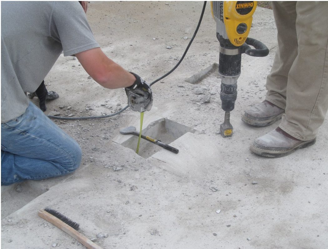
Figure 9. Achieving desired, constant depth of joint spall repairs using a bushing bit.
