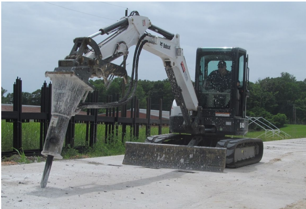
Figure 11. Jackhammer attachment (moil point) used to create “popout” spall repairs.
