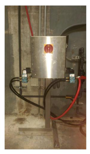
Figure 1 – Strainer power supply box
