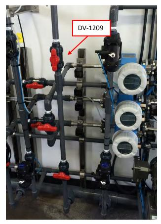
Figure 3 - Feed Flow Pipe and Valves
