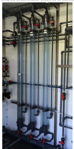
Figure 6 - Pressure Relief Water Columns
