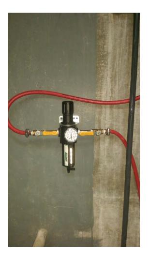
Figure 2 – Air supply valves in the "open" position
