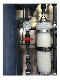
Figure 2 – Pressure gauge of the intake of ambient air next to the hollow fiber membrane.
