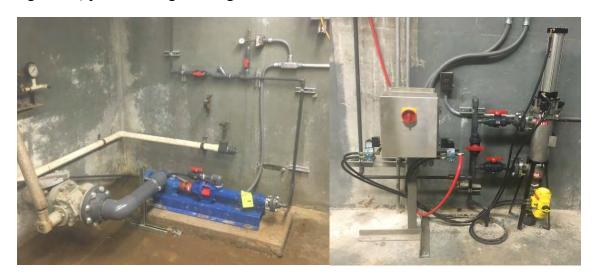
Figure 5.2 Feed Pump and Strainer for the Gas-sparged AnMBR.
