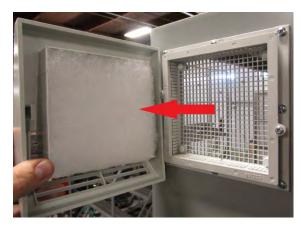
blow out with compressed air until clean. Re-install in reverse order of removal.
