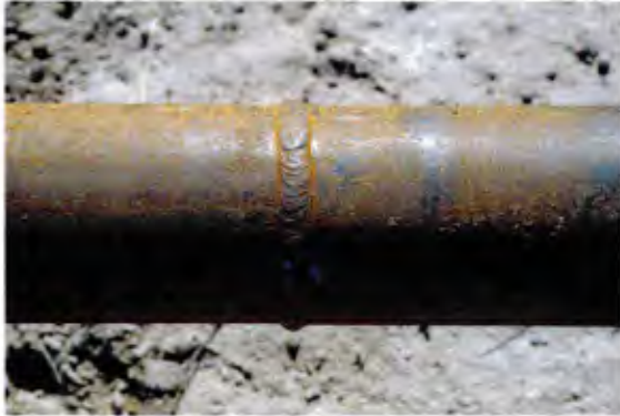
Close-up of pipe weld: Notice flash rusting.
