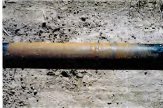
Pipe surface requiring field coating.
