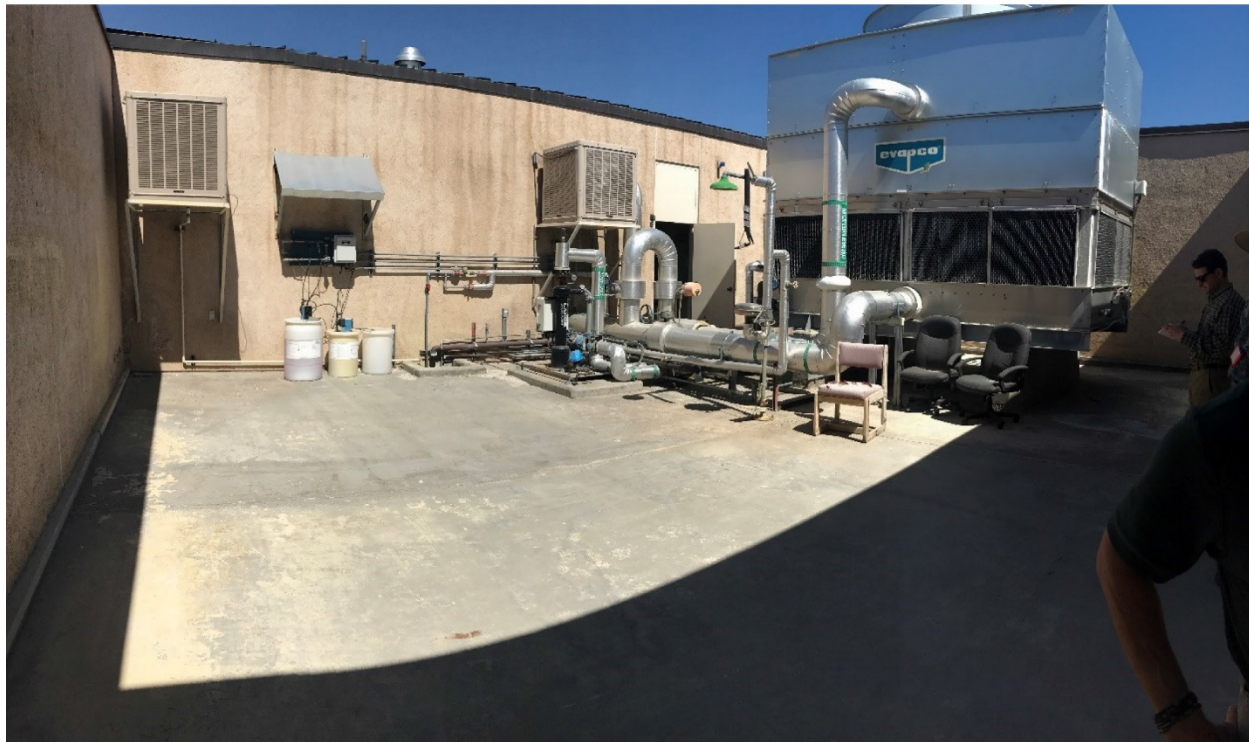
Figure 4. Interior of Fort Irwin Building 263 enclosure.
