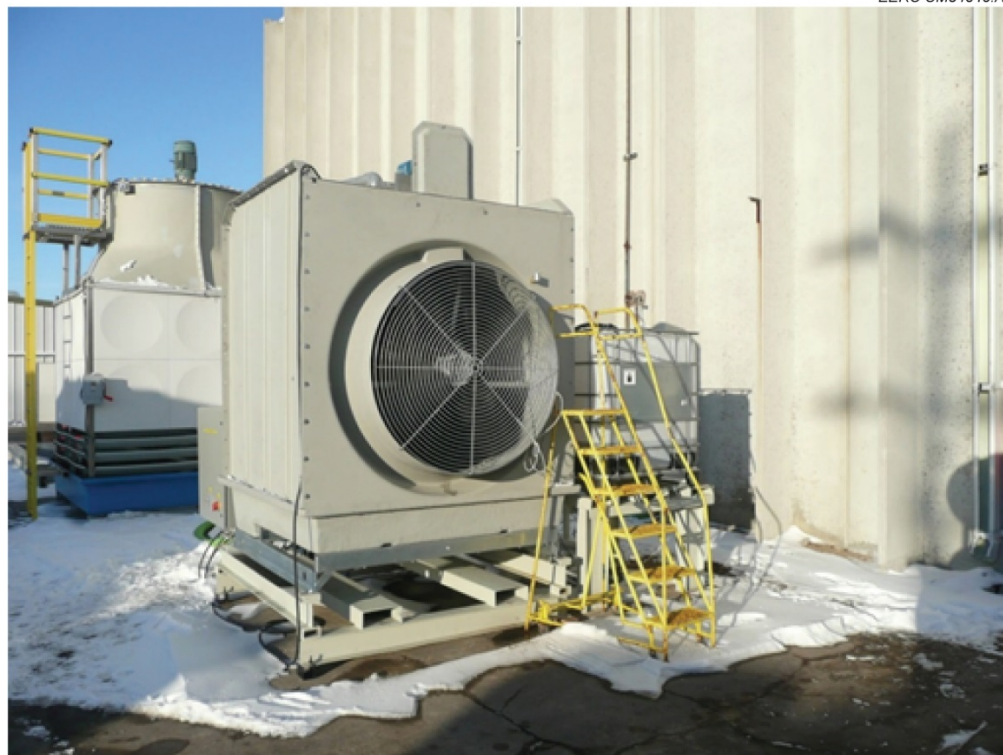
Figure 11. Front view of tower, pump skid, filter skid, and makeup tank.
