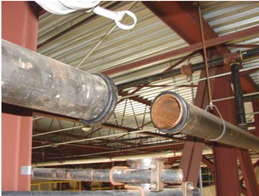
Figure 2. Deluge system with tee removed.
