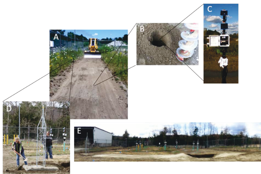
Figure 3. Preparation of the field site. A) Heavy equipment used to create soil lanes. B) Hole for soil moisture and temperature probes. C) Data loggers for probes. D) Installation of towers to host sensor-suites. E) Field site with sensors.
