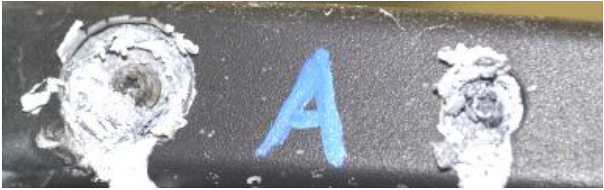
Figure 2: Galvanic corrosion effects of steel screws in a magnesium component exposed to 240 hours of ASTM B117 salt spray testing.
