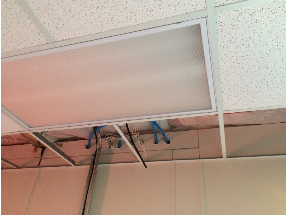
Figure 23. Conduits Installed in Building A6372 for Network Wiring
