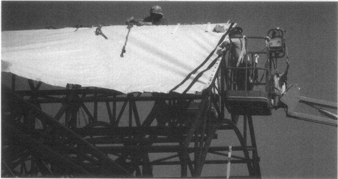
Figure 3. Fastening of one end of a membrane to the finished steel frame structure. Pg. 149 (C. G. Huntington)
