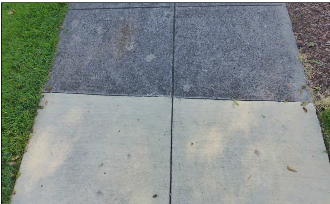
Figure 128. Detail of older, high-aggregate concrete (background) compared to the low-aggregate concrete installed in 2015 (foreground) on the sidewalk leading to the Superintendent's Lodge, 2017 (ERDC-CERL).
