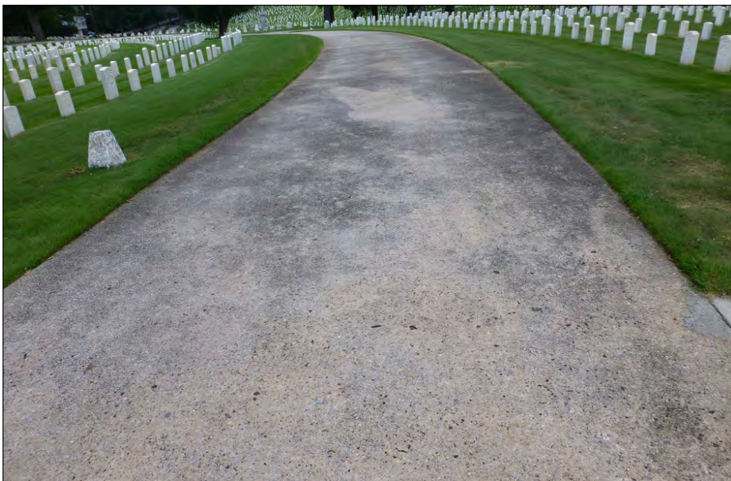
Figure 125. View looking east between Sections C [left] and G [right], showing the older, high-aggregate concrete road paving with no curbing that was installed in 1931 (ERDC-CERL, 2017).
