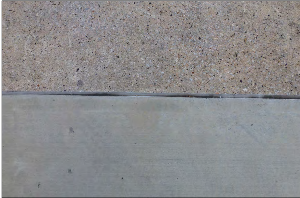
Figure 126. Detail of the low-aggregate concrete road paving installed in 2015 on the bottom of the photo, versus the high-aggregate concrete road paving shown at the top of the photo, installed in 1931 (ERDC-CERL, 2017).
