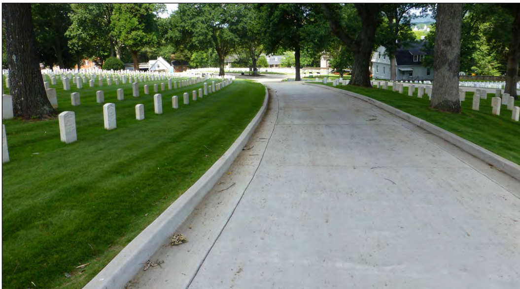
Figure 121. View looking northwest between Sections A [left] and B [right] toward the Superintendent's Lodge, showing the low-aggregate concrete road paving and curbing installed in 2015, 2017 (ERDC-CERL).
