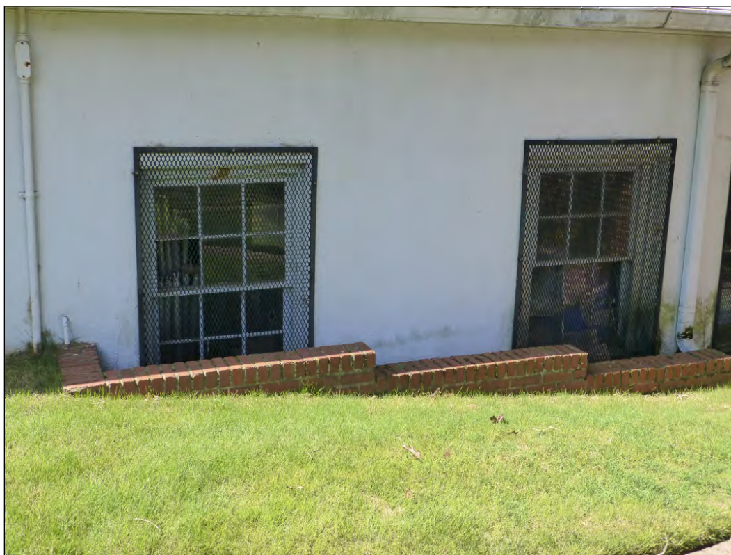
Figure 136. North side of the utility building, showing how it was constructed into the hill with a brick retaining wall, 2017 (ERDC-CERL).
