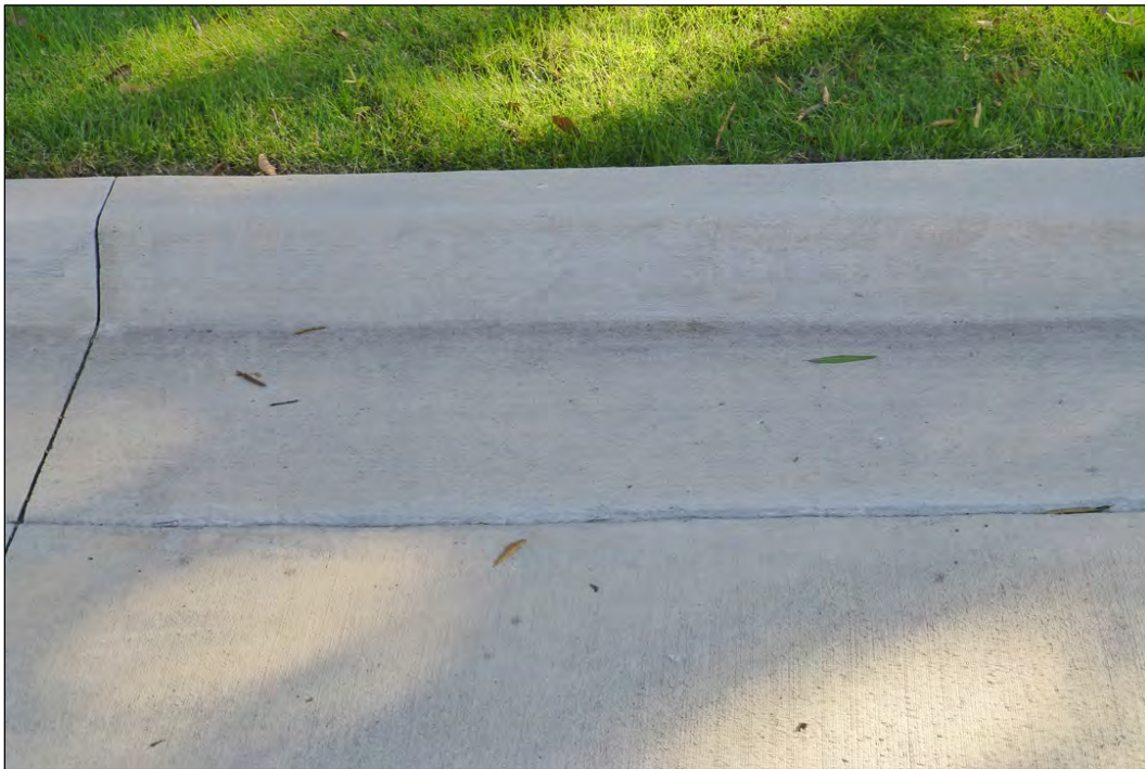
Figure 122. Detail of the low-aggregate concrete road paving and curbing installed in 2015 (ERDC-CERL, 2017).
