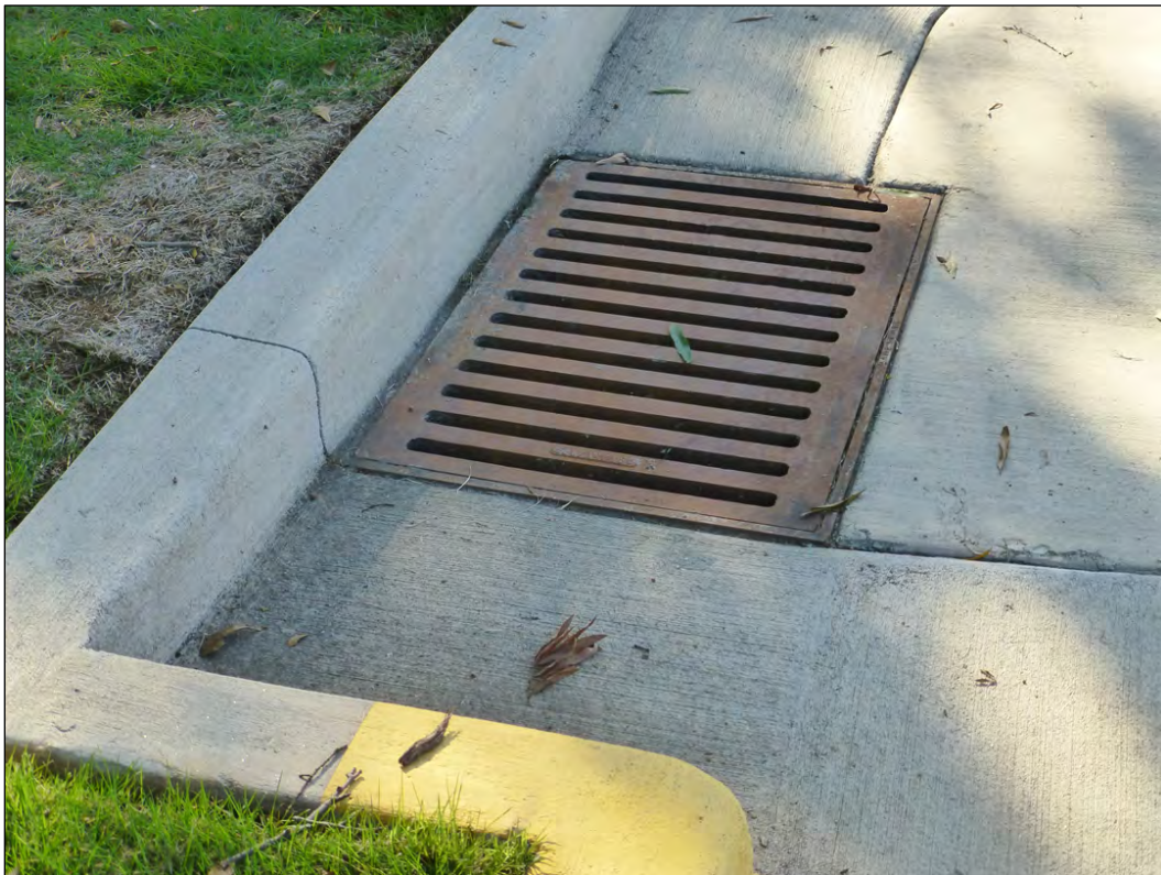
Figure 123. Detail of the low-aggregate concrete road paving, curbing, and storm drain grate installed in 2015 (ERDC-CERL, 2017).
