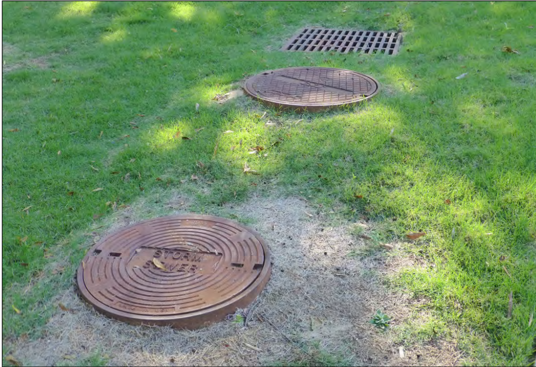
Figure 194. Storm drain and storm sewer manhole access, 2017 (ERDC-CERL).
