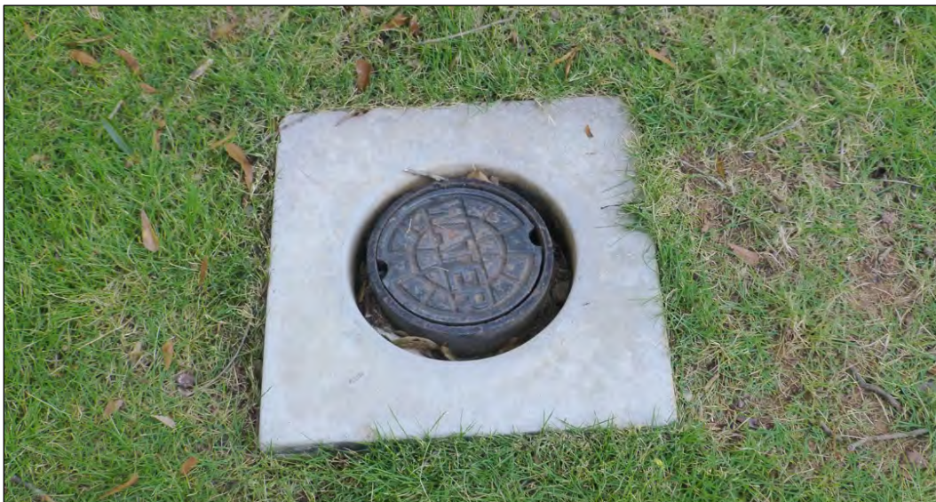
Figure 191. Water shutoff set within stone, 2017 (ERDC-CERL).
