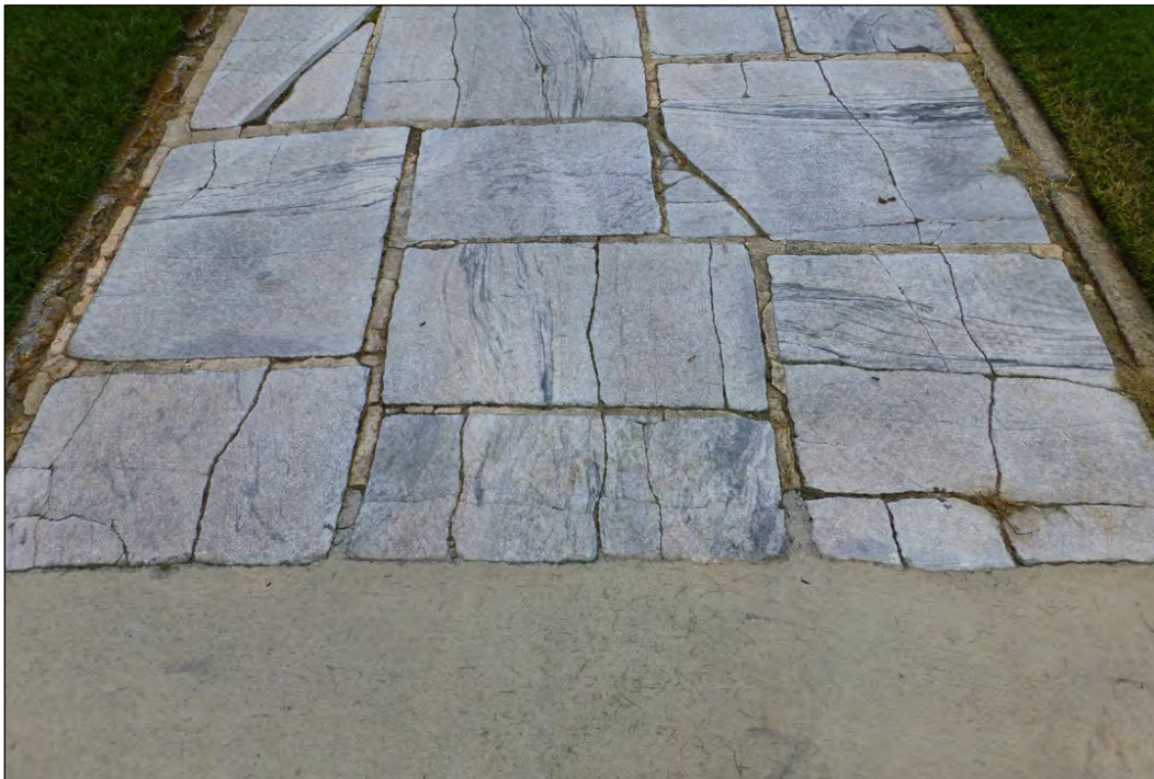
Figure 131. Detail of the portion of the flagstone path in Section U, where the low-aggregate concrete was used in 2015 (ERDC-CERL, 2017).
