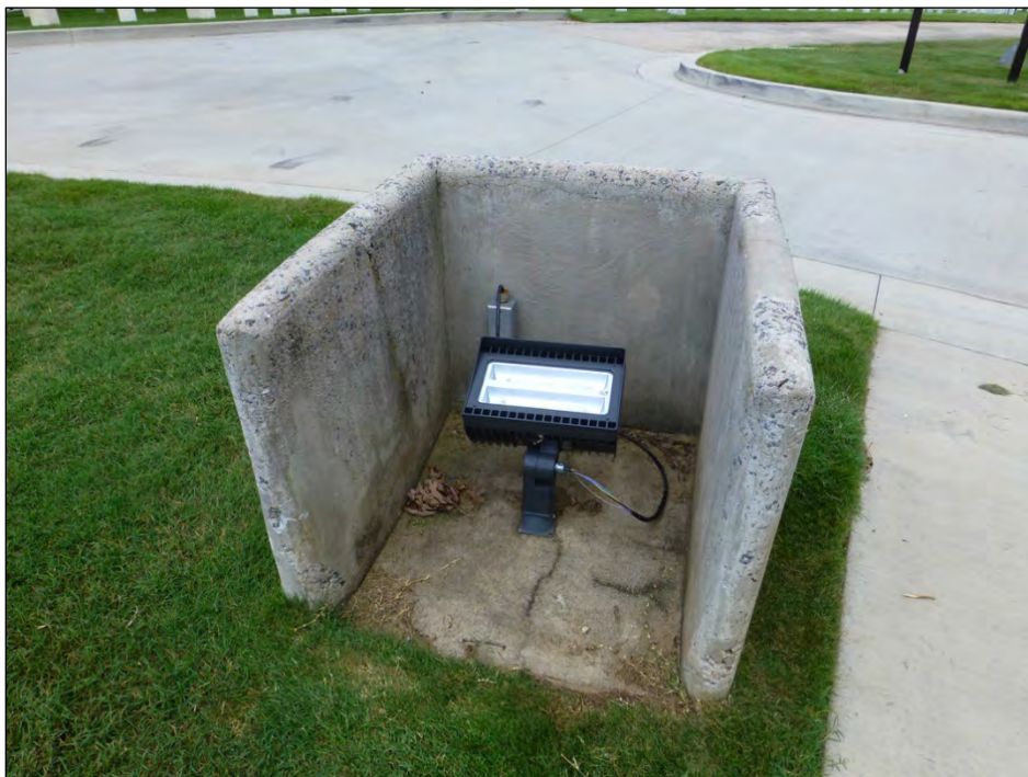
Figure 196. Concrete screen for flagpole floodlight, 2017 (ERDC-CERL).
