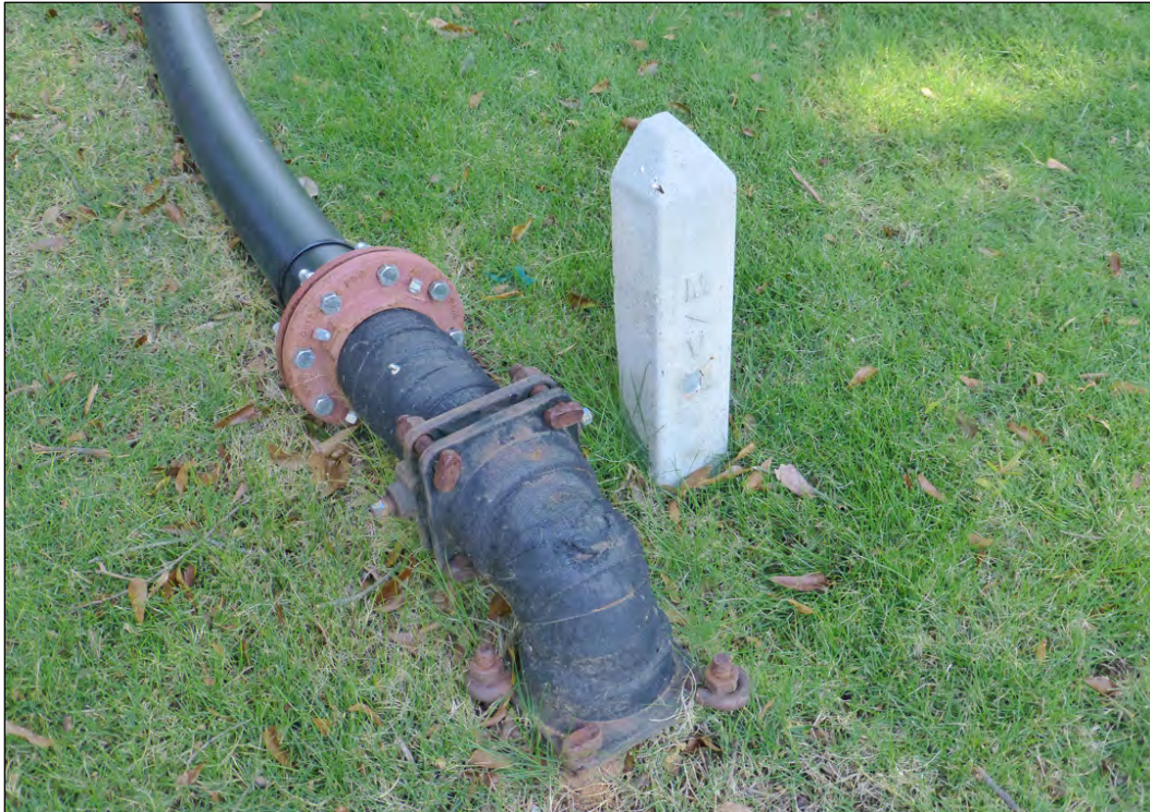
Figure 190. Standpipe for sprinkler system with rubber hose, 2017 (ERDC-CERL).
