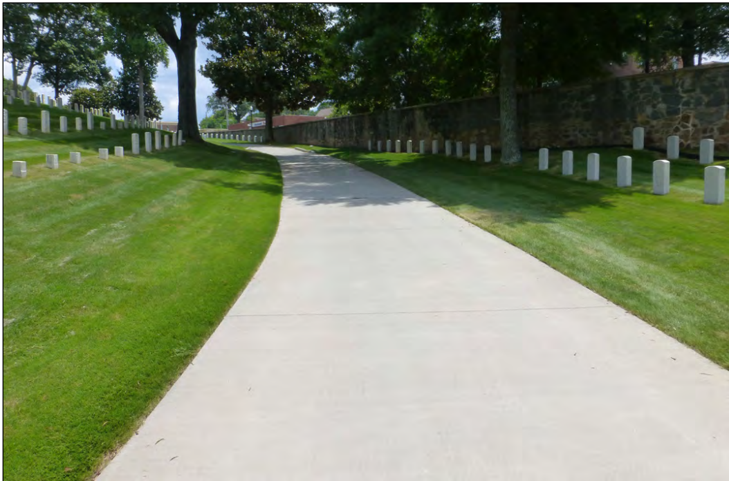
Figure 124. View looking east between Sections H [left] and J [right] showing the low aggregate concrete road paving with no curbing installed in 2015 (ERDC-CERL, 2017).
