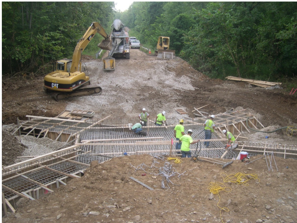
Figure 8. Bridge 42 during construction.
