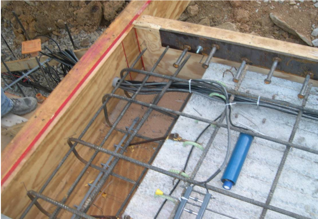
Figure 2. Corrosion potential reference electrodes (blue).
