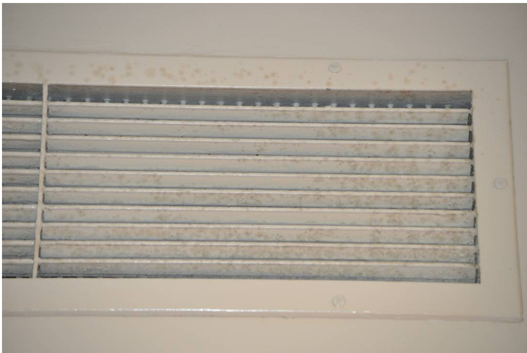
Figure 38. Air vent in Room 11, after 12 months.
