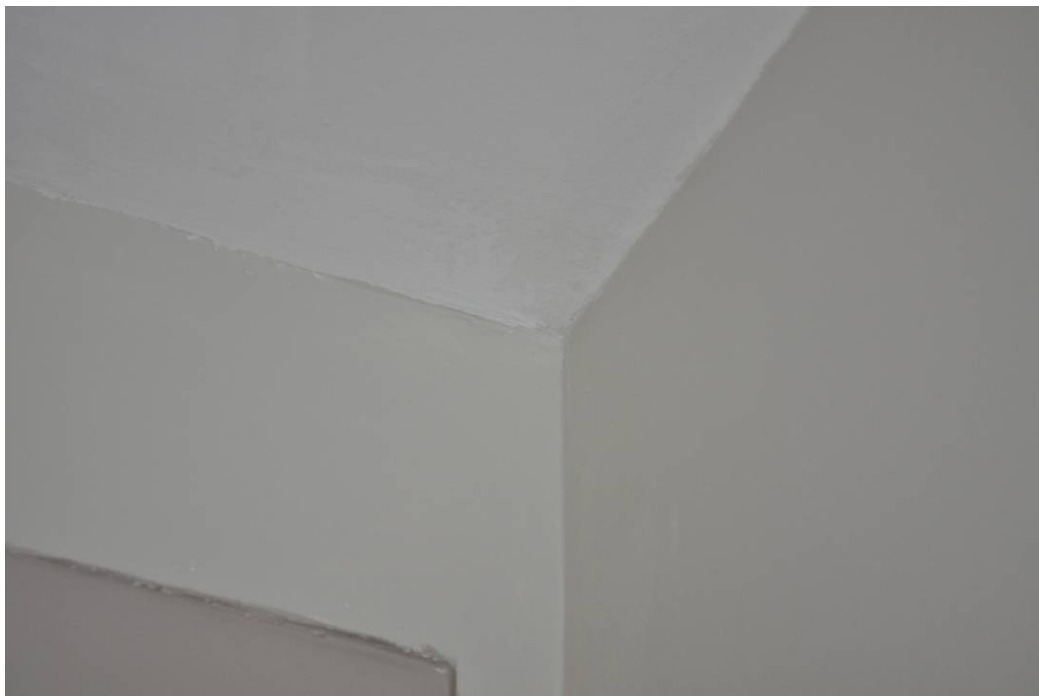
Figure 10. Walls in Room 4 coated with an unknown coating, and ceiling coated with Foster 40-20 after 4 months.
