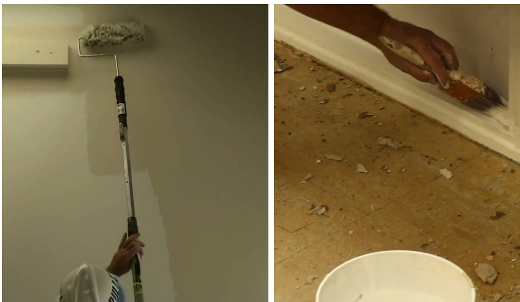
Figure 5. Coating application using 1-inch nap roller (left) and nylon brushes (right) for Sherwin Williams and Hirshfield's coatings.
