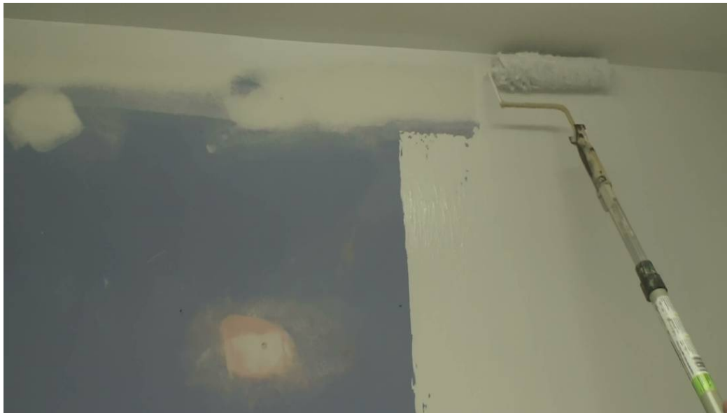
Figure 4. Sherwin Williams ProMar 200 acrylic primer applied to new gypsum board installed in Room 9.
