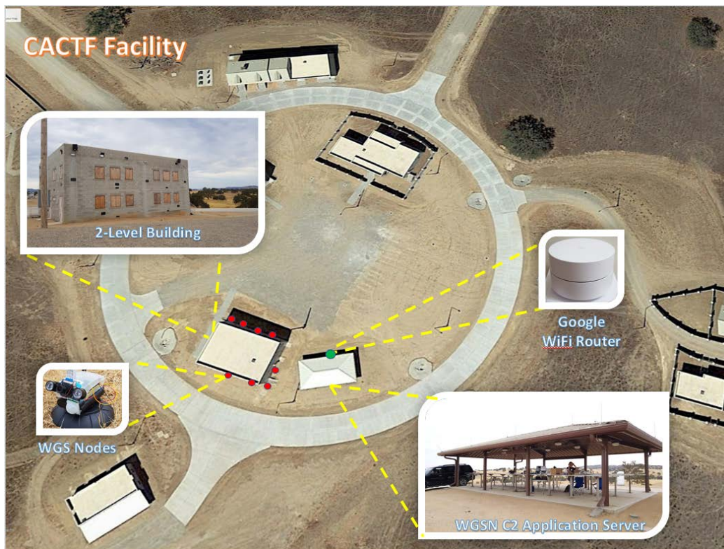
CACTF Facility, Camp Roberts, Lat 35.765090 and Lon -120.769728. Image retrieved from Google Earth, June 14, 2017.
