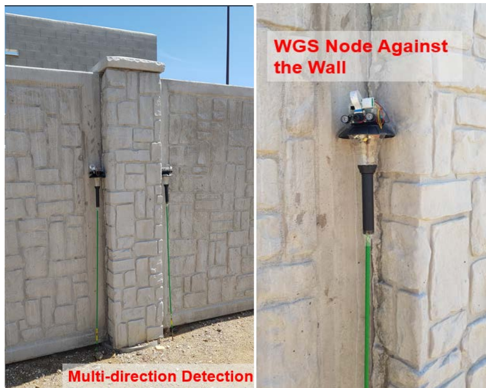
Figure 55. WGS Node Deployed against the Building Boundary Wall
