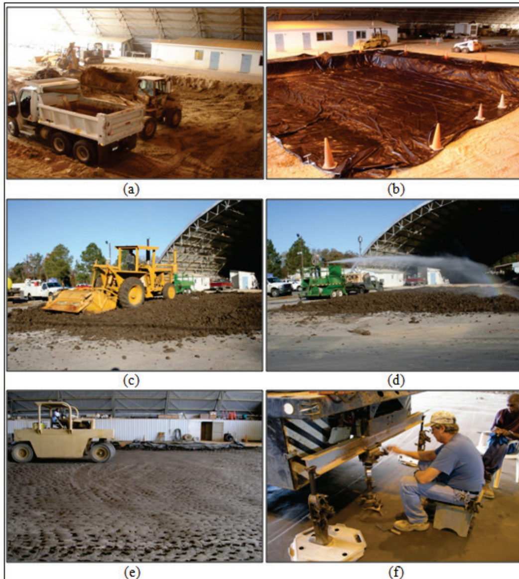
Figure 21. Full-scale test section construction sequence (a) Excavating test area in covered pavement test facility, (b) Lining pit with plastic to prevent moisture migration, (c) Mixing soil to achieve uniform moisture, (d) Adding water to adjust moisture content, (e) Compacting processed and installed subgrade material, and (f) Performing field CBR tests to ensure desired value was achieved.
