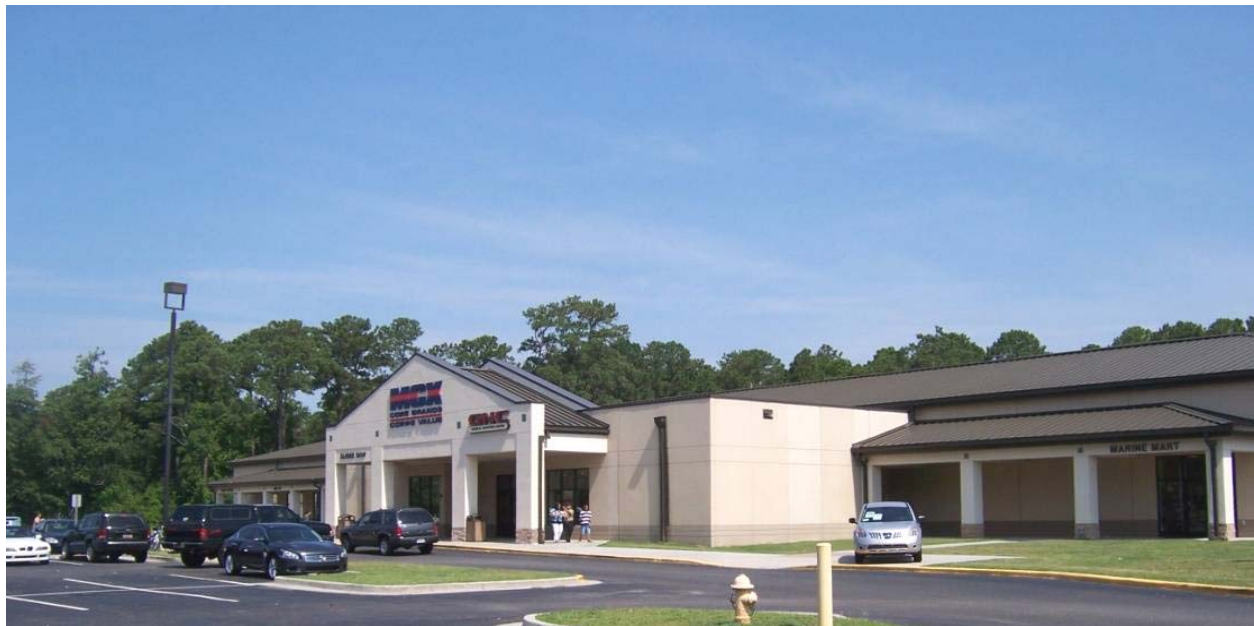
Figure 7. Building 1283 Base Exchange at MCAS Beaufort.
