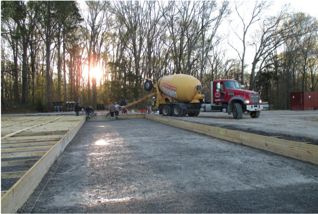
Figure 6. Placing PCC in Lane 3.
