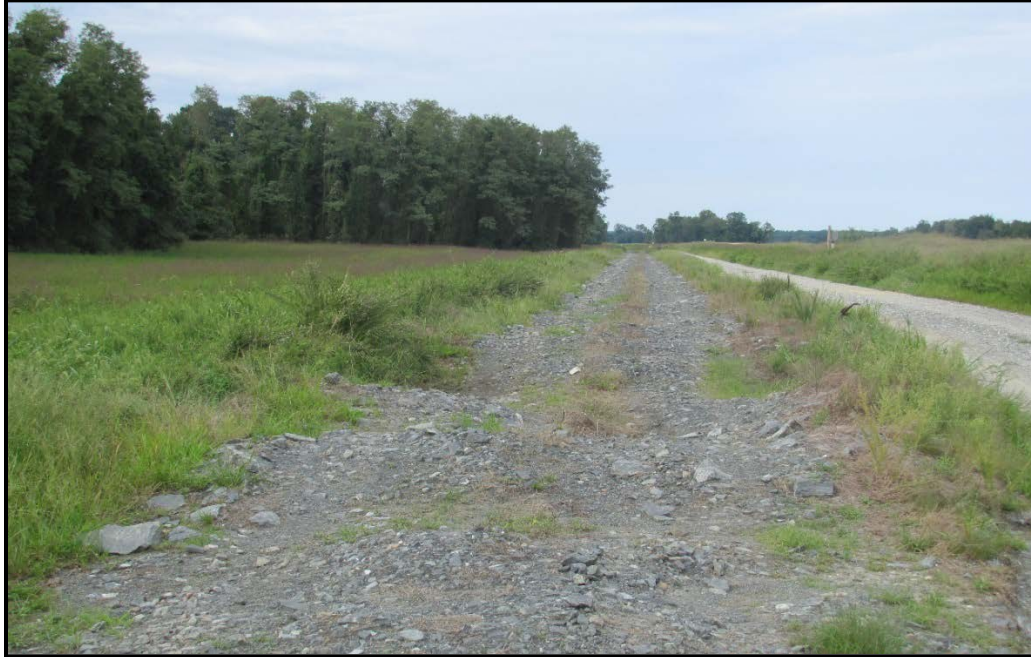
Figure 78. View of Perryman No. 5 Course.
