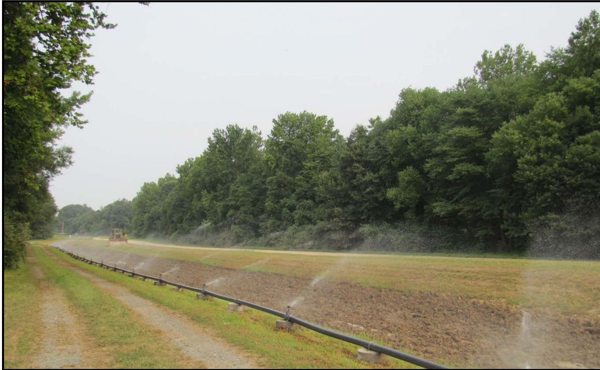
Figure 79. Mud Bypass Course with sprinklers operating.
