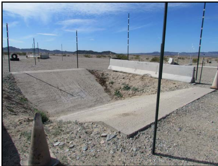
Figure 148. Direct approach V-ditch.
