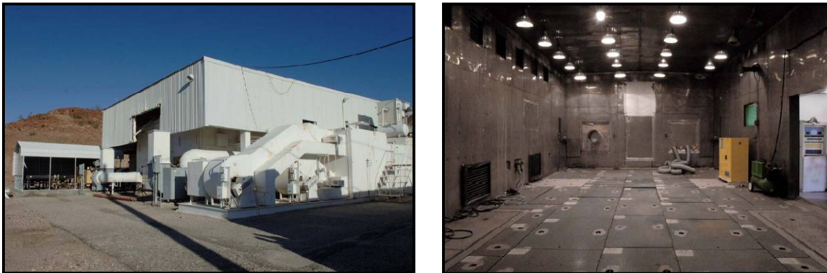
Figure 177. Outside view of LMPEC (left) and view into LMPEC from access door opening (right).
