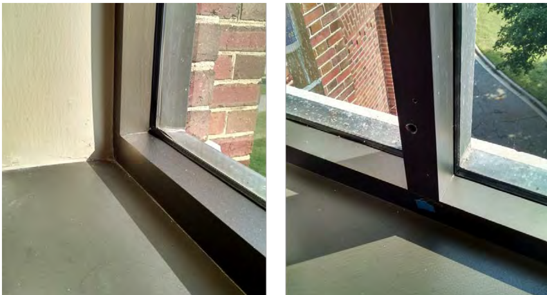
Figure 7. Single Pane Glazing at the Site, Pre-demonstration
