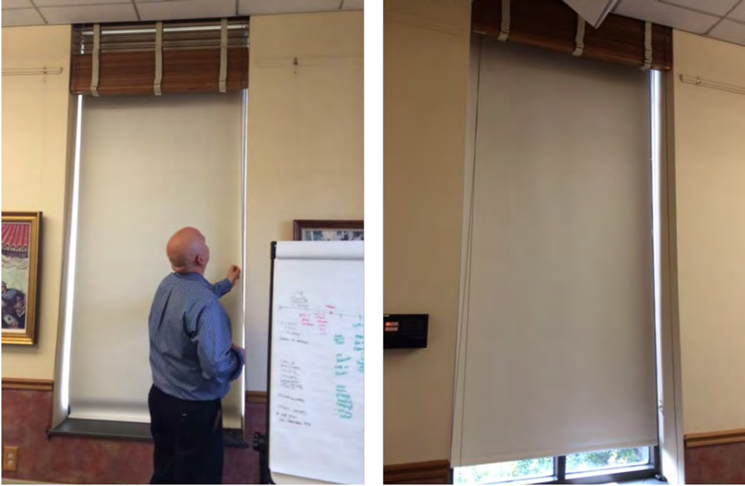
Figure 8. Dual Blind Treatments Typical of all Existing Windows
