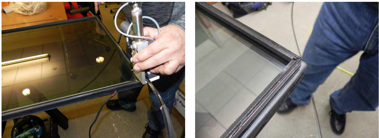
Figure 21. Perimeter Spacer / Seal was Applied at Site
