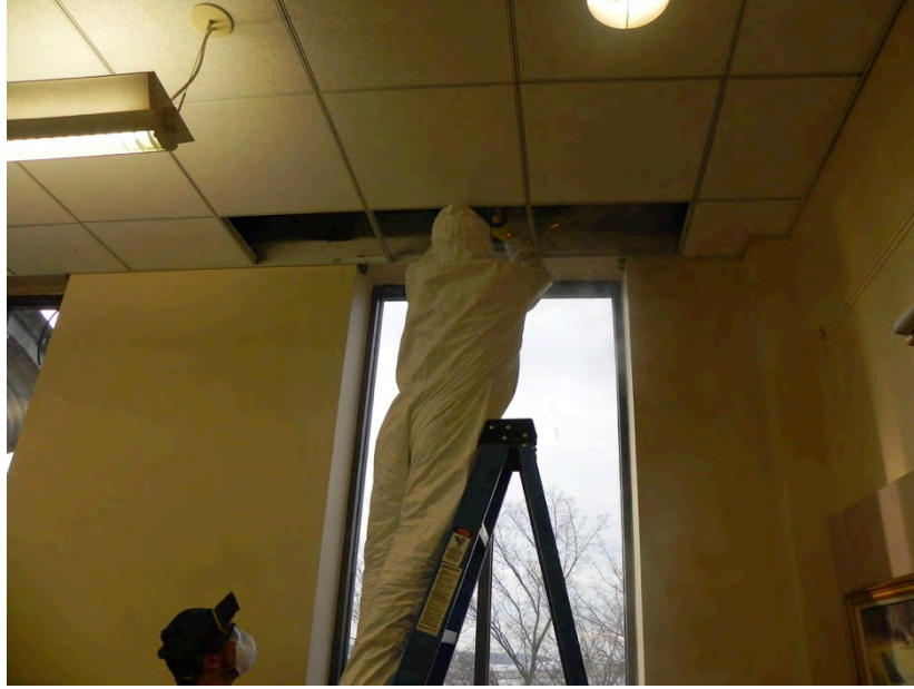
Figure 17. Installation of Dynamic Glass System Components in the Existing Ceiling Plenum
