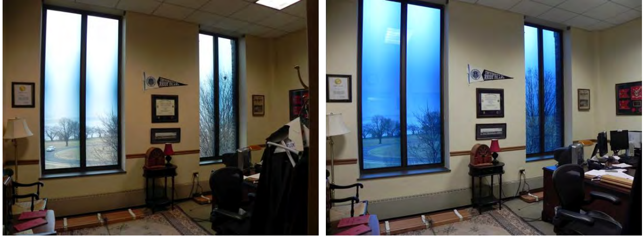
Figure 24. Glass Appearance as Commissioned – During Tint Transitioning
