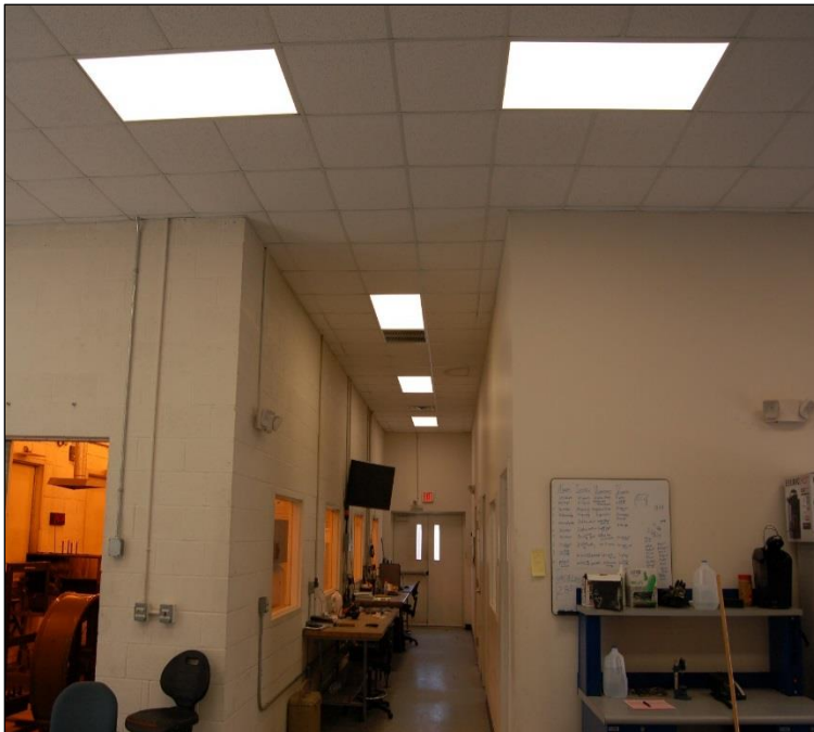
Figure 1-12. Upgraded Sylvania LEDVANCE lighting in Building 734.
