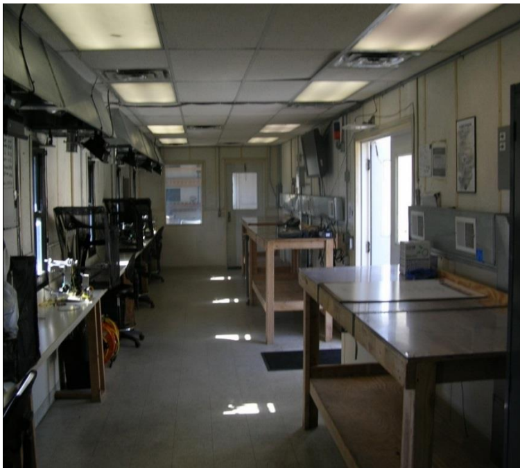
Figure 1-8. Fluorescent lighting at firing positions in Building 738A.
