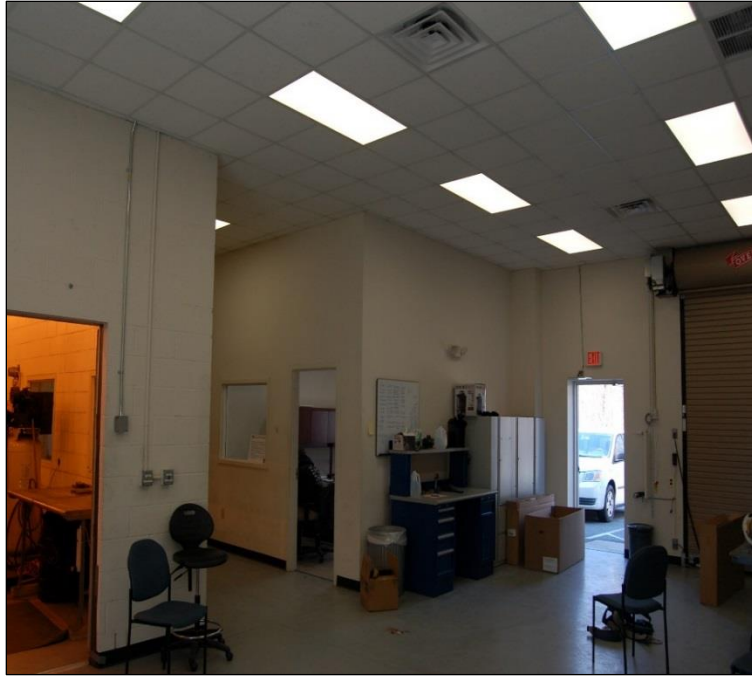
Figure 1-13. Upgraded Sylvania LEDVANCE LED lighting in Building 734.
