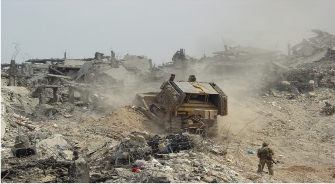
Figure 9. The D 9 Bulldozer Opening a Road above the NBC Ruins
