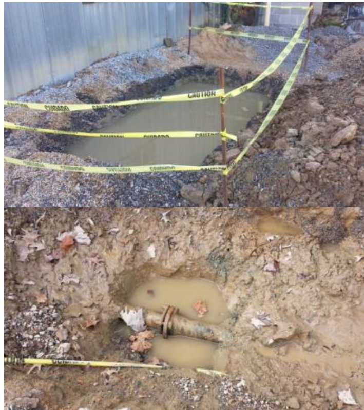
Figure 6-13. Excavation of the Large Leak Identified at ERDC
