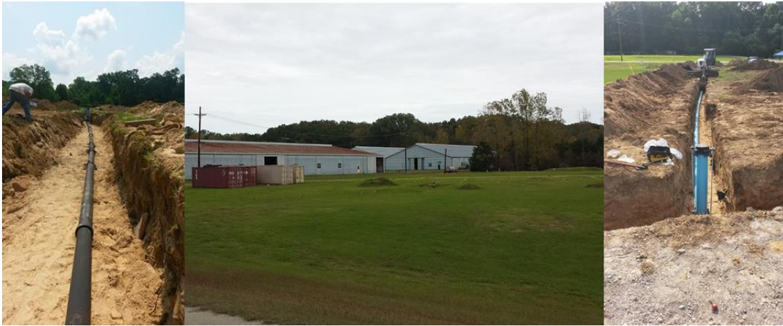
Figure 4-4. Test Bed Installation and Configuration (From left: DI pipe, aboveground view, and PVC pipe)
