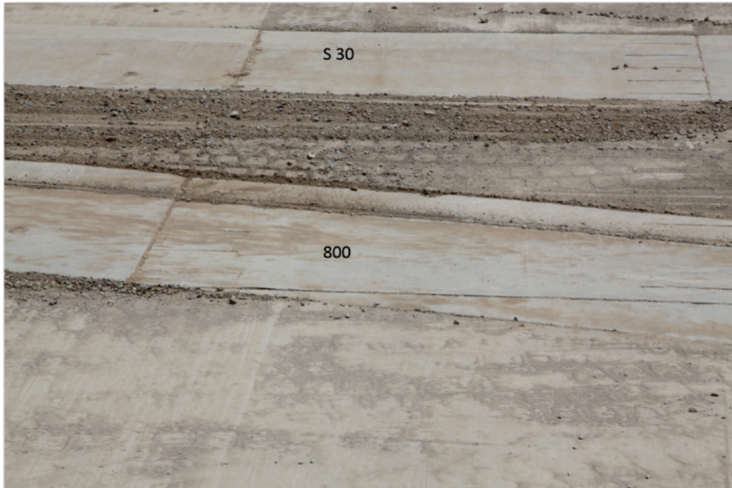
Figure 28. Tennant vacuum and brush activated in gravel.
