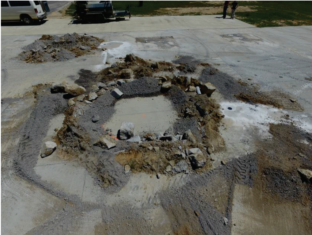
Figure 12. Mock debris crater used in equipment evaluations.
