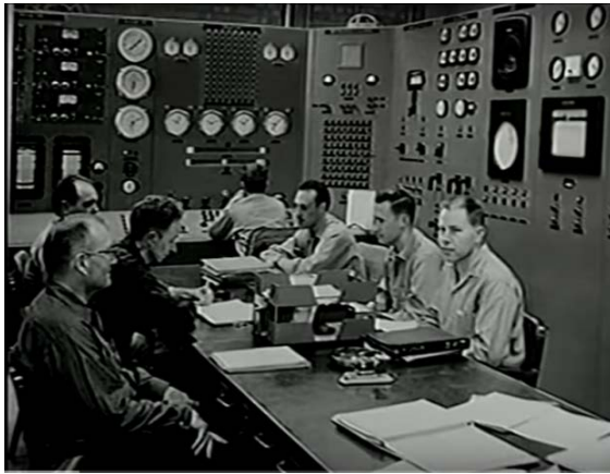
Control Room, Idaho National Laboratory 189
