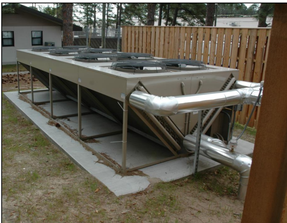
Figure 1.8. 96-ton dry fluid cooler installed at Building 584.
