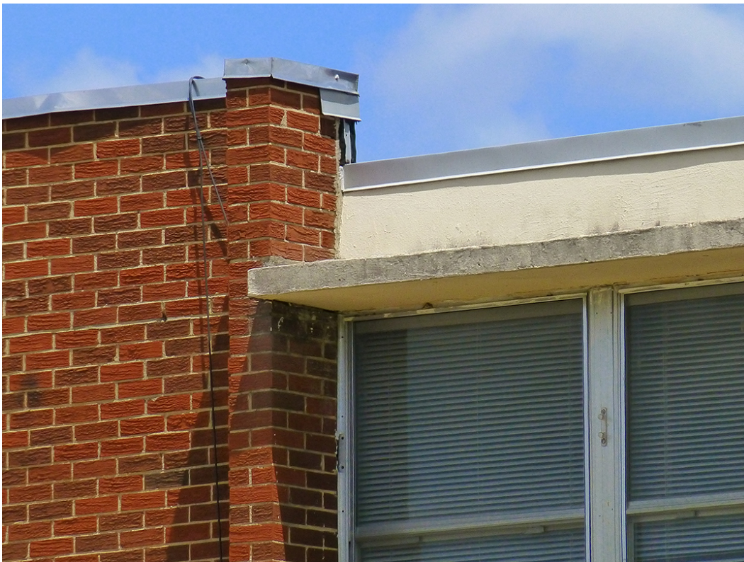
Figure 47. Detail of the concrete canopy above one of the third-floor windows on Building 33800 at Fort Gordon, GA (ERDC-CERL, 2016).
