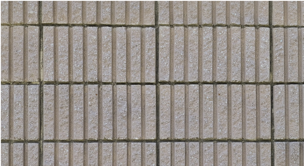
Figure 23. Detail of the split-rib concrete block on the side of Building 28414 at Fort Gordon, GA (ERDC-CERL, 2015).
