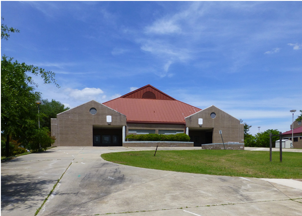
Photo 3. South side of 24414 at Fort Gordon, GA, showing large entrance plaza, clipped gable in the center, a cross gable over each entrance, precast-concrete columns, and glass-block window (ERDC-CERL, 2015).
