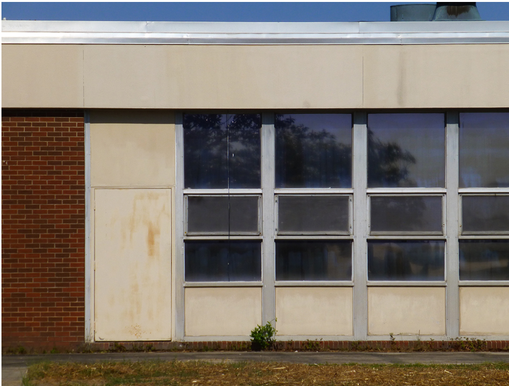
Figure 57. Looking at the original bright-aluminum window system on the east side of the old mess hall of Building 33800 at Fort Gordon, GA [the door on the left is not original] (ERDC-CERL, 2015).
