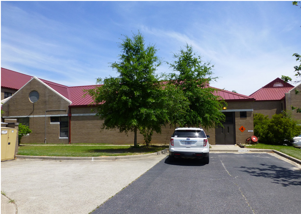
Photo 3. West side of 24411 at Fort Gordon, GA, showing cross gable on left and clipped gable on right (ERDC-CERL, 2015).
