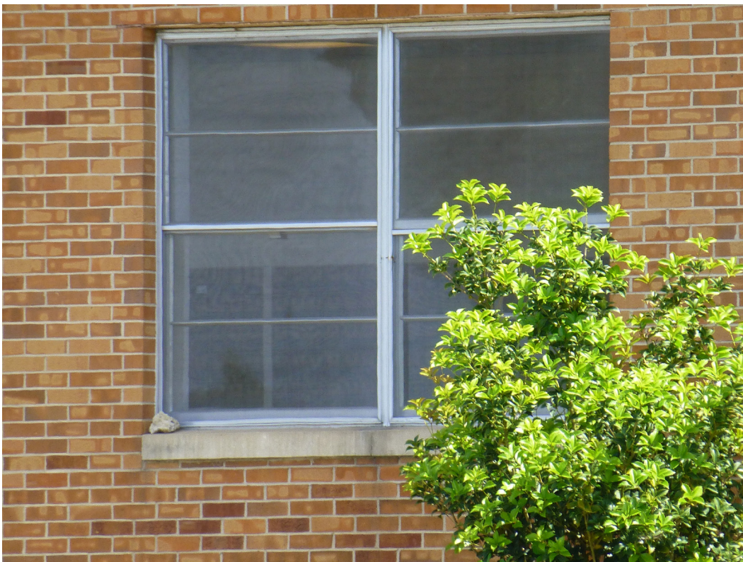
Figure 100. Detail of a paired two-over-two window on the northwest side of Building 36302 at Fort Gordon, GA (ERDC-CERL, 2015).
