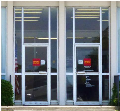
Bright-aluminum and plate-glass door frames.
