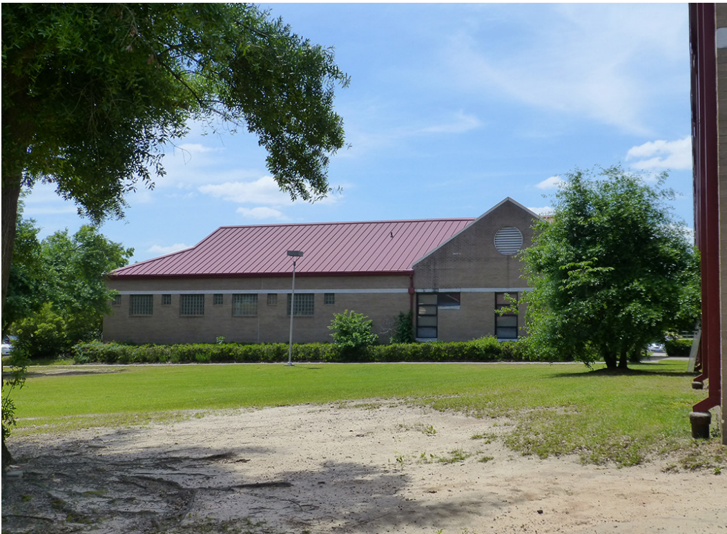
Photo 6. West side of 24411 at Fort Gordon, GA, showing clipped gable on left, cross gable on right, glass block windows, and precast-concrete belt course (ERDC-CERL, 2015).
