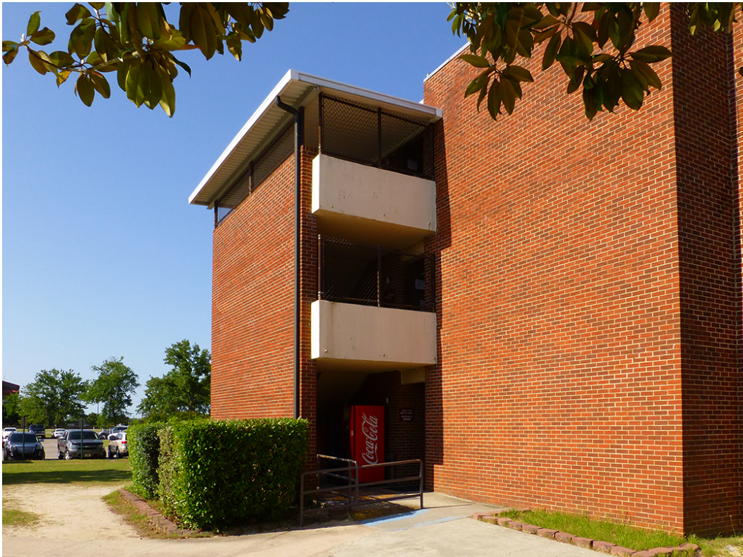
Figure 61. Detail of the external stair tower on the east side of Building 33800 at Fort Gordon, GA, showing the non-original roof and chain link (ERDC-CERL, 2015).
