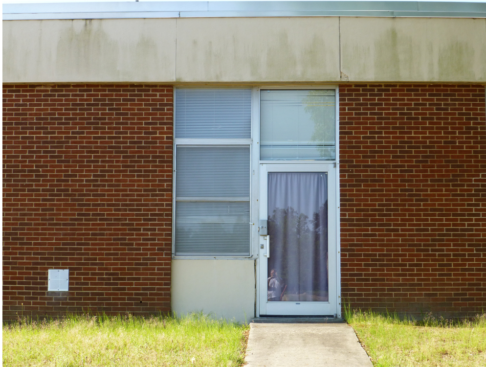
Figure 54. Original bright-aluminum plate-glass door on the north side of Building 33800 at Fort Gordon, GA (ERDC-CERL, 2015).
