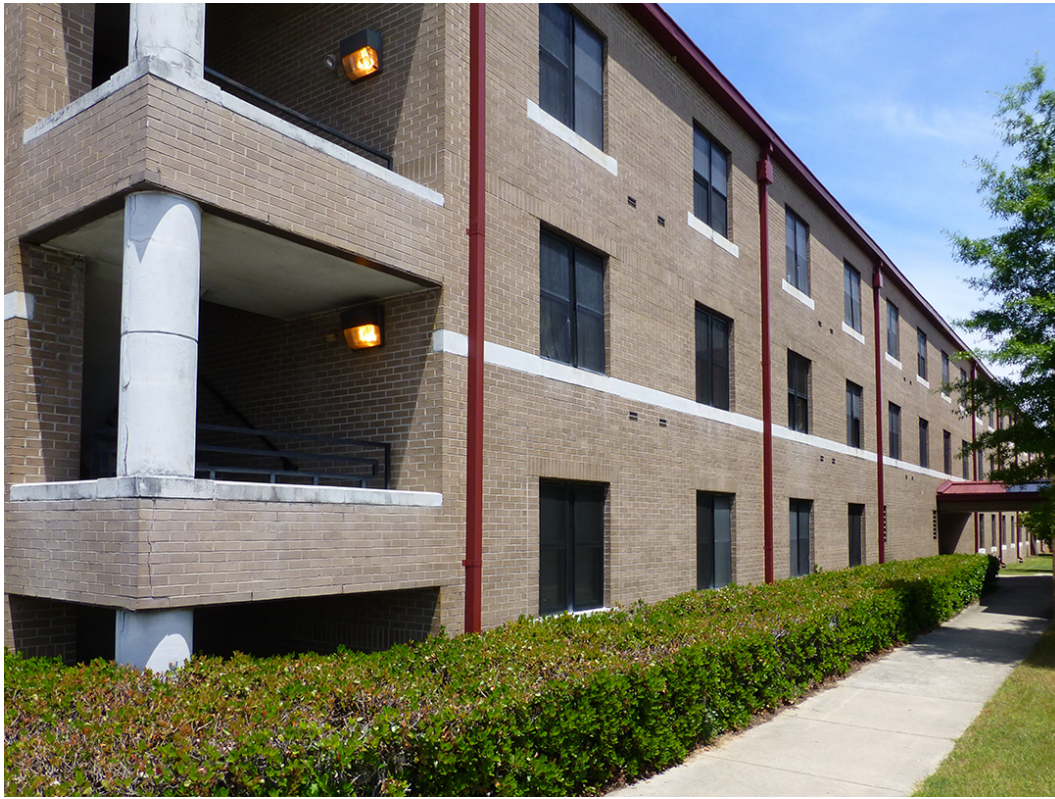
Photo 5. South side of Building 24413 at Fort Gordon, GA, showing open stair landings, precast-concrete columns, precast-concrete belt course, precast-concrete windowsills, and square window openings (ERDC-CERL, 2015).
