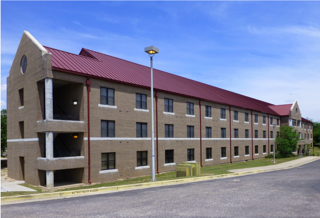
Photo 9. Southwest oblique of Building 24405 at Fort Gordon, GA, showing gable end with open stair landings, precast-concrete columns, and precast-concrete belt course (ERDC-CERL, 2015).
