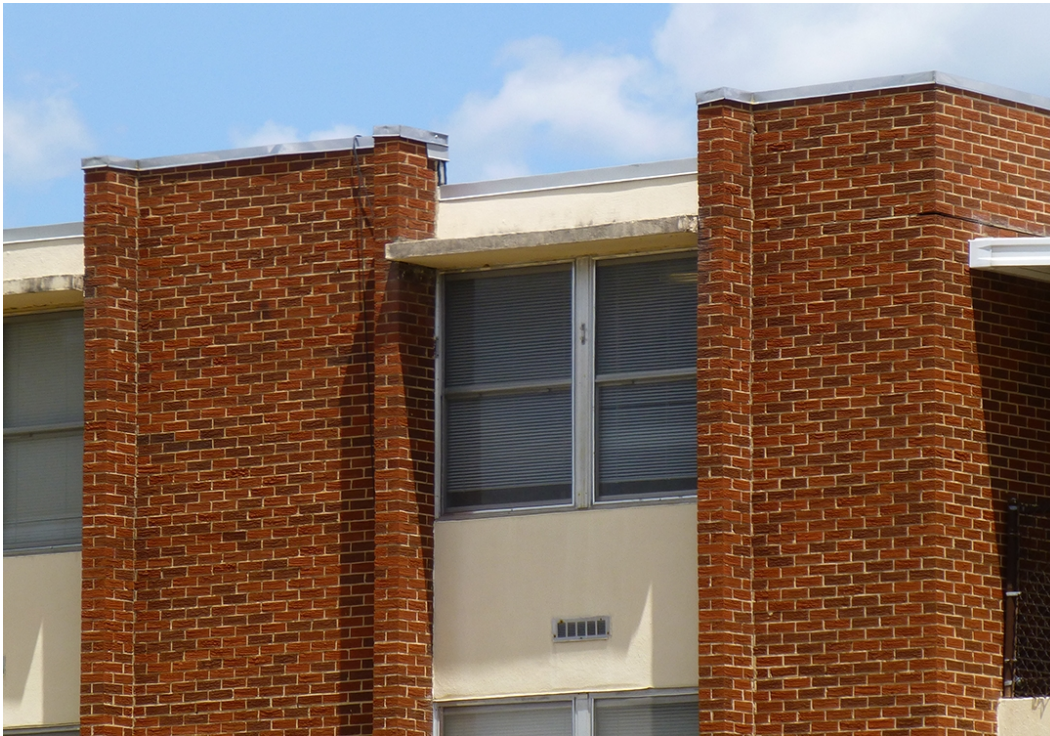
Figure 46. Detail of the bright-aluminum windows, stucco spandrels, and red brick detailing of Building 33800 at Fort Gordon, GA (ERDC-CERL, 2016).
