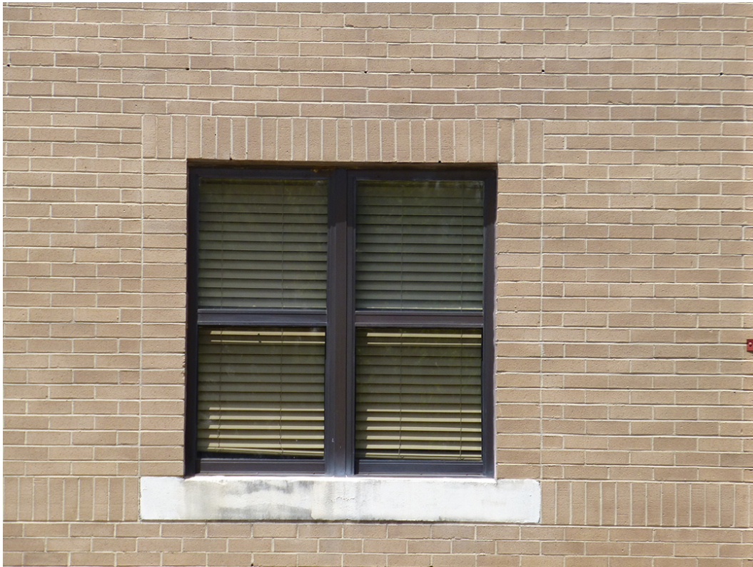
Photo 15. Detail of double window and precast-concrete windowsill on southside of Building 24401 at Fort Gordon, GA (ERDC-CERL, 2015).
