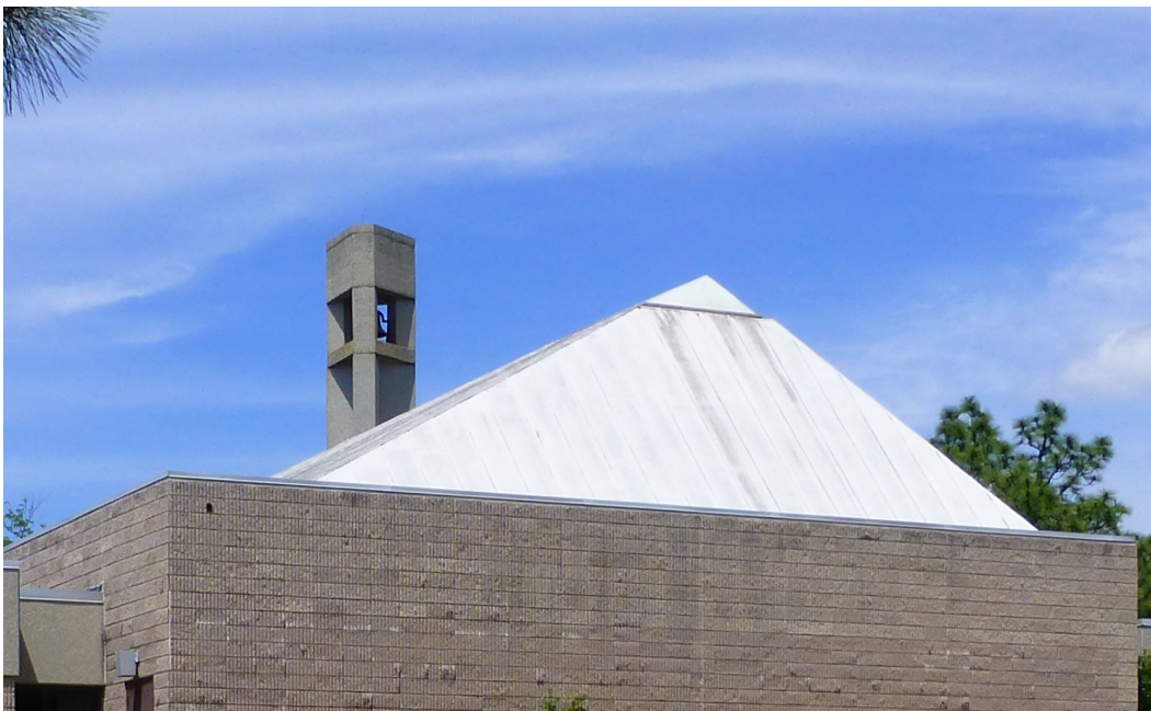
Figure 24. Terne metal-clad pyramidal roof with skylight cap on Building 28414 at Fort Gordon, GA (ERDC-CERL, 2015).
