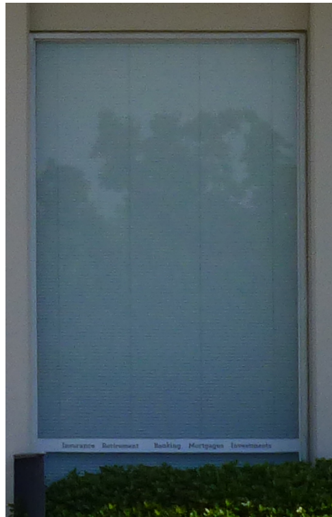
Bright-aluminum and plate-glass window frames.
