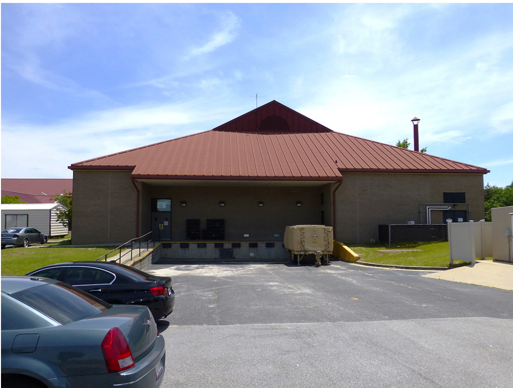
Photo 6. North side of Building 24414 at Fort Gordon, GA, showing clipped gable and loading dock (ERDC-CERL, 2015).
