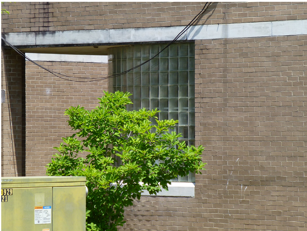
Photo 4. Northwest corner of 24411 at Fort Gordon, GA, showing curved glass block window, precast-concrete windowsill below, and precast-concrete belt course above (ERDC-CERL, 2015).
