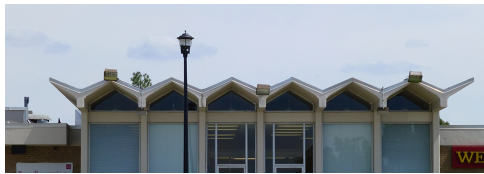
Pre-cast concrete folded-plate roof.
