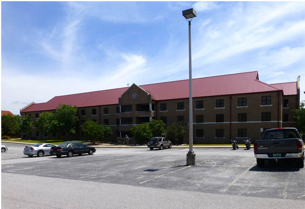
Photo 3. North side of Building 24413 at Fort Gordon, GA, showing the clipped gables, the cross gable, square window openings, precast-concrete belt course, and precast-concrete windowsills (ERDC-CERL, 2015).
