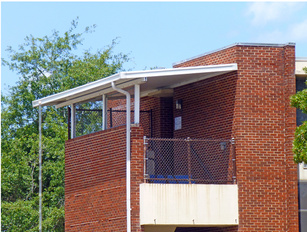
Figure 58. Detail of the external stair tower on the south side of Building 33800 at Fort Gordon, GA, showing the non-original roof and chain link (ERDC-CERL, 2016).
