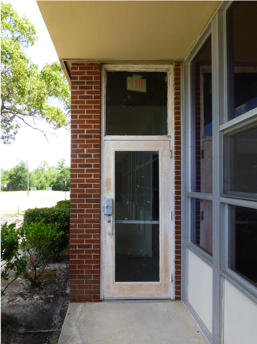
Figure 50. Original bright-aluminium plate-glass door that leads into the former mess hall on the west side (front) of Building 33800 at Fort Gordon, GA (ERDC-CERL, 2016).
