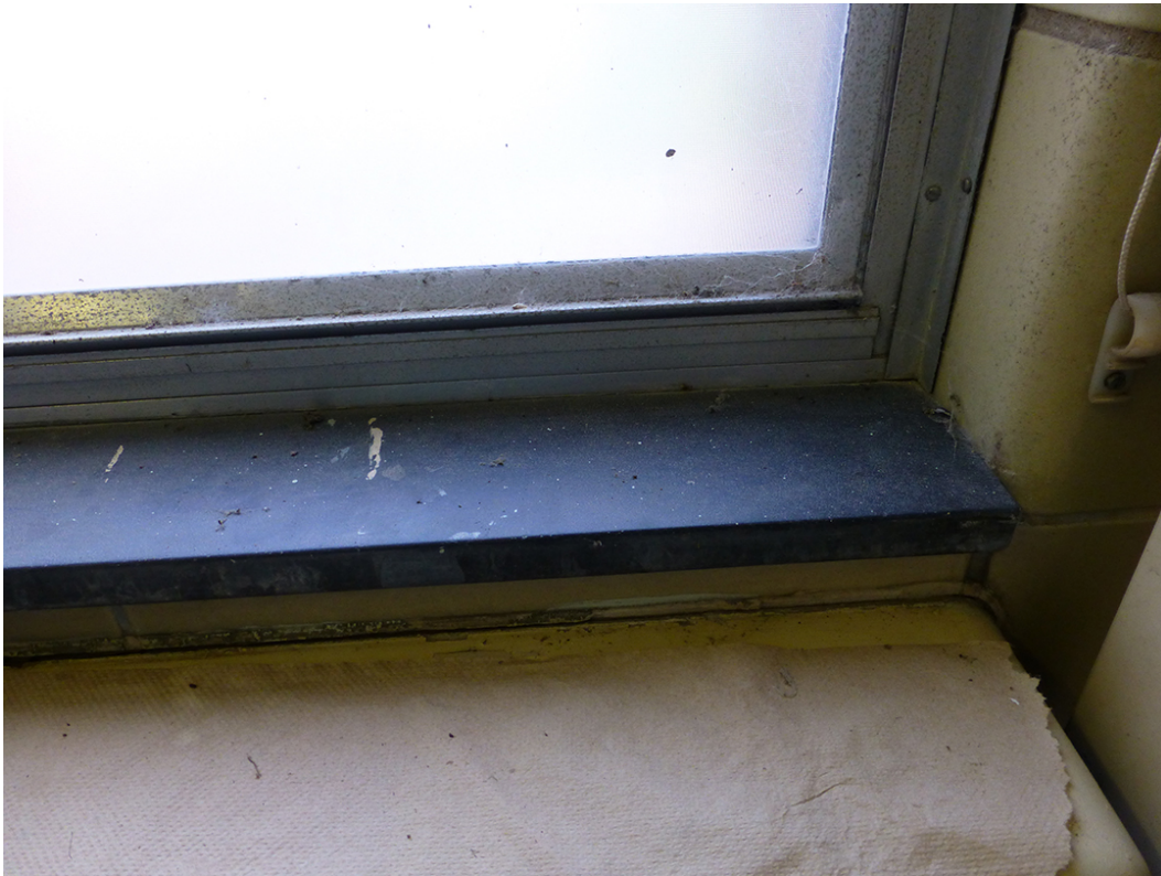
Figure 75. Detail of one of the original soapstone windowsills in the women's latrine on the first floor of Building 33800 at Fort Gordon, GA (ERDC-CERL, 2016).
