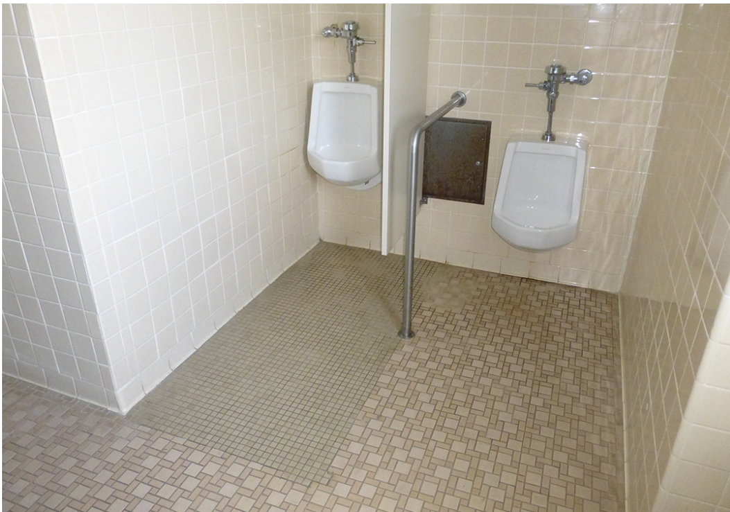
Figure 74. View of how the second tub area has been transformed with the removal of the tub and the addition of urinals in the men's latrine on the first floor of Building 33800 at Fort Gordon, GA (ERDC-CERL, 2016).
