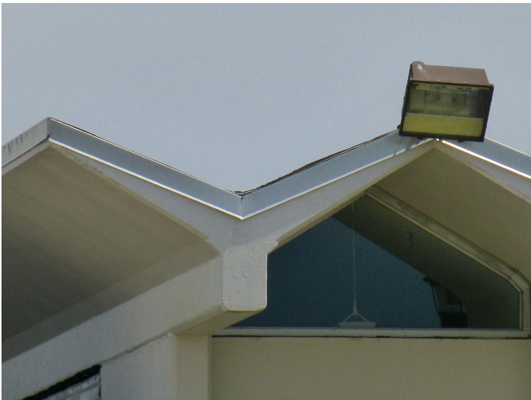
Figure 94. Detail of the pre-cast concrete folded-plate roof on Building 36300 at Fort Gordon, GA (ERDC-CERL, 2015).
