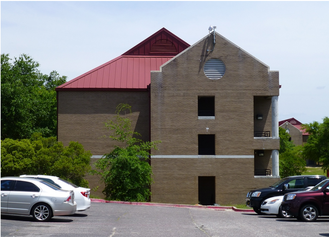
Photo 7. West side of Building 24407 at Fort Gordon, GA, showing gable end with open stair landings, precast-concrete columns, and precast-concrete belt course (ERDC-CERL, 2015).
