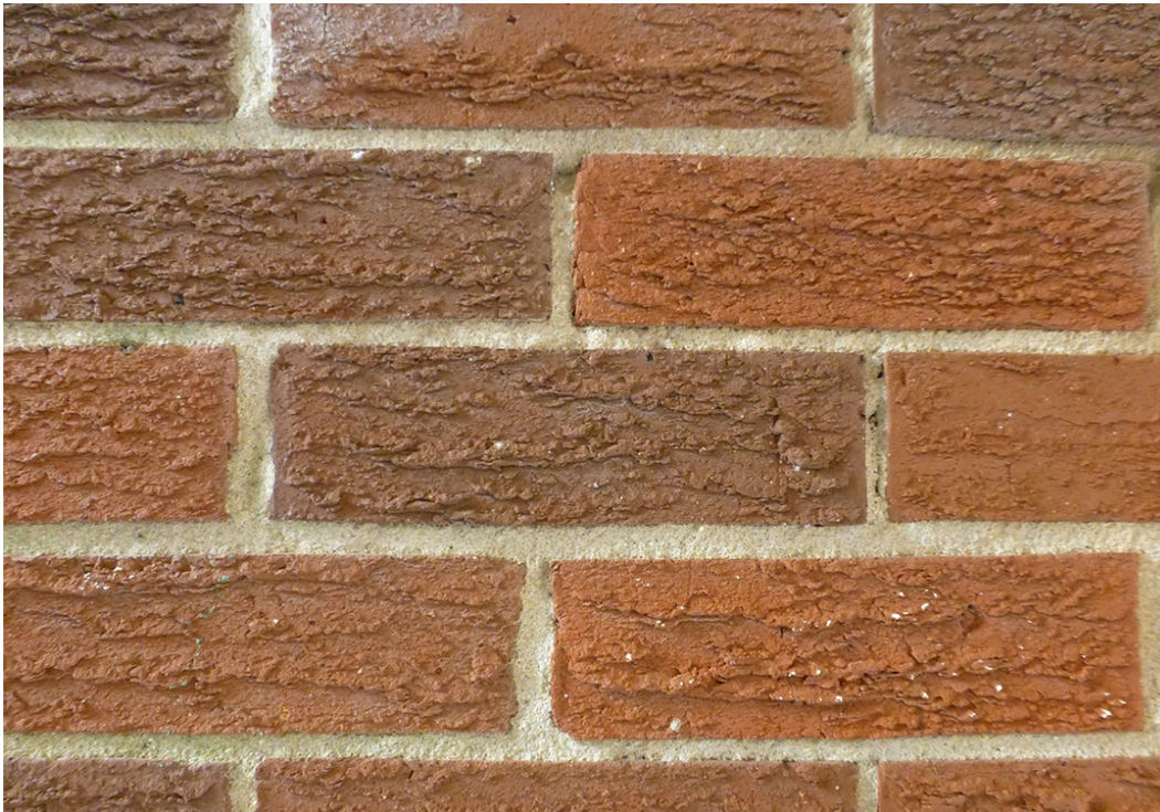
Figure 45. Detail of the textured red brick utilized on the exterior of Building 33800 at Fort Gordon, GA (ERDC-CERL, 2016).
