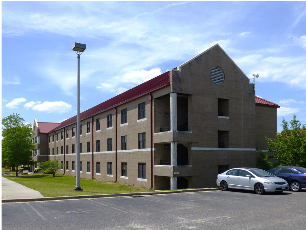
Photo 18. East side of Building 24404 at Fort Gordon, GA, with open stair landings and precast-concrete columns at the corner (ERDC-CERL, 2015).
