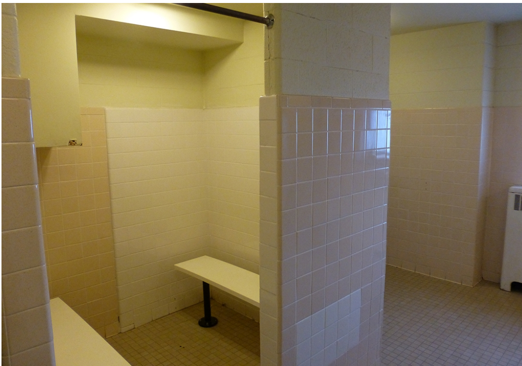
Figure 86. This tub has been removed and replaced with benches in the latrine on the second floor of Building 33800 at Fort Gordon, GA (ERDC-CERL, 2016).
