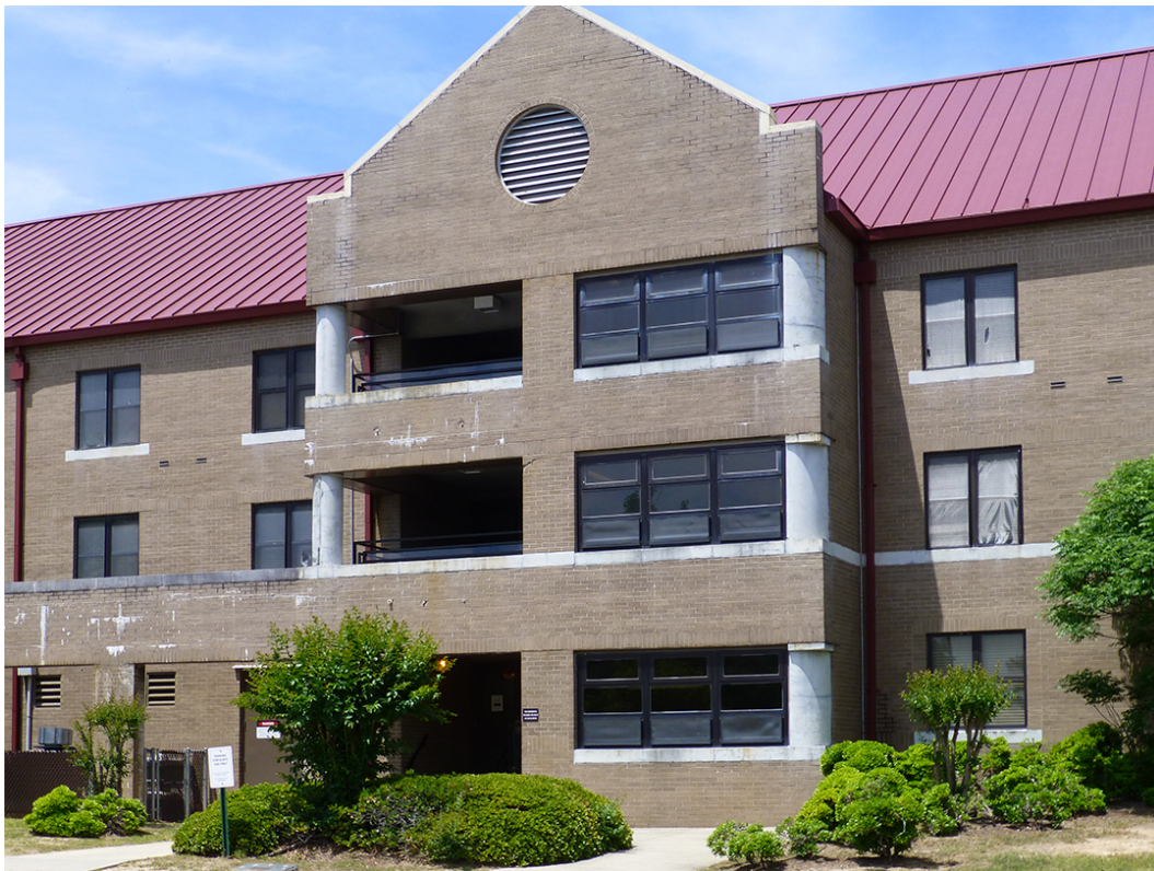
Photo 13. Detail of projecting entrance bay on southside of Building 24401 at Fort Gordon, GA, showing cross gable with balconies , precast-concrete columns, and precast-concrete belt course (ERDC-CERL, 2015).
