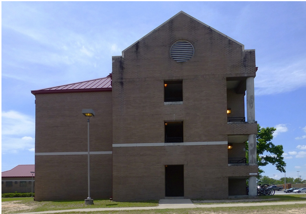
Photo 6. East side of Building 24413 at Fort Gordon, GA, showing gable end with open stair landings, precast-concrete columns, and precast-concrete belt course (ERDC-CERL, 2015).
