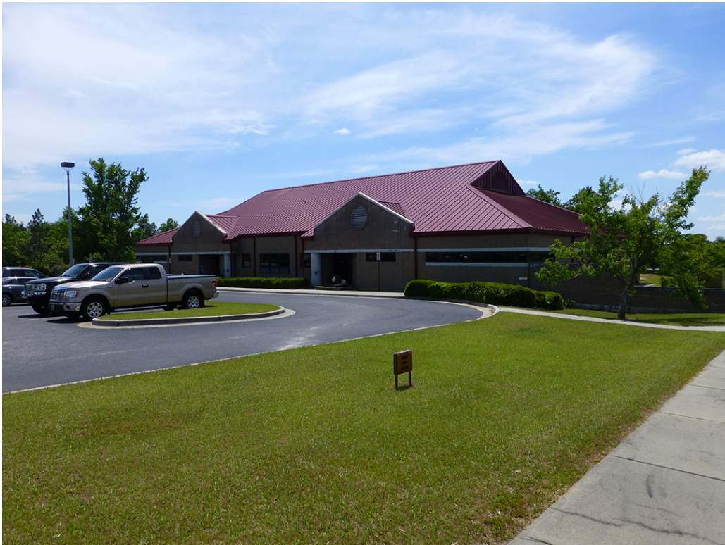
Photo 3. Northeast oblique of Building 24402 showing clipped gable, cross gables at entrances, precast-concrete columns, precast-concrete belt course, and precast-concrete windowsills (ERDC-CERL, 2015).
