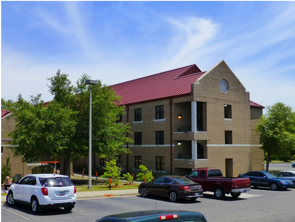
Photo 11. Northwest oblique of Building 24401 at Fort Gordon, GA, showing precast-concrete columns and open stair landings (ERDC-CERL, 2015).
