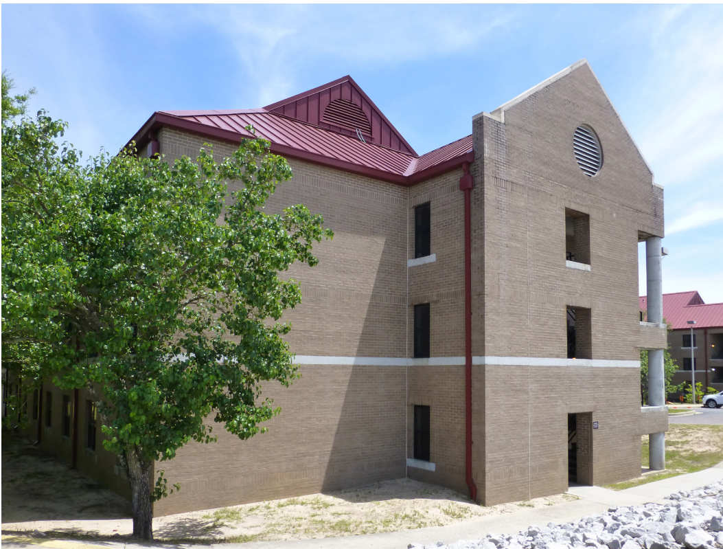
Photo 8. West side of Building 24405 at Fort Gordon, GA, showing gable end with open stair landings, precast-concrete columns, and precast-concrete belt course (ERDC-CERL, 2015).
