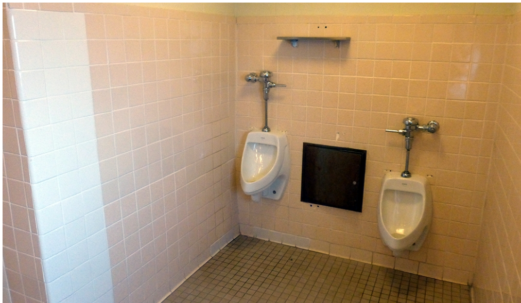
Figure 87. This tub has been removed and replaced with urinals in the latrine on the second floor of Building 33800 at Fort Gordon, GA (ERDC-CERL, 2016).
