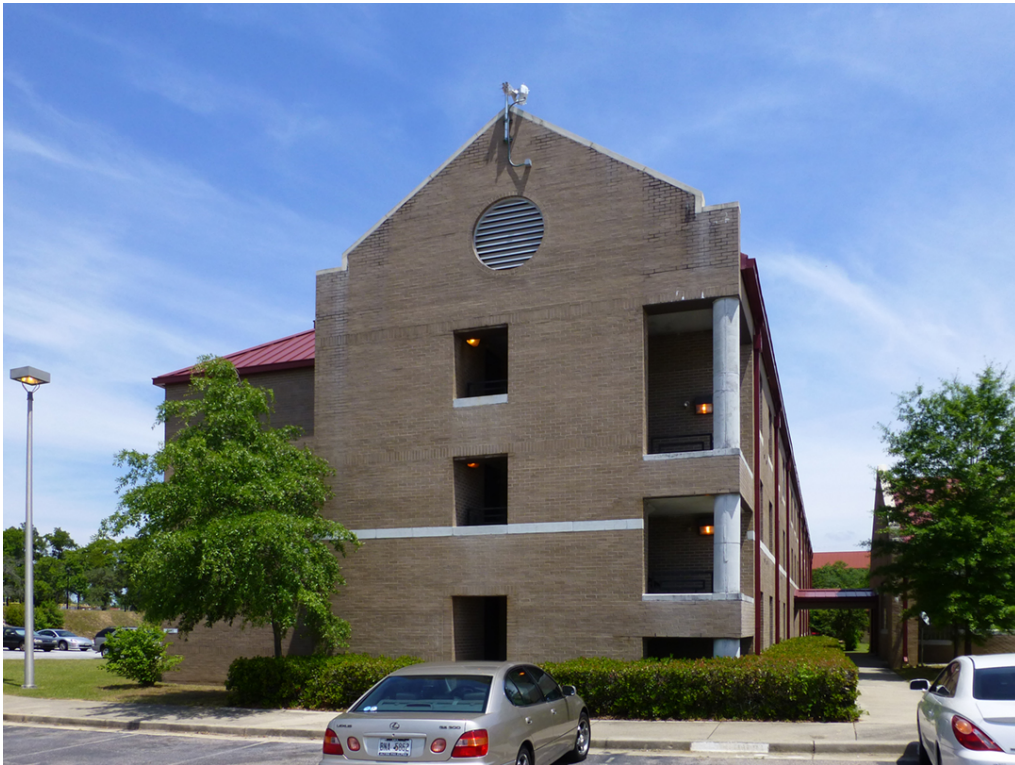
Photo 4. West side of Building 24413 at Fort Gordon, GA, showing gable end with open stair landings, precast-concrete columns, and precast-concrete belt course (ERDC-CERL, 2015).
