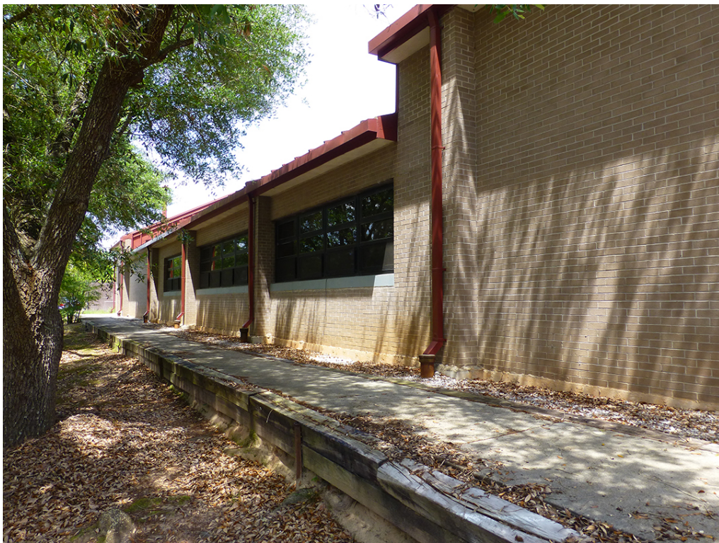
Photo 4. West side of Building 24414 at Fort Gordon, GA, showing tan brick, brick buttresses, and window openings (ERDC-CERL, 2015).
