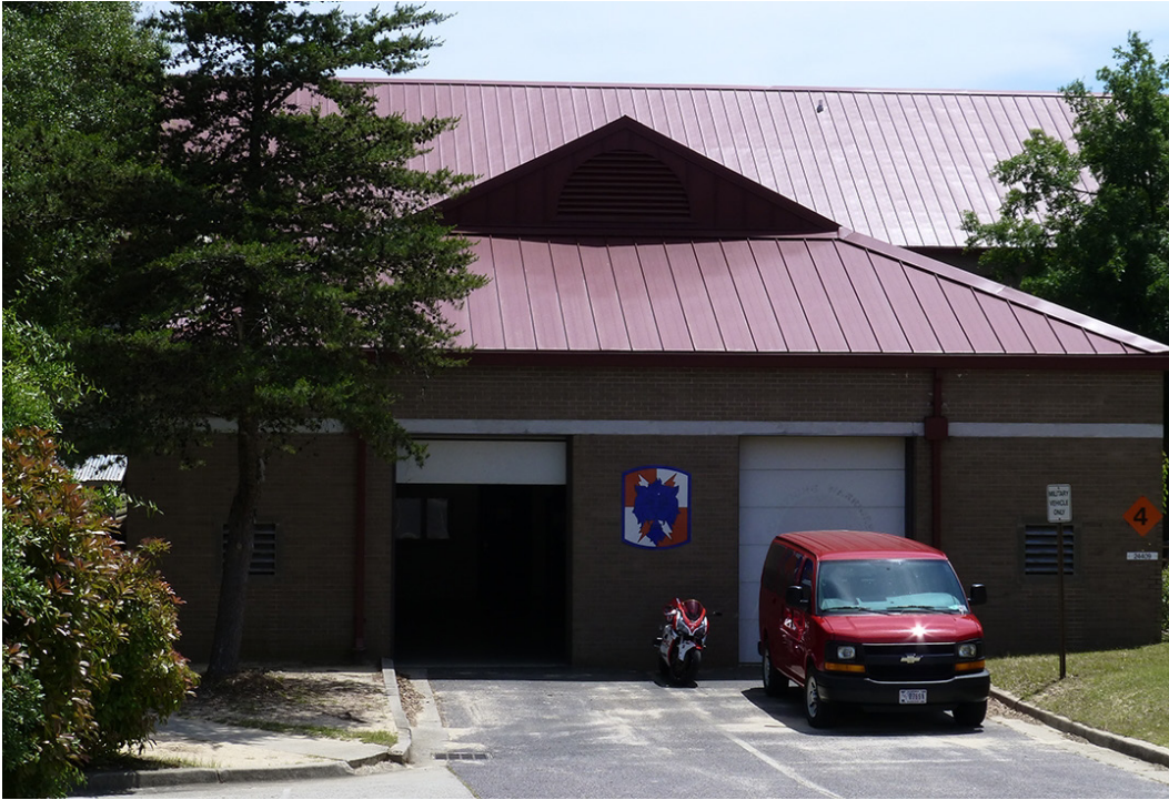
Photo 5. North side of 24409 at Fort Gordon, GA, showing clipped gable and two large openings with panel lift doors (ERDC-CERL, 2015).
