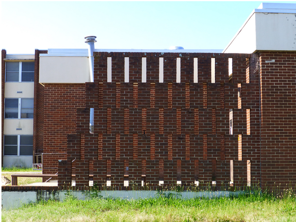
Figure 53. Close-up of original perforated block wall on the north side of Building 33800 at Fort Gordon, GA (ERDC-CERL, 2015).
