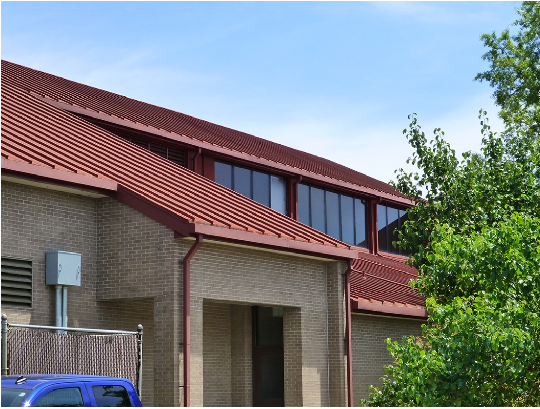
Photo 7. Detail of west side of Building 24414 at Fort Gordon, GA, showing west entrance, red metal roof, and clerestory windows (ERDC-CERL, 2015).
