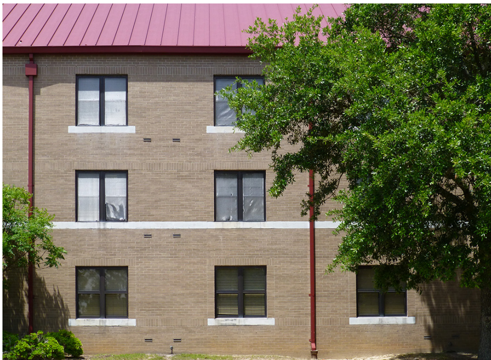
Photo 14. Detail of windows on southside of Building 24401 at Fort Gordon, GA, showing square window openings, precast-concrete belt course, and precast-concrete windowsills (ERDC-CERL, 2015).
