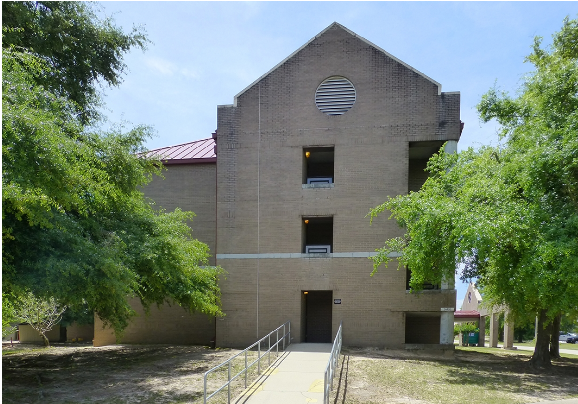
Photo 10. East side of Building 24405 at Fort Gordon, GA, showing gable end with open stair landings, precast-concrete columns, and precast-concrete belt course (ERDC-CERL, 2015).
