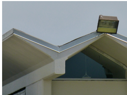
Detail of pre-cast concrete folded-plate roof.
