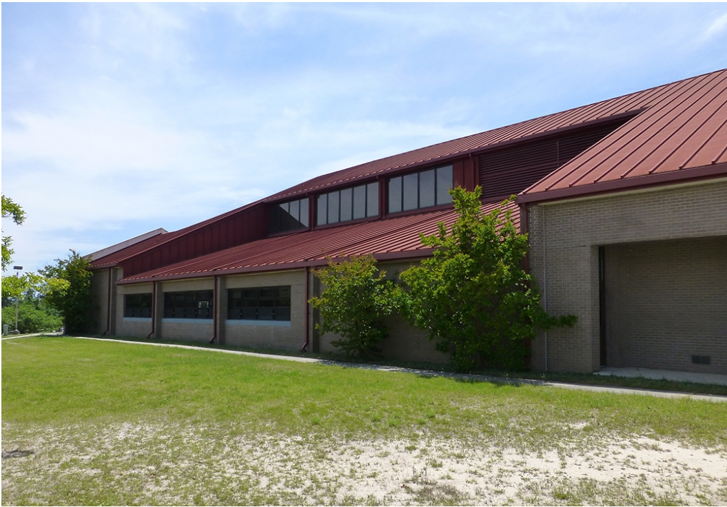
Photo 5. East side of Building 24414 at Fort Gordon, GA, showing red metal roof, high-height space, and clerestory windows (ERDC-CERL, 2015).
