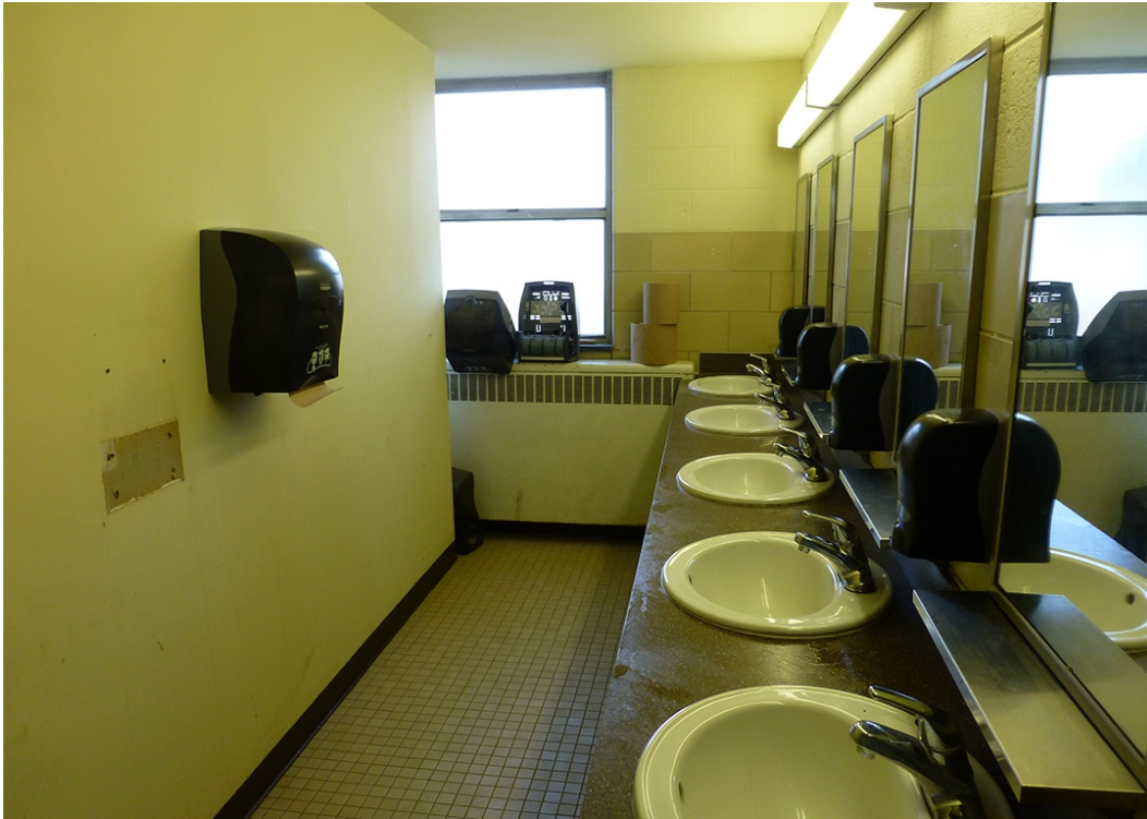
Figure 85. Sinks in the lavatory were removed and replaced, and a wall was constructed to separate the room into male and female latrines on the second floor of Building 33800 at Fort Gordon, GA (ERDC-CERL, 2016).
