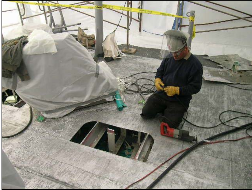
Figure 2. A Worker Prepares to Replace a Stress Corrosion Cracking Damaged Ship Section. Source: [3].
