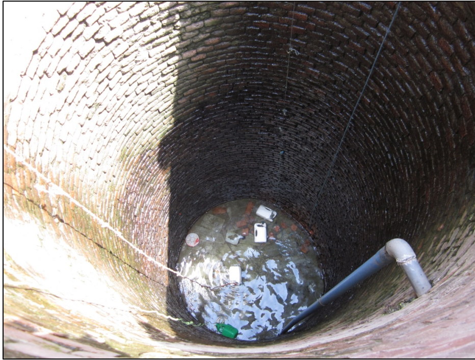
Figure C14. Nearly dry well in India (commons.wikimedia.org, 2014).
