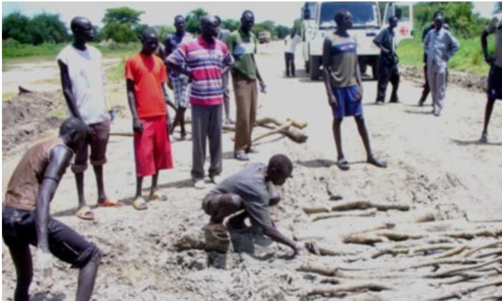
Figure C33. Locals repair potholes on Juba-Bor road, South Sudan (voanews.com, 2011).
