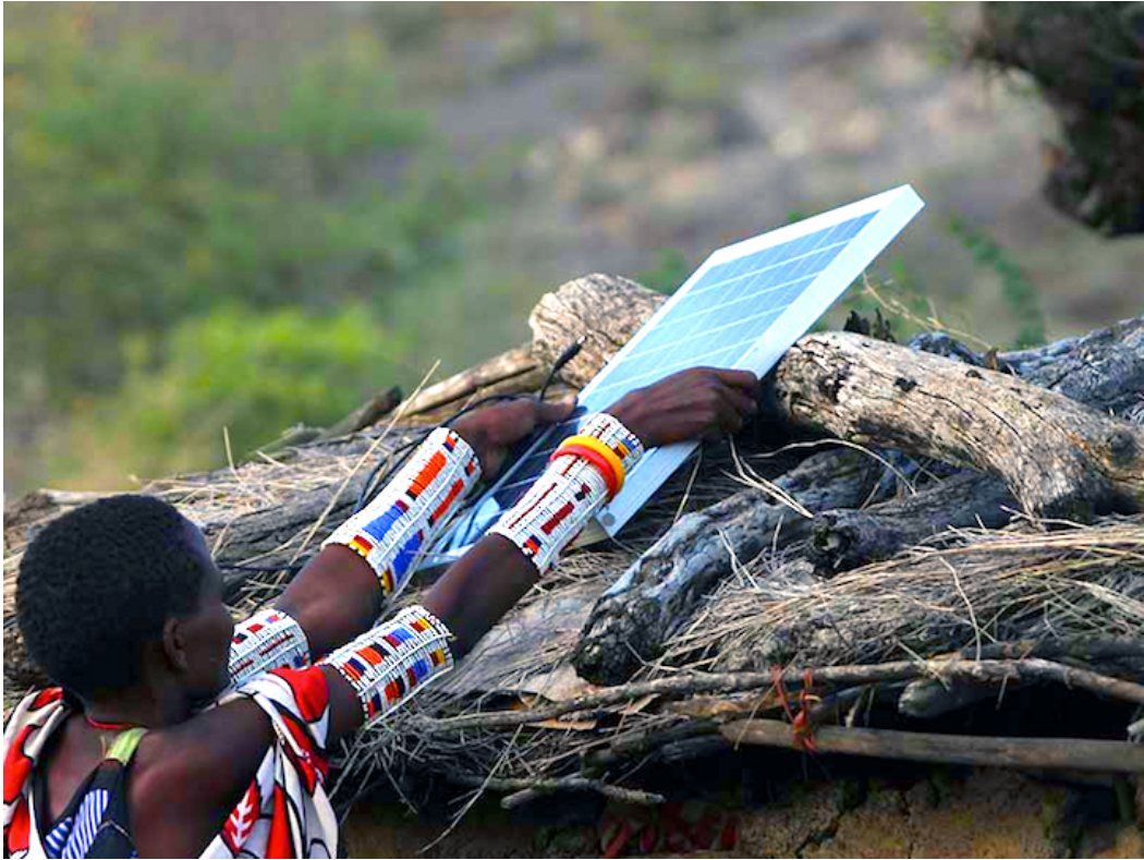
Figure C12. Installation of solar panels in Africa (inhabit.com. 2015).
