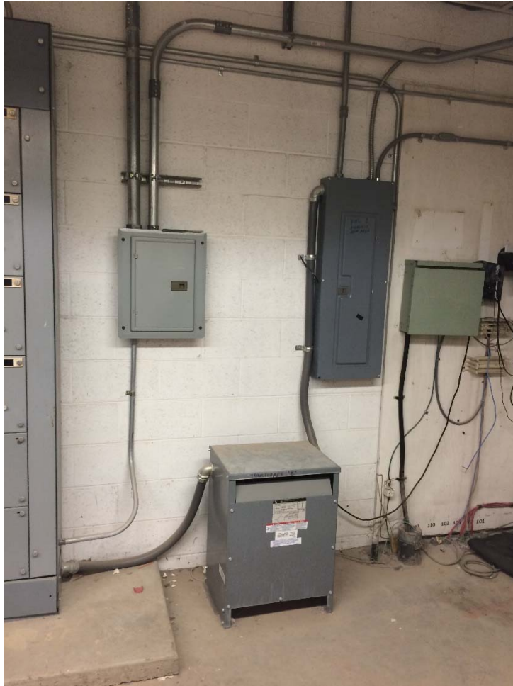
Figure 7. Photo Inside of the Electrical Room at Building B1588, Showing a 480-208V Transformer Mounted to the Floor, and Electric Load Panels Mounted to the Wall.
