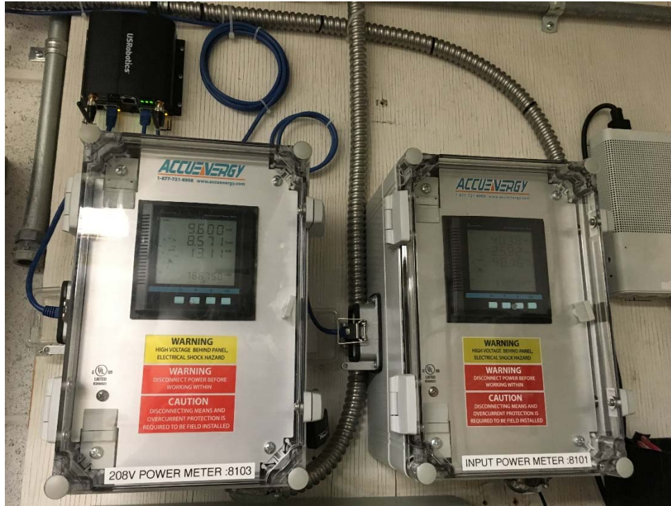
Figure 12. Installed Meters and Cellular Router for Data Retrieval.
