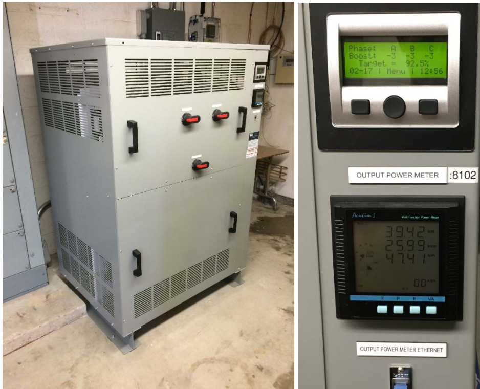
Figure 11. The EVR device installed in the building, and the meter panel display.
