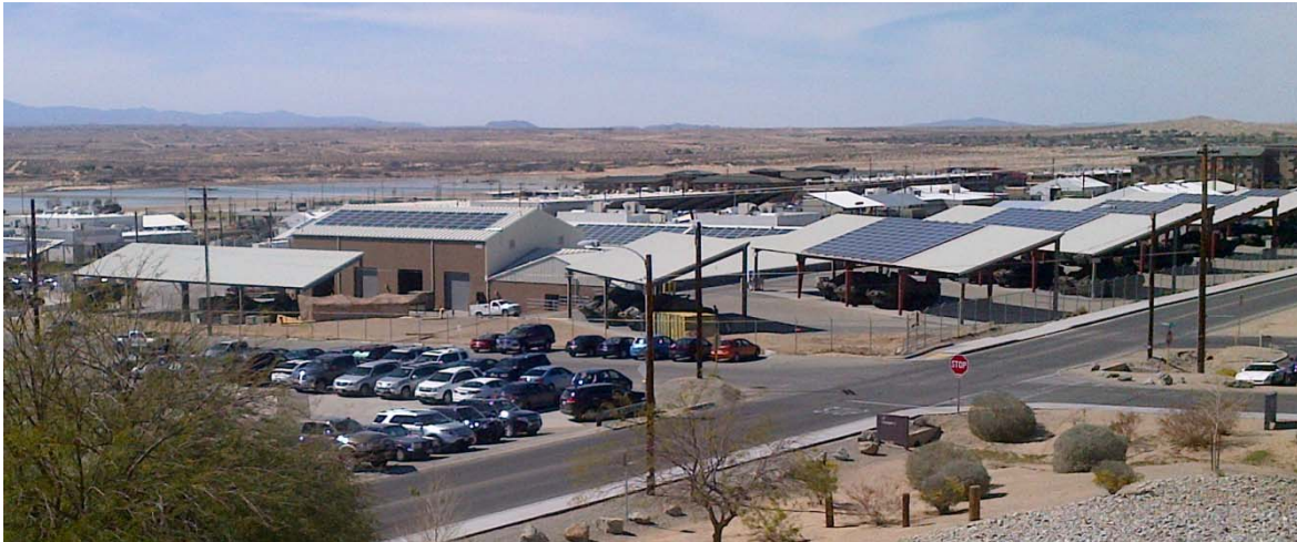
Figure 5. Photo of Equipment Garages with Rooftop Solar Installations at MCAGCC in Twenty-nine Palms, CA Showing Pole Mounted 12.5kV AC Distribution Network.
