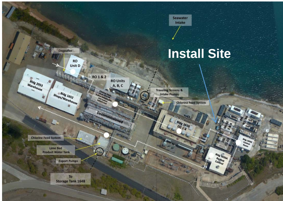
Figure 2. GTMO Installation Site
