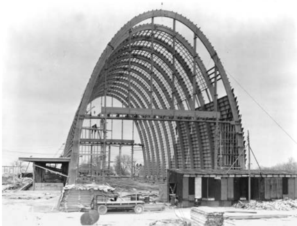
When completed, the all-wooden Radar Test Facility (Building 821) supported pioneering stealth technology research
