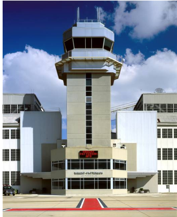
Wright-Patterson's new control tower, 2003
