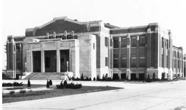
Building 12, Technical Data Library and Museum
