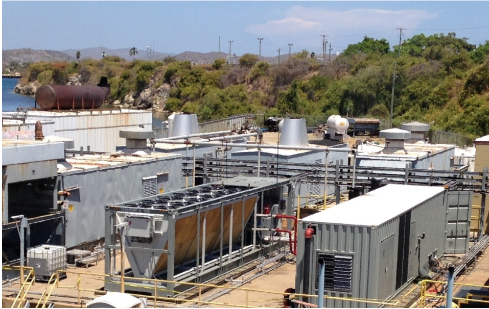
Figure 5. ORC and Genset Installation at GTMO
