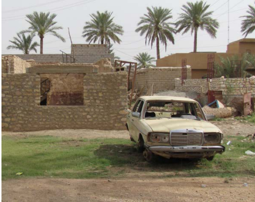
Figure B-3. Remnants of Jassim's house
