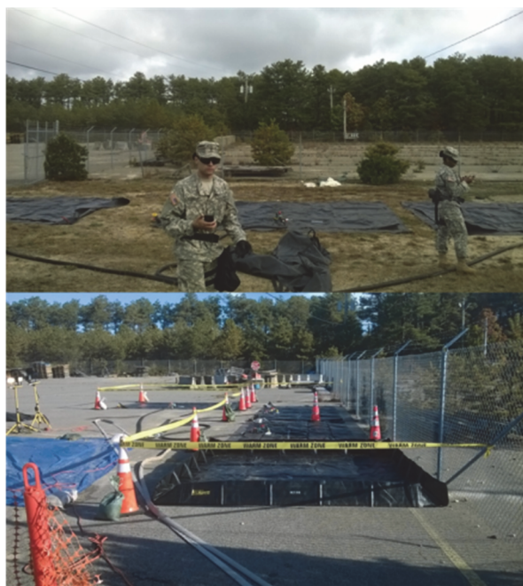
Figure 4. Massachusetts National Guard 272 nd Chemical Company CBRN Response Team's effluent collection blivets. Each of the three active blivets holds up to 1500 gallons of effluent waste, with one reserve blivet on hand to extend capacity.
