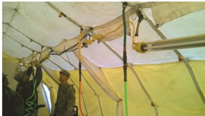
Figure 1. Soldiers setting up water and power lines in the Interior of a personnel decontamination tent. Figure courtesy of Massachusetts National Guard.
