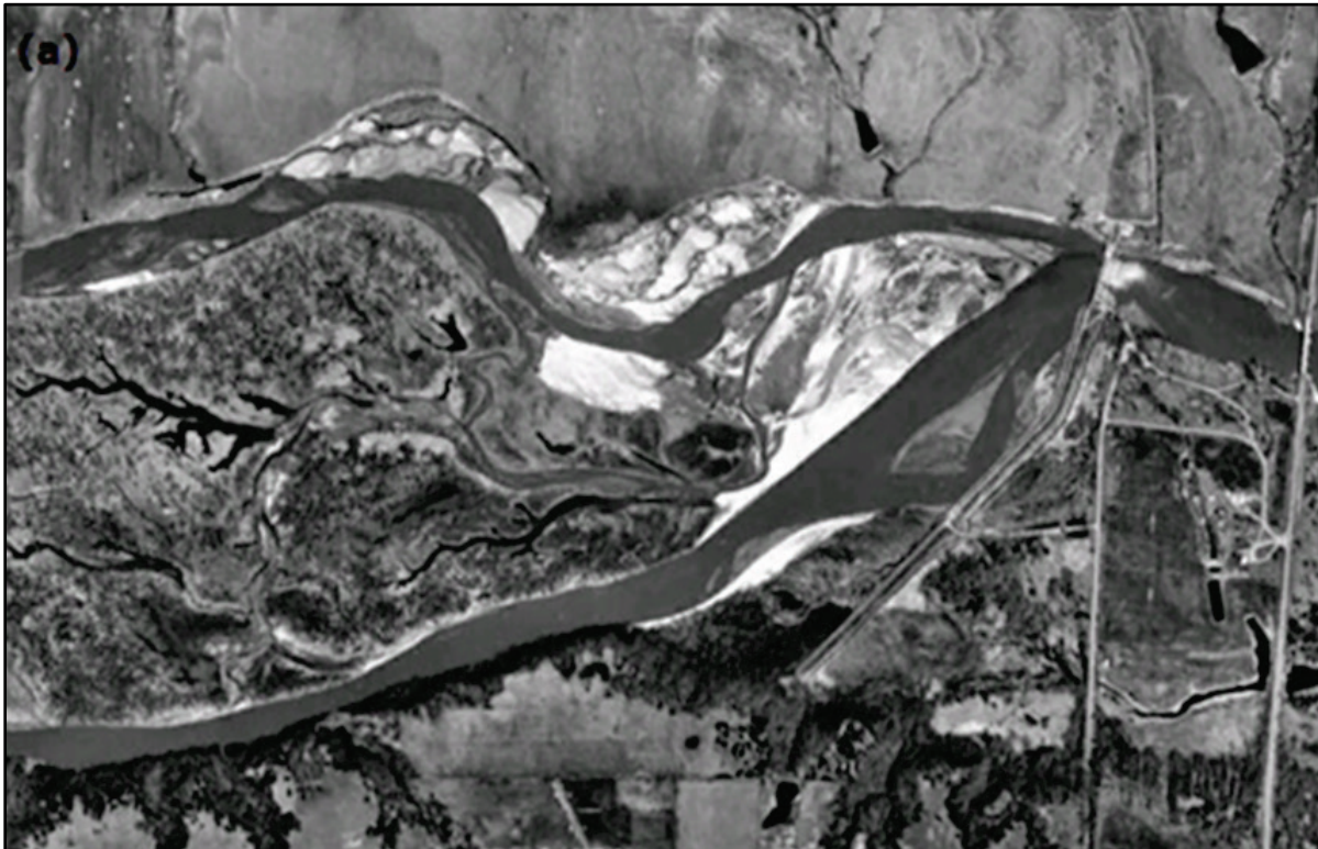
Figure 2. Spencer Dam during flush.
