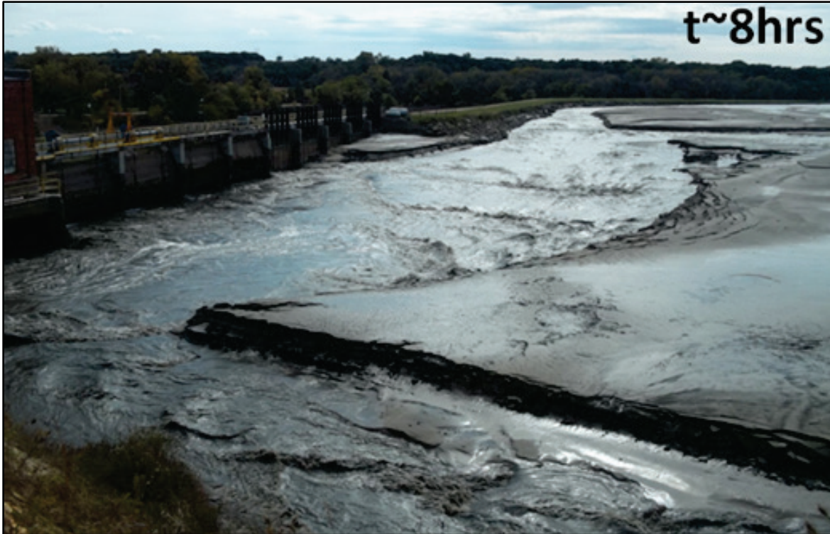
Figure 5. Multiple channels eroded throughout 6 October 2014. Time approximately 8 hours (hr) after opening main gates.
