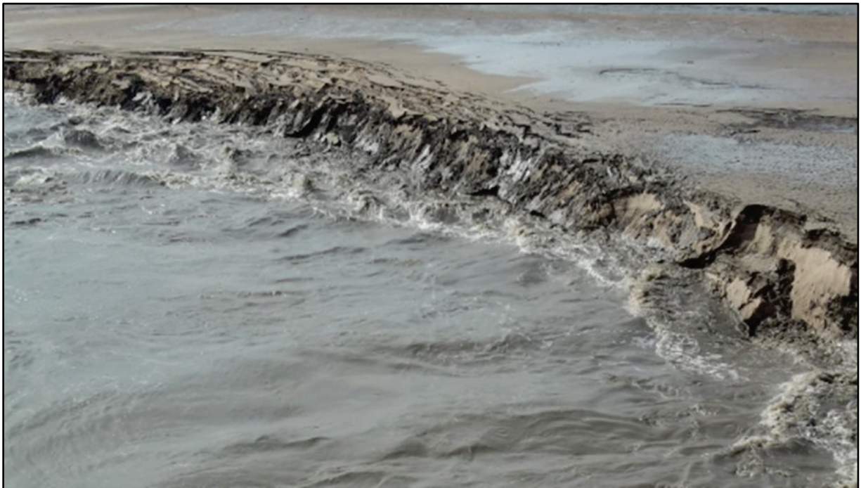
Figure 12. Lateral erosion processes (undercutting and slumping) observed during the flush in the vicinity of the cross section shown in Figure 10.
