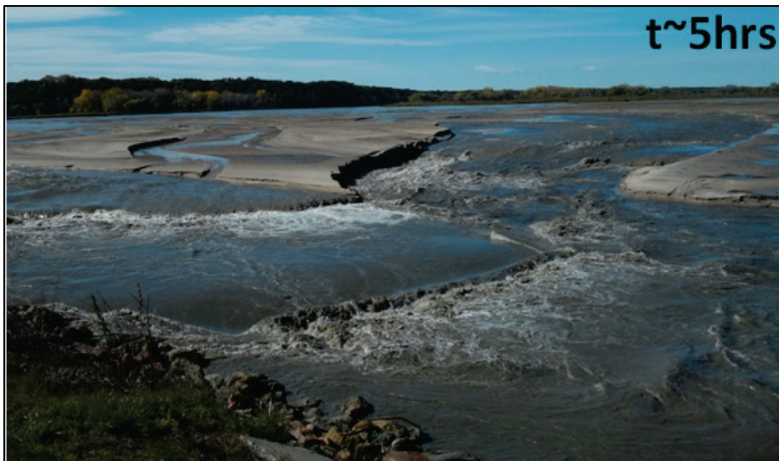
Figure 4. Opening sluice gate that was 4 ft lower than main gates pushed a head cut rapidly upstream through reservoir sediment. Time approximately 5 hours (hr) after opening main gates.
