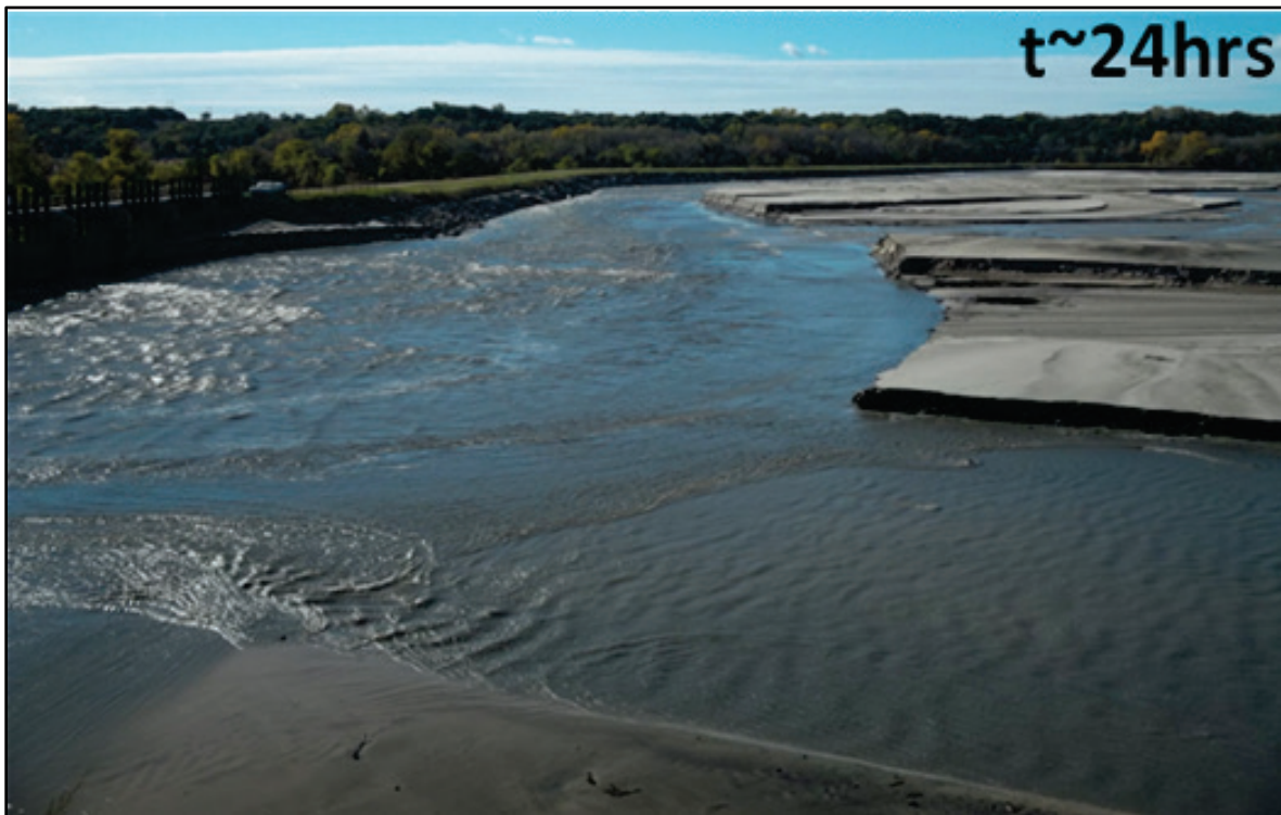
Figure 6. Historic channel incised enough to capture most of the flow, stranding the rest of the reservoir sediment in terraces. Time approximately 24 hr after opening main gates.
